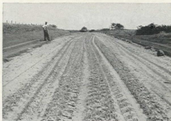
The sandy type soil in place ready for processing by the P&H Soil Stabilizer.
