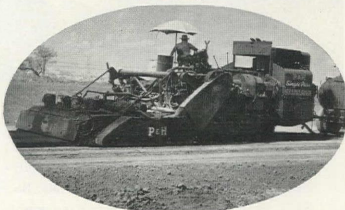
The P&H Soil Stabilizer processing at a rate of 500 lineal feet, 24-foot highway per hour.
