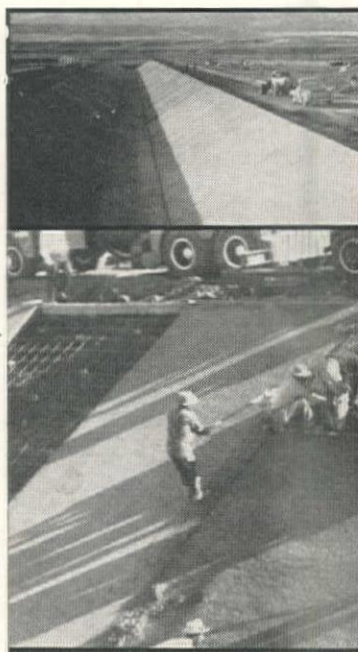
Templeton Gap Spillway, Colorado Springs, Colo. Angle 45°, Concrete slump ¾". Extra men on screed for weight only.
