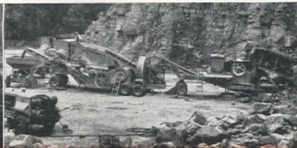
4 TwinDual Secondary with 546P Primary. High capacity with two portable units for quarry operation
