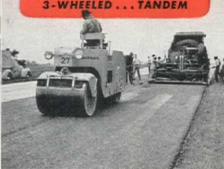
3-WHEELED ROLLERS with hydraulic scarifiers. TANDEM ROLLERS of the variable weight type. All with gas or diesel engines.
