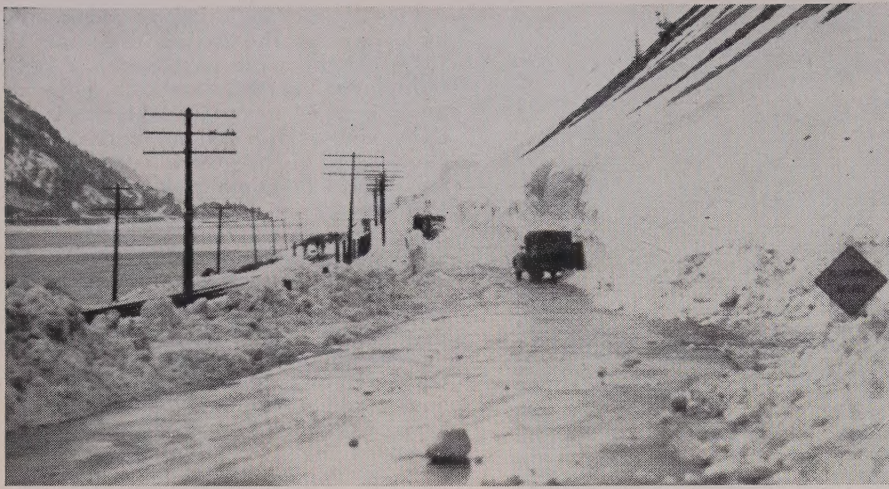
A SEVERE WINTER , coupled with a continuing increase in heavy truck traffic, caused excessive damage to Oregon highways. At left, a sleet slide last January cut off travel entirely on the Columbia River Highway 8 mi. east of Cascade Locks.
