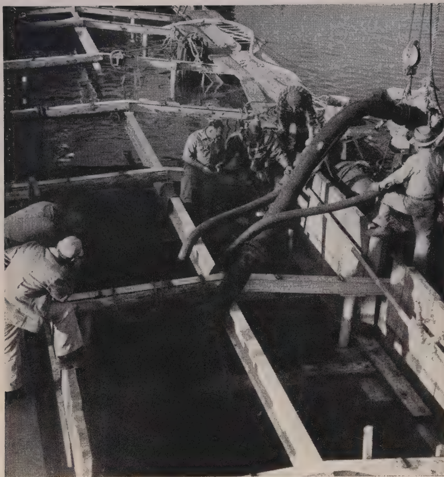
AFT END of the dredge during raising operations, with timber cofferdam around 300-kw. generator pit. Bulkheads around the two engine rooms were placed 1 ft. above water.
