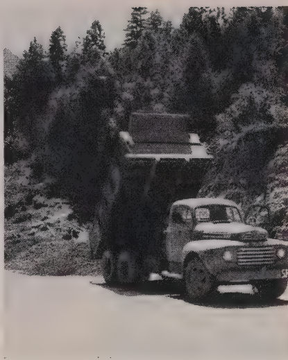
SURFACING consists of a 12-in. depth of river gravel, dumped and spread in the 30-ft. width of roadway.
