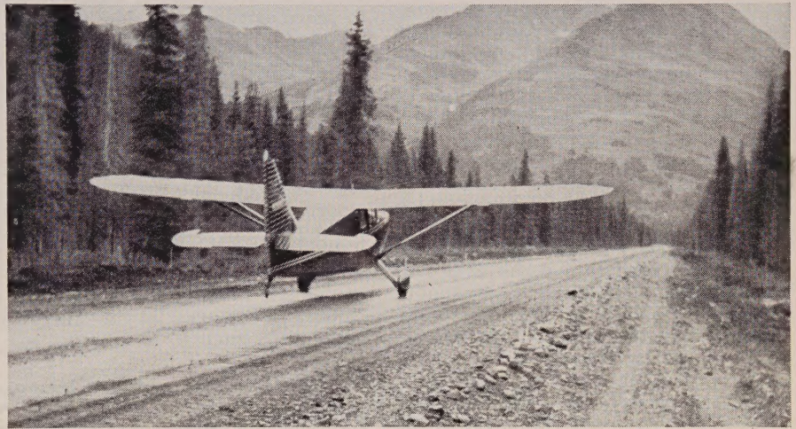
PLANE taking off from new grade on the C. F. Lytle Co. and Green Construction Co. Turnagain Arm contract section. Due to isolation of the work, airplanes were used constantly for transportation of personnel and emergency supplies, such as critical repair parts.
