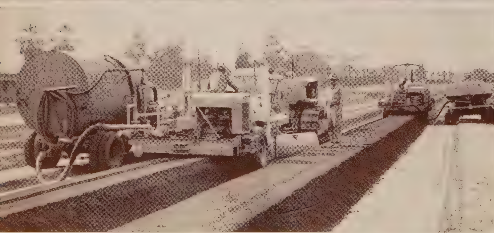
SOIL CEMENT stabilization is now extensively used in California. View is of a recent job at Riverside, with J. A. Payton as contractor. Two Wood Model 54 Roadmixers were used to prepare the roadway with a 5-in. thickness. An average of 300 tons was mixed per hour, and soil cement for 2.6 mi. of the 26-ft. roadway was mixed in 30 hours.
