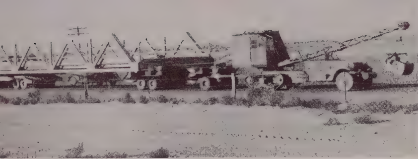
A 70-TON truss bridge was fabricated in the shop and then hauled to the construction site by the road department of Churchill County, Nev. Riding on two 3-axle dollies, the assembly was towed by a Quick-Way Model E dragline.
