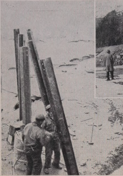
GLACIER CREEK Bridge, above, was constructed near Girdwood, on the Turnagain Arm project. At left, welders splicing built-up steel rails for use on the bridge. Contractor was J. J. Badraun.
