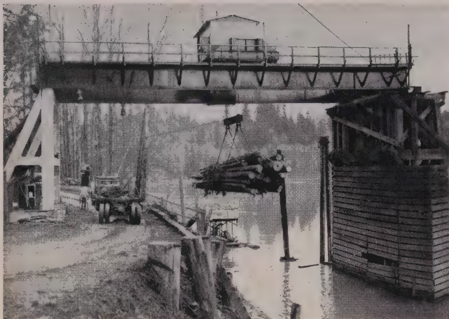
AT THE RIVER , entire load of logs from each truck is lifted by a 60-ton electric crane and dropped into the river. The 75-ft. trackway spans both the road and river.
