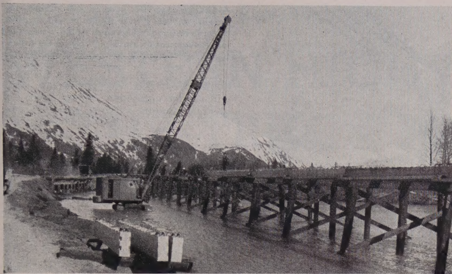
CRANE placing precast concrete stringers on one of the trestles at the east end of Turnagain Arm, this one constructed by Munter & Phillips, subcontractors to Lytle-Green.
