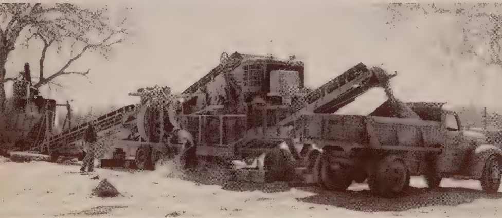
JUST put into operation by Clark County, Nevada, this new Tel Smith 7A Dual Crushing, Screening and Loading Plant, with about 25% to be crushed, is turning out from 60 to 80 cu. yd. per hour when making minus \frac{3}{4} -in. material and from 70 to 90 cu. yd. per hour when making minus \frac{1}{2} -in. material.
