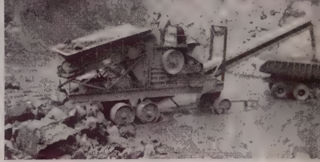
LARGE QUARRY ROCK is reduced to road ballast size by a Lippman Portable Primary Crushing Plant on a Washington highway job. Crusher on this unit is an 18 x 36 Grizzly King. Capacity is 100 tons per hour on hard rock with a 3-in. discharge opening.
