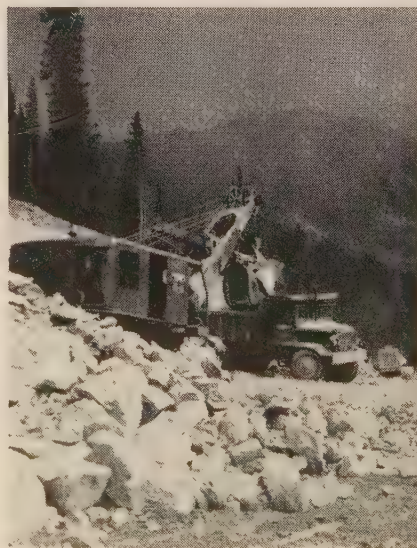
VIEW of construction at 11,000 ft. elev. Extra equipment was required for high elevation.
