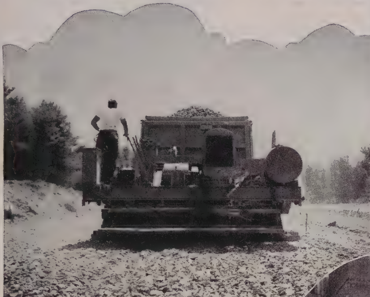
Right: Detail of rubber tired stone attachment.
