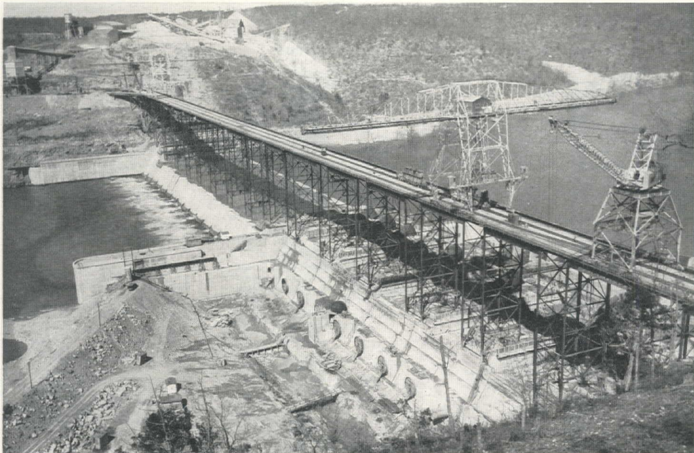
OVERALL VIEW of the Bull Shoals damsite, with about 900,000 cu. yd. of concrete in place. Powerhouse area is in left foreground. Note aggregate and concrete plants on opposite river bank.
