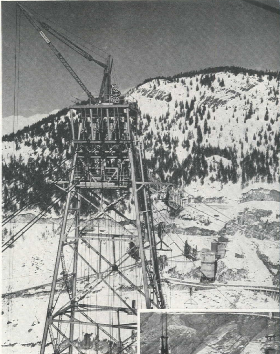
THE 200-FT. main headtower, above. This tower supports three of the four cableways. Visible across the canyon are the right abutment key, concrete mixing plant, and the trackway for the "goose" with the trestle crossing the keyway. AT RIGHT, two 8-cu. yd. Crowe buckets suspended over the Flathead River canyon when concrete was being placed in a fault zone, which can be seen at the bottom of the canyon.
