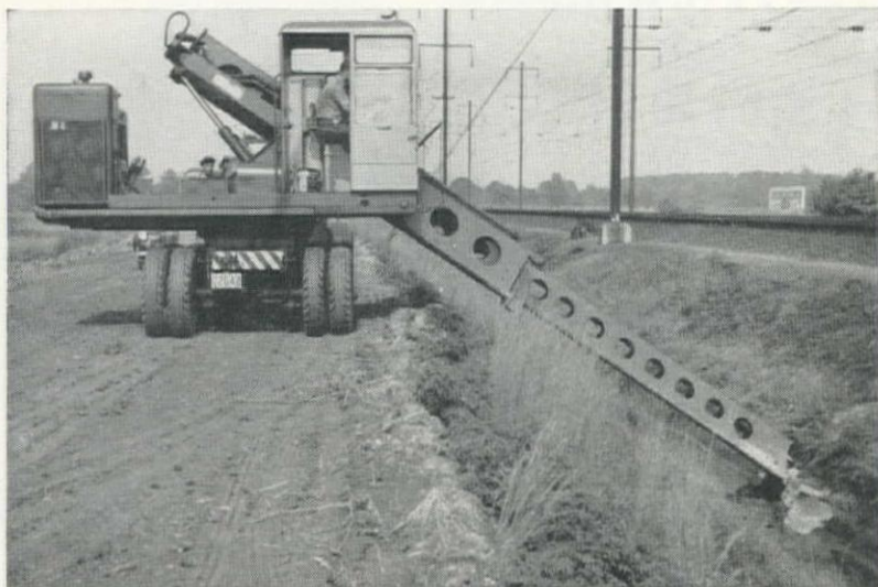
◀ The Gradall stretches far to do a fast, neat clean-out job on ditches.
