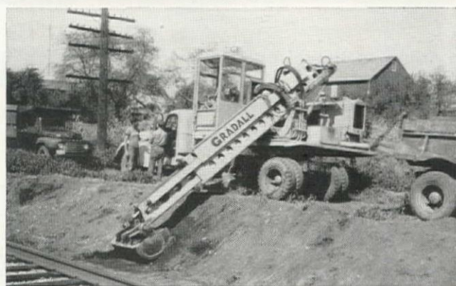
↑ In this restricted location working under low-hanging power lines the Gradall widens bottom and does a precision job following contours of this ditch.
