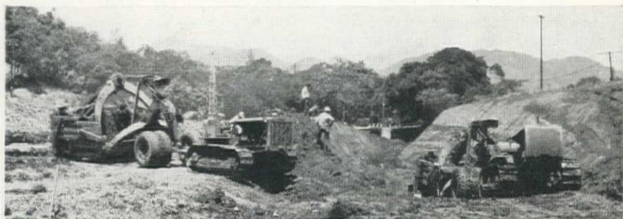
EXCAVATION for relocated channel was handled by LeTourneau Carryalls. The Carryalls, Woolridge Terra Cobras and Caterpillar jeep scrapers combined for the roadway grading.
