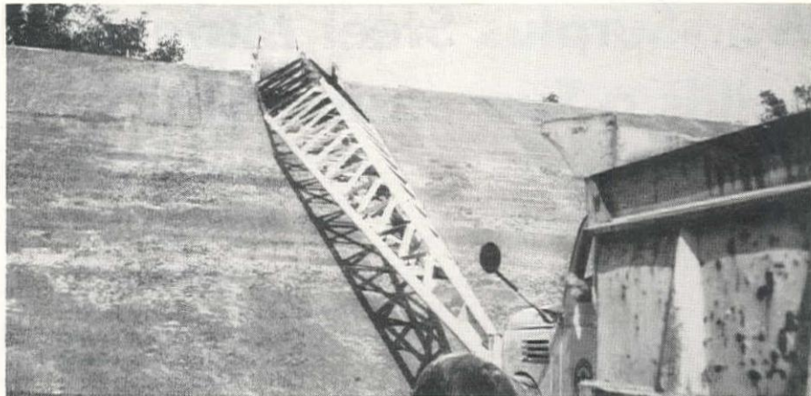
A SPECIAL push boom handles a 6-ton roller on the sub-base of the slopes. A front-end drive truck was found to have ample speed and control to handle the roller.
