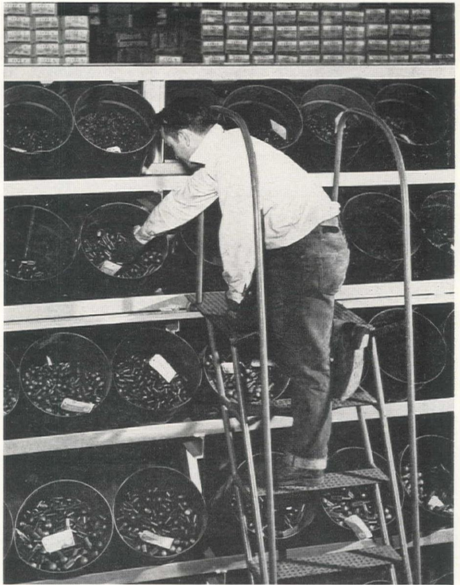
SPACE-SAVING WAREHOUSE RACK USES 10-GAL. STEEL DRUMS
