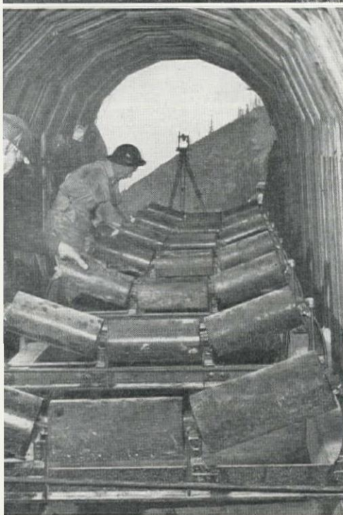
SCREENED AGGREGATE , above, being discharged from conveyor onto a stockpile. Crater is caused by removal of aggregate through a conveyor tunnel. At left, rollers for the 36-in. conveyor belt being installed. Belt delivers aggregate to top of screening mill.
