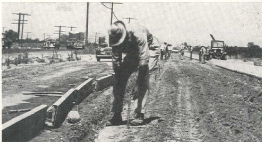
SETTING header boards was done after the subgrade was thoroughly compacted.
