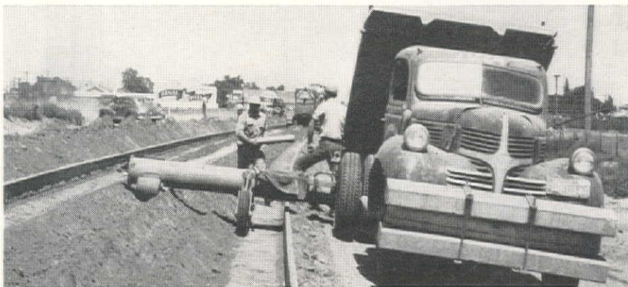
CEMENT SPREADER in operation. Note uniform windrow and undisturbed base.
