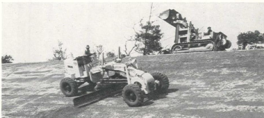
AN AUSTIN-WESTERN 99 motor grader was used to trim 2:1 slope sub-base. Supporting line from tractor on slope berm helped to insure accurate blade work.
