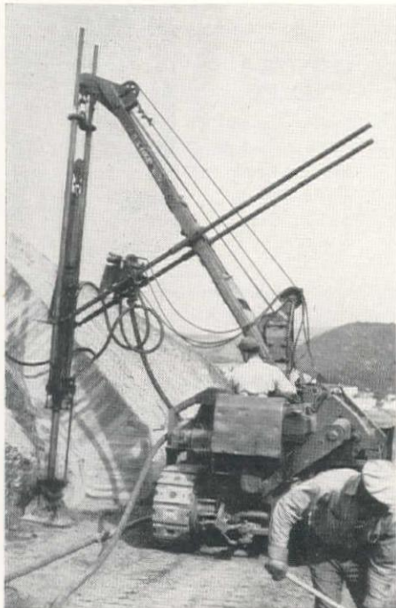
A TRACTOR-MOUNTED compressed air tamper was developed for close-quarter tamping around the cutoff wall and up a V-cut on the slope.
