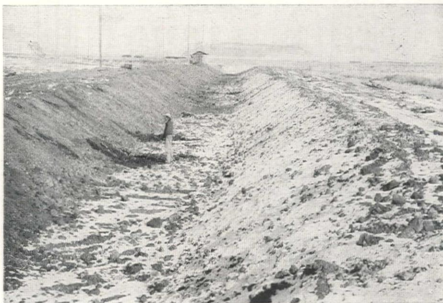
APPEARANCE of completed prefabricated lining installation with a 12- to 18-in. layer of cover material in place. This cover is not compacted when placed, but is consolidated by water action during use. Note snow, indicating cold conditions under which lining was placed.
