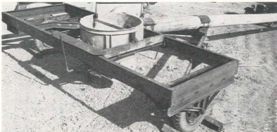
A BOTTOM-DUMP bucket for low-slump concrete was mounted on a frame with a gin pole for placing concrete on the slopes. Frame acts as a crane, allowing side movement.
