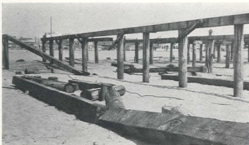
THE RE-SALVAGED piles were also used in 1929 for a pier at Venice, Calif. View above was in 1948 when this pier was being demolished. Piles were still sound after 57 years.
