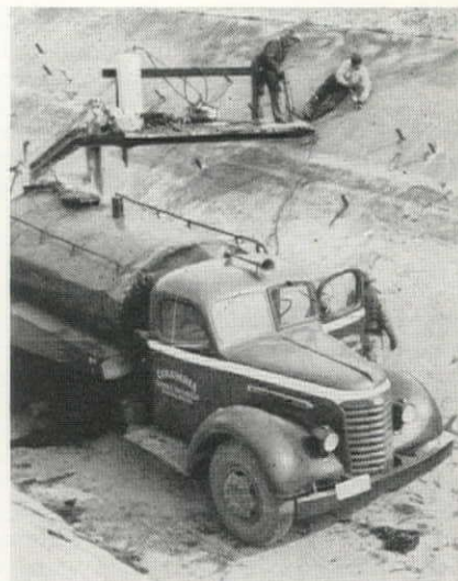
HOLES for application of asphalt on the canal's slopes were reached from a platform attached to a fork lift device mounted on a tractor. In this view, holes are being plugged.
