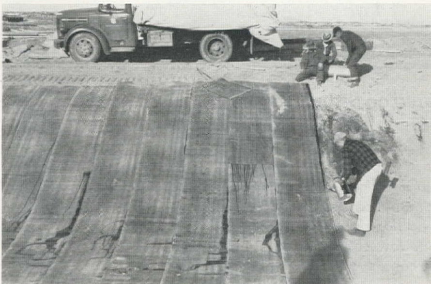
POURING RC-O asphalt cement on lap area between strips. Workmen at top of bank are holding roll of lining which will be rolled down the slope and lapped over edge of sheet in place.
