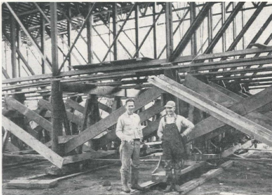
THE THREE elements of the falsework are shown above—steel trusses on a platform of used piling, which in turn was supported on heavy mud sills. Sills were lowered by undercutting and tracks and wheels (left) were inserted for removing the falsework.
