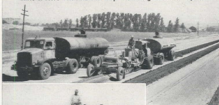
"One-man" pavement construction in California with modern mixers. Note Bitumuls non-stop "refueling" from transport.
