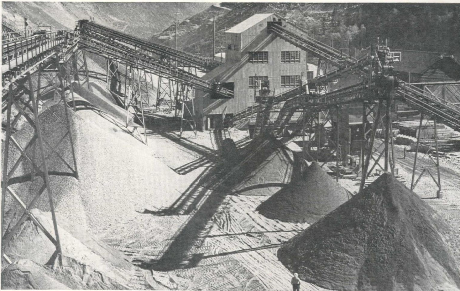
THE SCREENING plant and aggregate storage area. At left are finished product stockpiles. Sand piles on right are, front to rear—medium, coarse and fine. Compare this view with the flow diagram on the opposite page. At right, a general view of the raw aggregate stockpiles and stacker. An underground conveyor carries this material to the screening plant.
