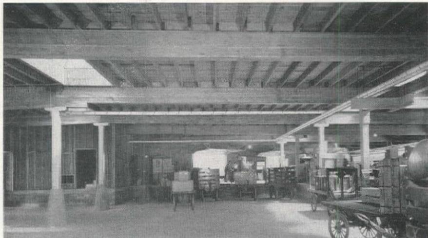
38-foot glued laminated beams support roof structure of freight terminal.
