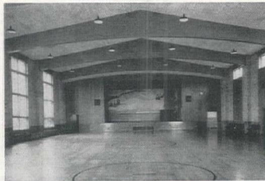
Cambered and tapered beams provide primary structural members for roof of this gymnasium. The Architects: Johnson, Bain, Brady & Grainger, Seattle, Washington.
