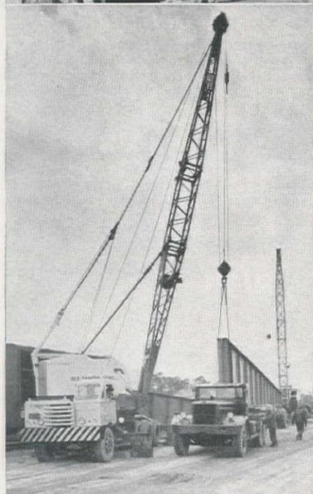
Above: A K-370 and a K-25 operating on barge erecting steel on approach to bascule span.
