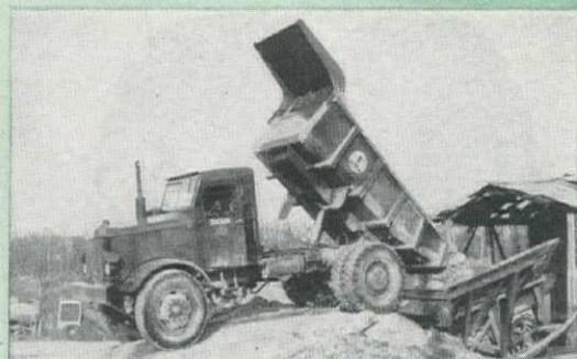
High dumping angle and fast-acting Euclid hoist assure quick dumping. Here the "Euc" dumps a capacity load of limestone into crusher at the H. & R. Stone Company quarry at Ridgeville, Ind.
