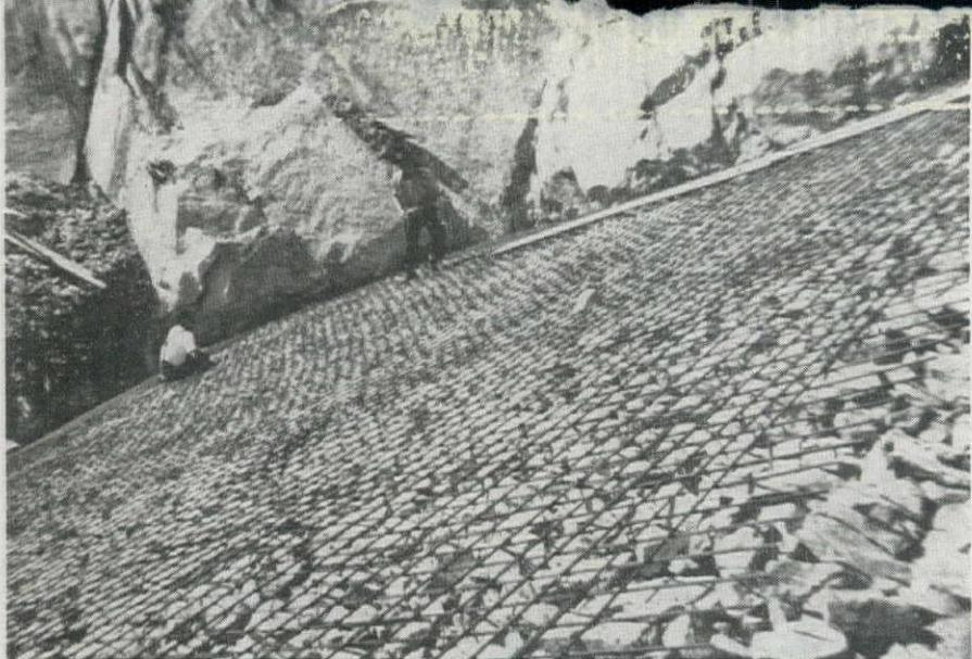
PLACING reinforcing steel on the upstream face of the dam. Completed face consists of concrete with a minimum thickness of 6 in., placed wet and without the use of forms.
