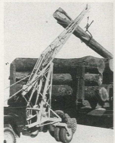
to 12 ft. from the "A" frame. It can be moved with heavy loads suspended in air. No blocks are necessary. A patented "hook-up" feature makes possible use of the entire weight of the truck or tractor for counterbalance. Lifting capacity of the Cradle Boom Handi-Hoist is rated at 6,000. Boom can be set at any angle desired. Can be attached to any make tractor or Willys Jeep.
