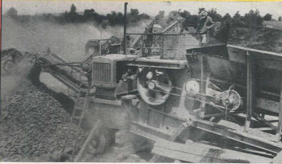
► This "Caterpillar" Diesel D8800 Engine is one of four used to power a crushing plant for the Harms Brothers, General Contractors, Sacramento, Calif. Production averages 1400 tons of  $\frac{3}{4}$  rock in 8 hours. Another D8800, two D13000s and a D17000 complete the reliable, money-saving "Caterpillar" line-up here.
