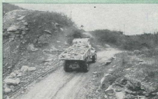
Powered by a 125 h.p. diesel engine, the Model UD has a top speed of 35.7 m.p.h. and plenty of power for steep grades. The 860' haul road at the C. A. Langford quarry near Cookeville, Tenn., has a maximum grade of 10%.
