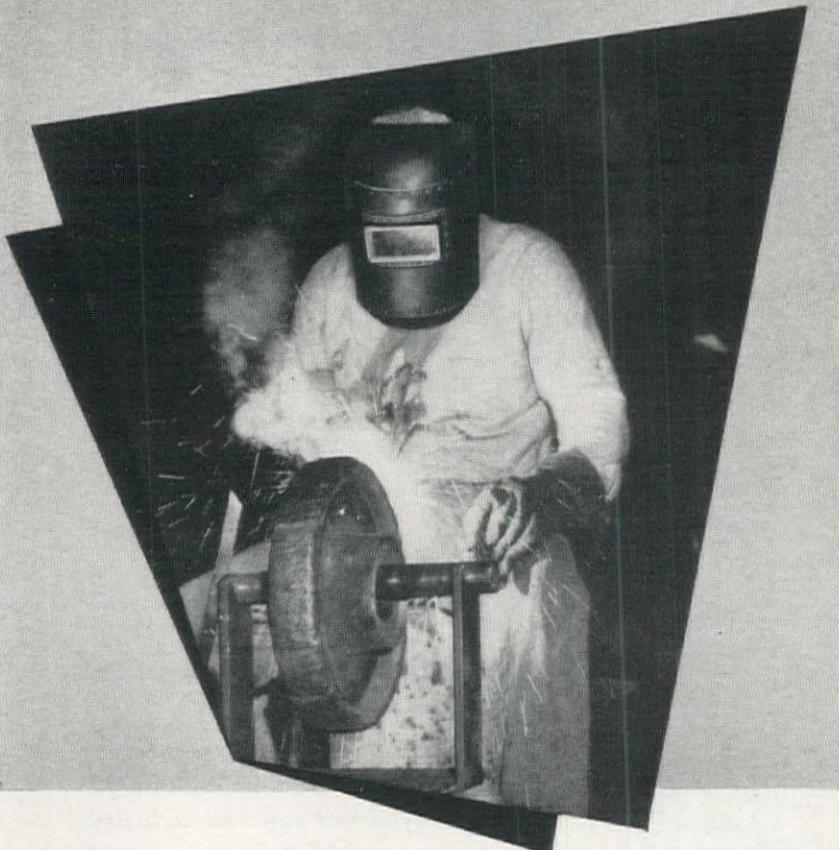
Because of the hardness and other desirable characteristics of these alloys, they provide high resistance to all types of wear—abrasion . . . impact . . . heat . . . corrosion. One application often adds 2 to 25 times longer service life to *worn or new* parts . . . big dividends in savings of “down-time” and replacements.
