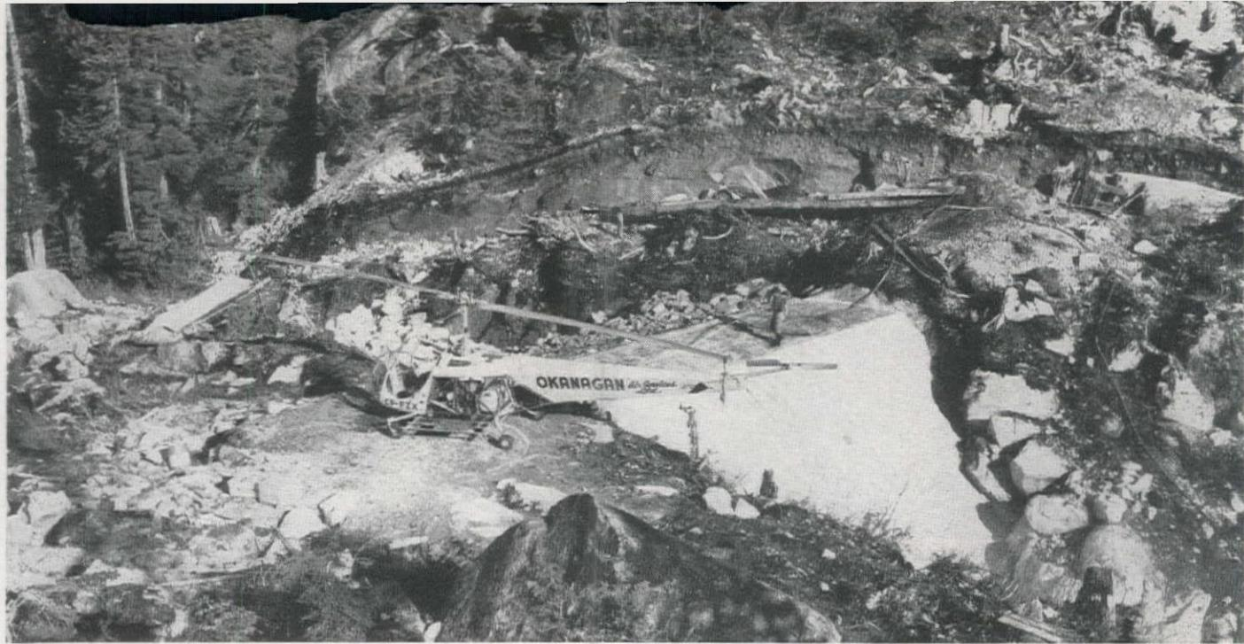
THE HELICOPTER on its landing field at the dam site. The landing spot, originally 10 by 12 ft., was later enlarged by blasting to approximately 15 ft. square at the pilot's request. Visible are the nearly completed dam, foreground, and the cut for the spillway, background.
