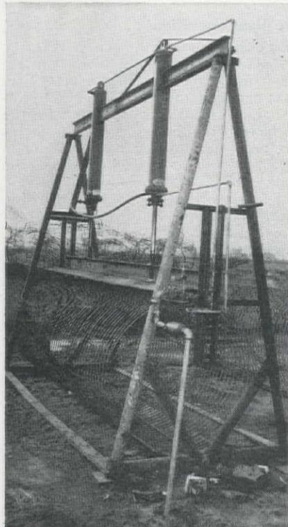
**SPECIAL MACHINE** with automatic spacer wraps spiral reinforcing steel cage for the concrete pipe. Foot control, left, leaves welder's hands free for tacking lateral rod to spiral. An end frame swings off the drum axle when the cage is shaped and the drum form collapses.
