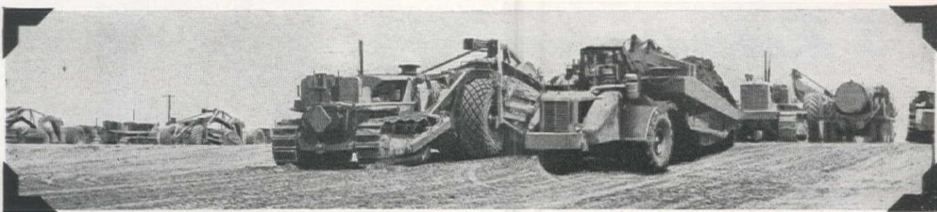
HEAVY-DUTY DIESEL AND GASOLINE EQUIPMENT, owned by 8 contractors, moved over 12,000,000 cubic yards of earth on this cut and fill job—an extension to the Los Angeles Airport—in 13½ months! General Contractors are N. M. Ball & Sons, Berkeley; Harms Bros.,
