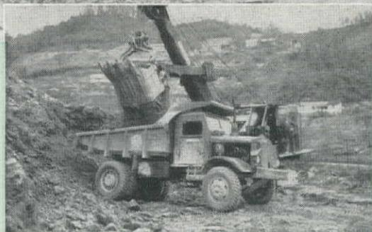
The Acme Construction Company uses this 10-Ton Rear-Dump on a highway construction job at Matoaka, W. Va. The "Euc" is loaded with earth and shale by a 1 1/4 cu. yd. shovel.
