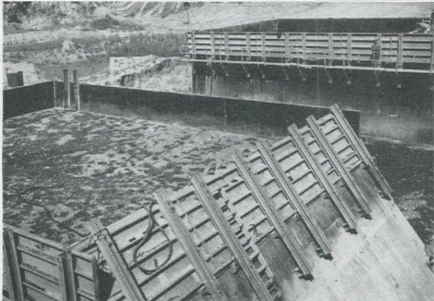
POURING CONCRETE for the spillway monoliths. Top, one of the cranes unloads a bucket of concrete from a flatcar, which travels on two sets of railroad rails within the widespread rails for the big cranes. Note use of steel forms for monoliths in view at bottom.
