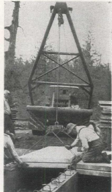
PLACING the first panels of the deck. As erection proceeded, the crane-truck was run onto the newly-set panels. Unloading panels at the site required four working days; erection required another four working days.
