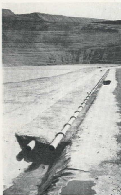
DRAINS in the reservoir floor on top of the membrane will collect and deliver any seepage to the outlet works.
