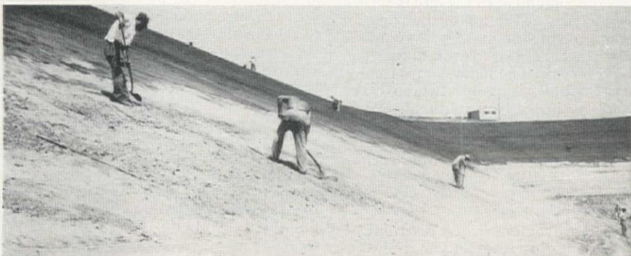
HAND-TRIMMING finished inside slopes preparatory to membrane application.
