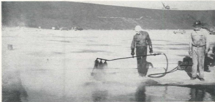
SPRAYING seal coat on reservoir floor preparatory to placing gravel blanket.
