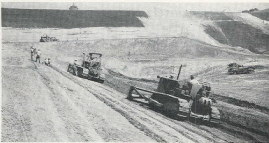
TRACTOR-GRADERS handled accumulated material for grading near the bottom.
