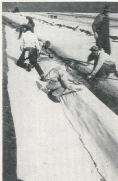
LAYING cotton cloth reinforcement before spraying of the final seal coat.
