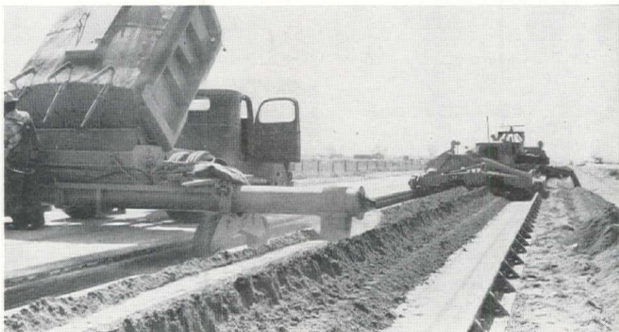
ANOTHER TYPE of distribution for applying bulk cement operates with a screw conveyor supported on out-board wheels depositing into a trough left when the windrow was formed.
