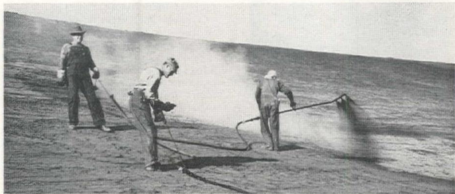
SPRAYING final asphaltic seal coat on an inside slope to complete membrane.
