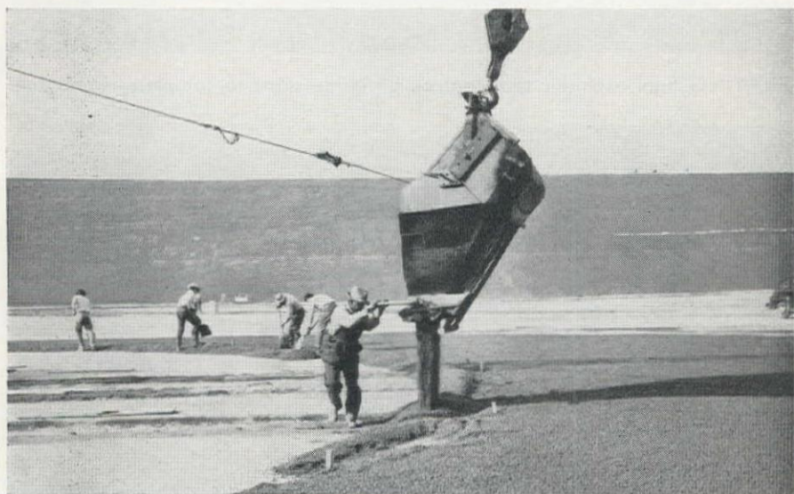
PEA GRAVEL blanket spread on top of membrane will conduct seepage to drains.
