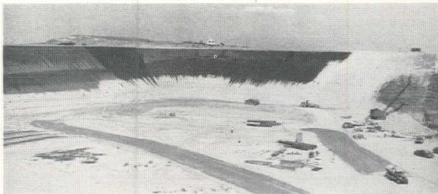
VIEW across the reservoir area showing part of the asphaltic penetration coat.
