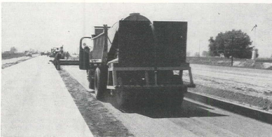
FINAL COMPACTION by pneumatic-tired roller provides a harder surface with better texture.
