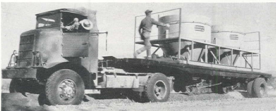
CEMENT is applied from containers mounted on a distributor which is geared to place on the windrow a pre-determined amount per square yard of base to be treated.
