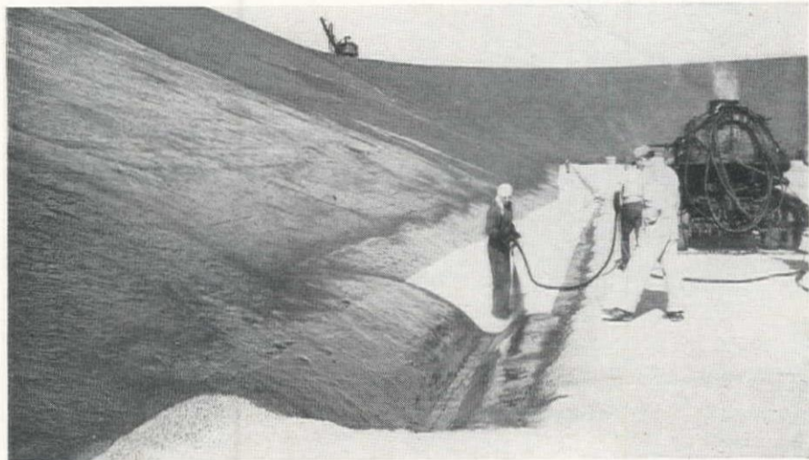
SPRAYING final seal coat on cloth reinforcing in ditch at toe of inside slope.
