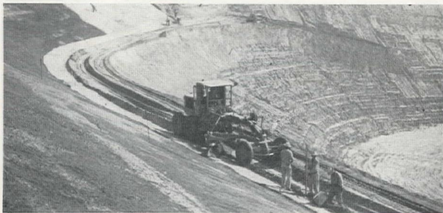
HORIZONTAL rough grading proceeded from top to bottom of the inside slopes.
