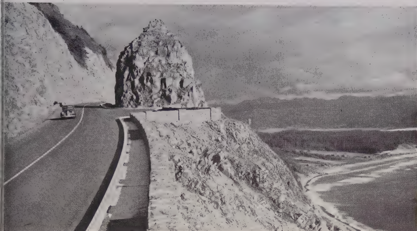
U. S. 101 along the Pacific Coast in Oregon. Rough terrain is only one of the problems facing Western road builders.
