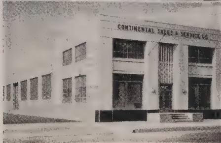
B. F. TOBIN, JR. , upper right, is President of Continental Sales & Service Co.; HARVEY N. HOLT , left, is Vice-President. Facade of the firm's new headquarters building, bottom.
