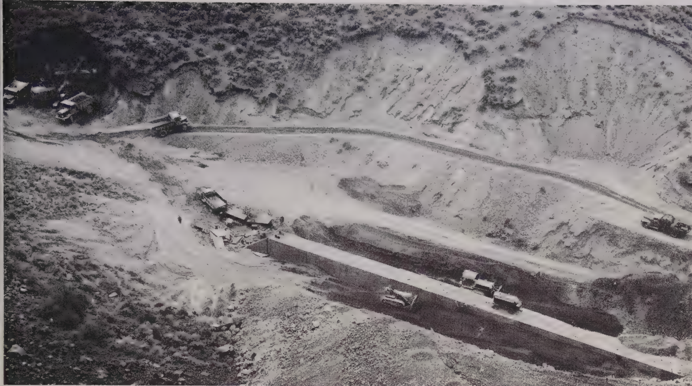
EXTENSIVE grading over long stretches of rough terrain requires a variety of heavy equipment for Western highway construction. Illustrated is the construction of a box culvert by Peter Kiewit Sons' Co. for highway relocation on the Grand Coulee Irrigation Project in Washington.
