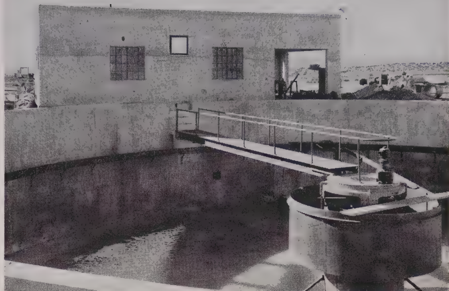
THE INGENUOUS design of small sewage disposal plants is exemplified by this plant at Santa Fe, N. Mex. Two "Caterpillar" gas-operated electric sets provide the plant's power.
