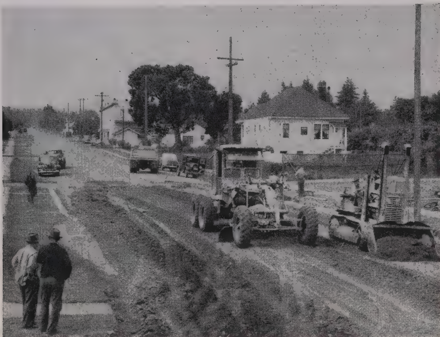
MANY Western cities will place special emphasis on street construction during 1950. Illustrated is a typical street grading operation—this one at Port Angeles, Wash.
