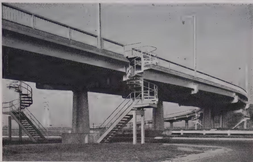
BY-PASS STRUCTURES combining efficiency and pleasing appearance are being constructed on major routes throughout California. Illustrated is a structure on U. S. 101 near San Mateo.
