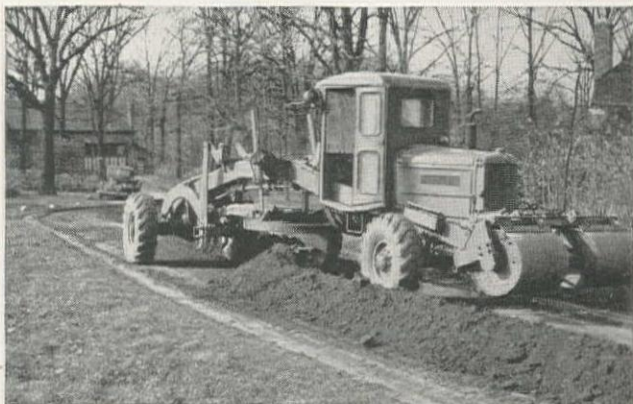
Using All-Wheel Steer to offset the front and rear trucks enables the A-W machine to do superb finishing on any slope. In the picture above, the grader is finishing an inslope, working up from the ditch, leaving no tire marks to mar the surface.
