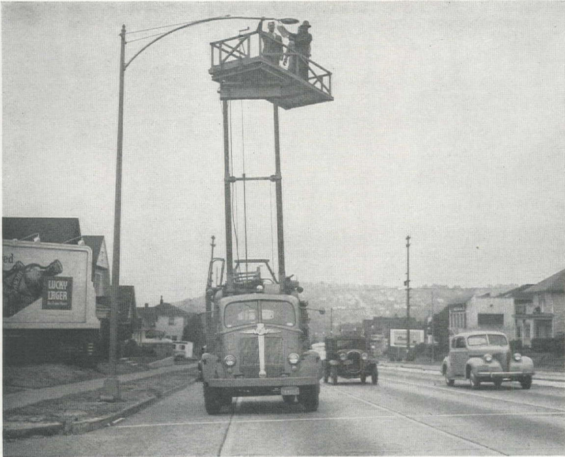
WITH A LIFT of 30 ft., this hydraulically-operated truck platform is used for installation and maintenance.
