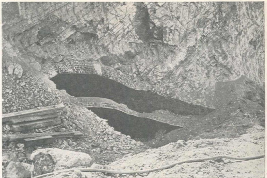
BRICK ARCHES of original (1901) and modified cross-sections of Broadway Tunnel (1916) as demolition approached the north portal surprised engineers with their strength.
