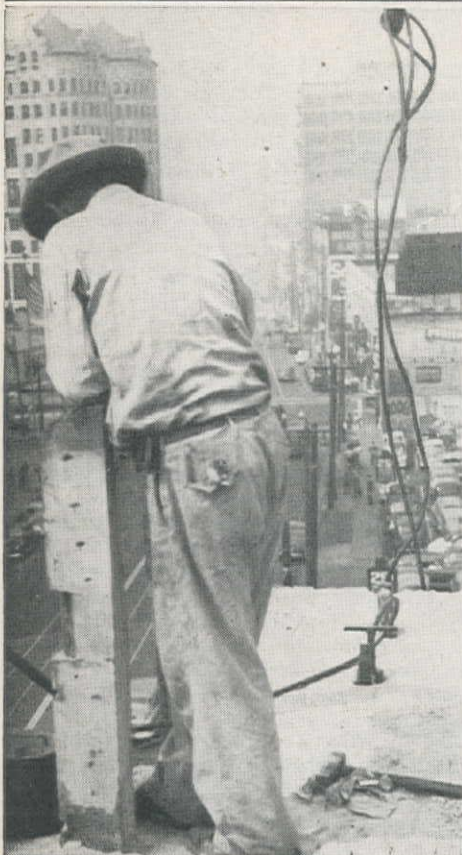
HYDRAULIC PRESSURE unit for demolishing concrete at Broadway tunnel portal. The Roc-Jak (top) includes ten pistons which are expanded in a 3½-in. hole previously drilled by jackhammers. The hand-operated Roc-Jak, (lower left) produces pressures up to 150 tons in a 2-ft. hole, and breaks off a whole corner section of concrete portal wall (lower right).
