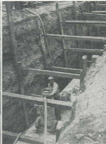
GROUND WATER conditions emphasized the need for careful jointing. Concrete pipe was trucked from a local yard (left) and laid up with a Nicholson Groutweld machine (right).
