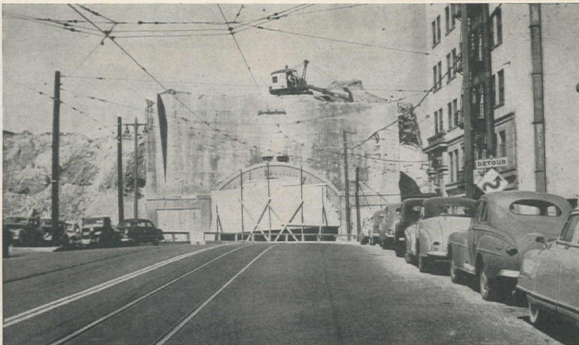
WORK STARTS on the south end of old Broadway Tunnel, which was removed as part of the project that removed Moore Hill. The populated district precluded the use of blasting to remove the concrete of this famous structure first opened in 1901.
