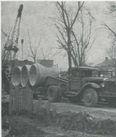
GROUND WATER conditions emphasized the need for careful jointing. Concrete pipe was trucked from a local yard (left) and laid up with a Nicholson Groutweld machine (right).
