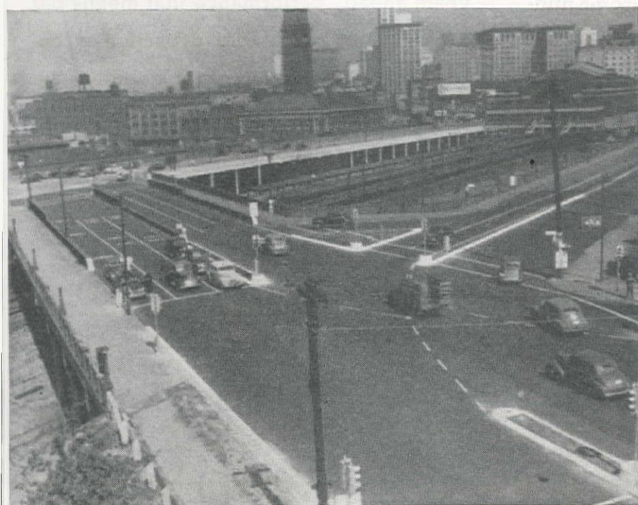
AFTER— Same intersection after the application of modern traffic engineering, showing channel islands, traffic-actuated signals, and striping.
