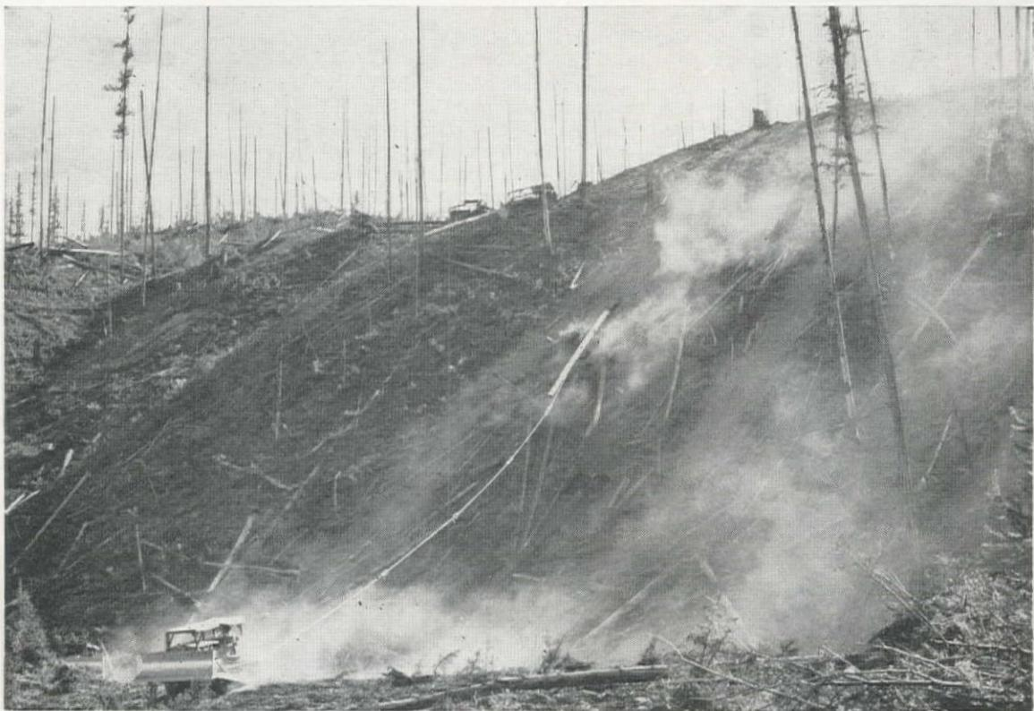
DRAGGING an 800-ft. loop of 2-in. cable, equipped with swivels at 100-ft. intervals, down a snag-covered slope was the unique development of a contractor in clearing thousands of acres of burned-over land in the reservoir site.
