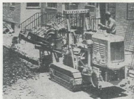
and 10 to 20 in. wide. Other new features are: Clog-proof crawler tracks; operator-controlled conveyor giving instant control of the spoil bank; patented "Presto-Points" for quick and easy replacement of rooter teeth, and a crumbing shoe giving perfect grading and clean trench bottom, and which can be swung up and away to permit digging right up to foundation, walls and trees.
