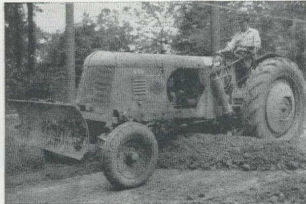
Huber's versatile Road Maintainer—a lift loader, berm leveler, bulldozer, patch roller, snow plow, or rotary broom all in one.
