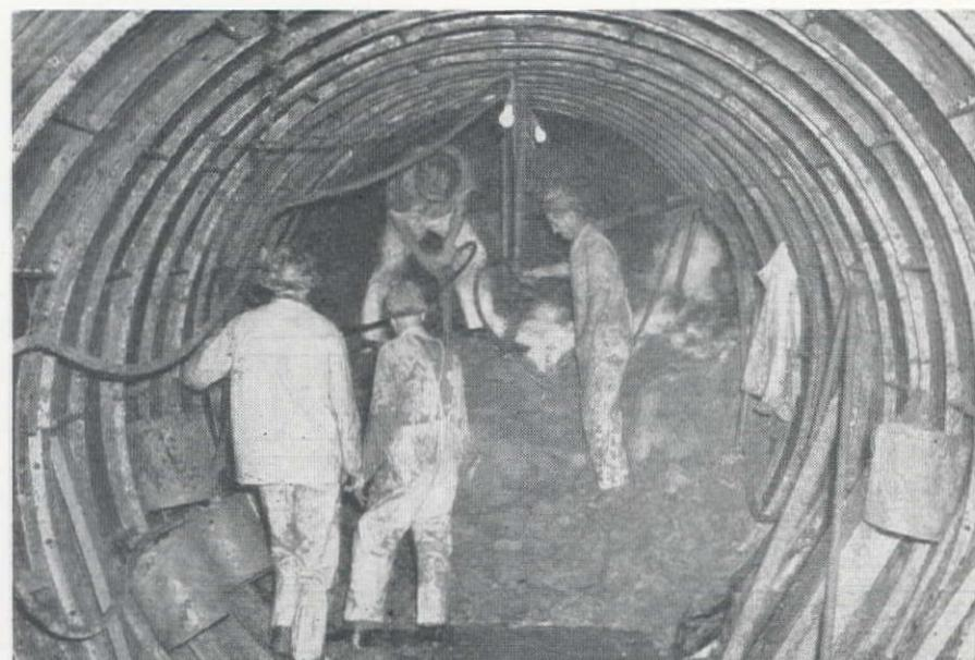
plate, precast sections of pipe, and placing of concrete backfill into the space between the outer wall of the pipe and tunnel lining. The section of tunnel described here called for 84-in. I.D. pipe with a wall thickness of 7 in. This left a working space of 8 in. between pipe and tunnel lining.
