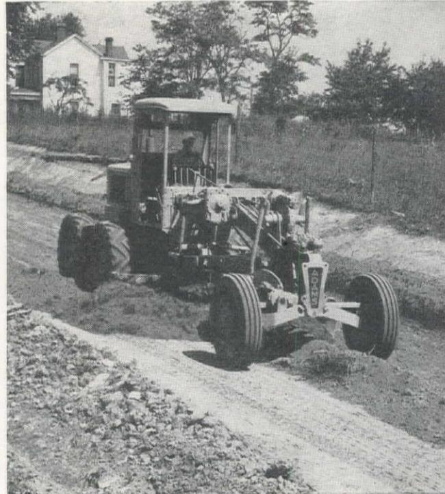
In the picture above, Mr. Perley Dodge poses with the Model 101 Adams Motor Grader which for 19 years he operated for Columbia County, Wisconsin. Despite approximately 39,000 working hours, this machine required only normal maintenance service.
