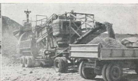
When fitted with shovel-loading hopper, the "201" Plant is completely portable. No parts need be removed for transporting.
