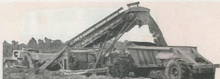
GM Diesel-powered Euclid loader, pulled by Allis-Chalmers HD-19 tractor, teams up with 7 GM Diesel-powered Euclid bottom dumps to move as much as 150,000 yards of earth a month.
