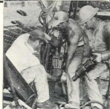
Heavy-duty CP Air Impact Wrench easily runs nuts up to 1 1/4" bolt size. CP Pneumatic Corner Drills speed drilling and reaming operations.
