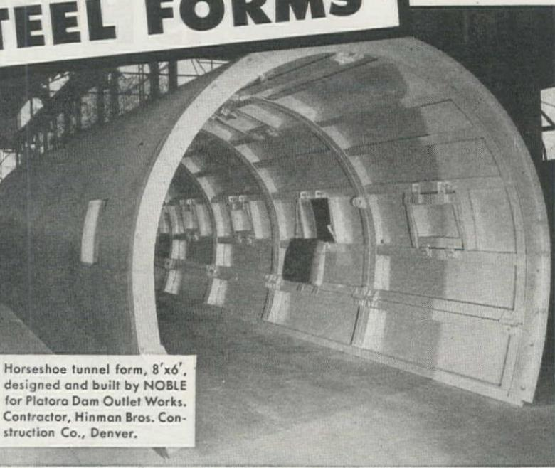
Horseshoe tunnel form, 8'x6', designed and built by NOBLE for Platora Dam Outlet Works. Contractor, Hinman Bros. Construction Co., Denver.
