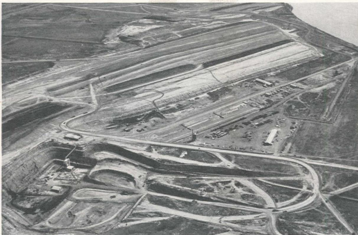
WITH 10,000,000 cu. yd. in place the embankment and powerhouse excavation in the foreground, this aerial view shows the general area of operations.
