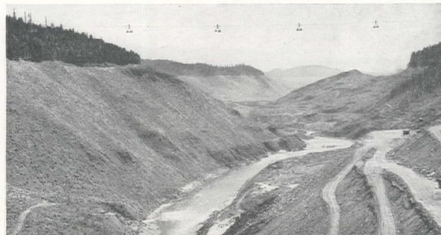
snags and brush not already loosened. In the bunching operations the rakes loosened and shook the dirt and rocks from the roots, permitting clean burning in the piles. Fire was permitted to run through one area after the de-snagging operation had been done, after which the tractors moved in and rooted and bunched the remaining stumps and unburned tree trunks.
