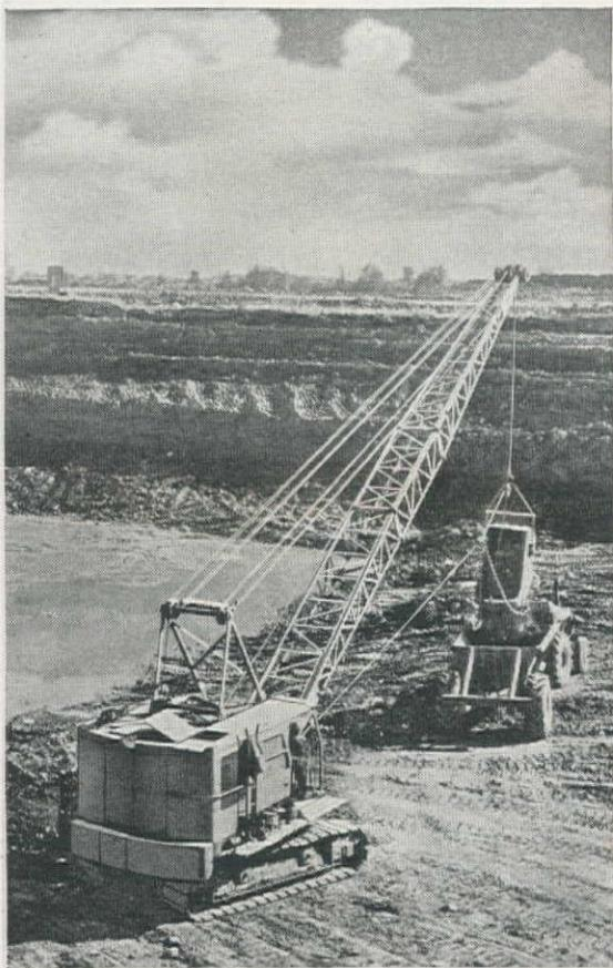
GM Diesel-powered Koehring 605 dragline with 1 1/2 yd. bucket, loads shale in Euclid bottom dump. The GM Diesel-powered Euclids haul 17 yard loads up a 15% grade climbing out of the cut.
