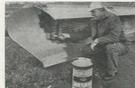
spray gun. It also acts as an effective means of preventing rust. It helps to prevent the piling up of snow and eliminates costly delays necessitated by "clearing" or breakdowns from overloading. A plow may be placed in operation within 20 min. after application of the wax.
