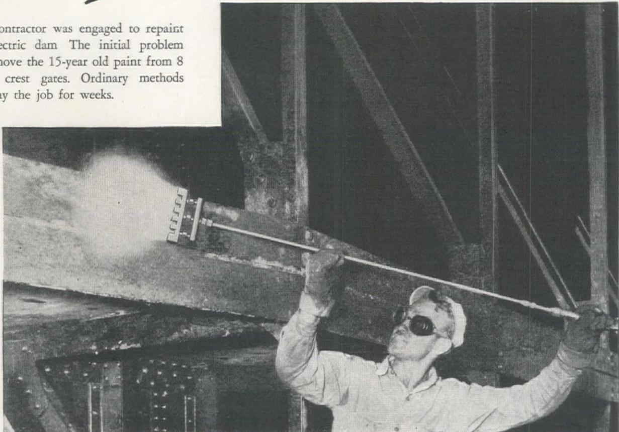
The Airco Technical Sales Representative suggested oxyacetylene flame cleaning with Series 9200 Torches and Airco Style 120 tips. Quickly and easily applied, the intense heat of the flame cockled the old paint, loosened scale and drove off surface moisture in a single operation.
