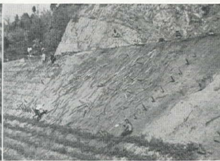
SOIL LOSS on this slope was 17,000 cu. yd. during one heavy storm. The slope was graded, sloped and wattled, right, so that ten years later, losses are negligible.
