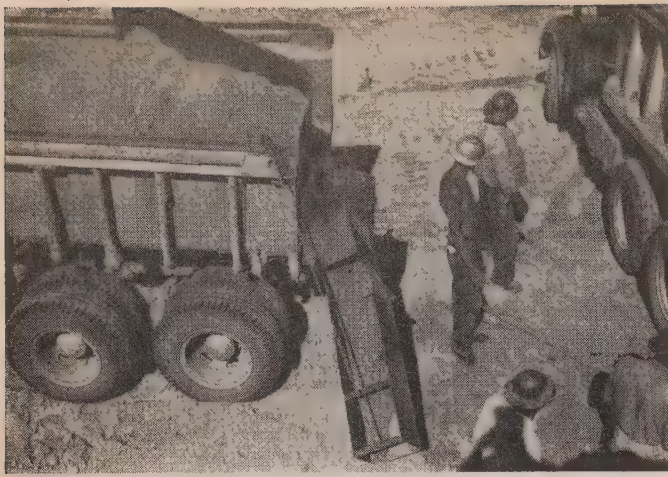
A SPECIAL SAND SPOUT attached to a truck is used for placing sand in the thin filter blanket along the slopes of rock fill on the north abutment at McNary Dam on the Columbia River near Plymouth, Wash., by McNary Dam Contractors. The spout enables crews to put the sand where it is needed in just the amount that is needed. Sand is guided into a hopper box by baffles on the dump body, and a chain from the edge of the body connected to the end of the spout positions the gadget.
