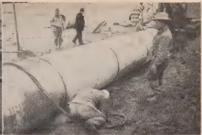
Engineer's office, figure the chances of getting in 200 ft. of pipe before the tide stops the job. At right, N. COLUCCIO supervises guniting of one of the joints of the 42-in. pipe. Trenching in the beach sand was done with a Model 25 Northwest crane, rigged alternately with a dragline for excavation and a sling for lifting and placing each section of the pipe. This particular outfall is one of many improvements being built by the City of Seattle to increase its present system.
