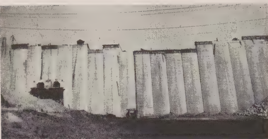
AT FRANCISCO MADERO DAM , a round-head buttress-type structure, use of efficient low-heat cement and an appropriate system of contraction joints saved 2,000 tons of reinforcing steel.
