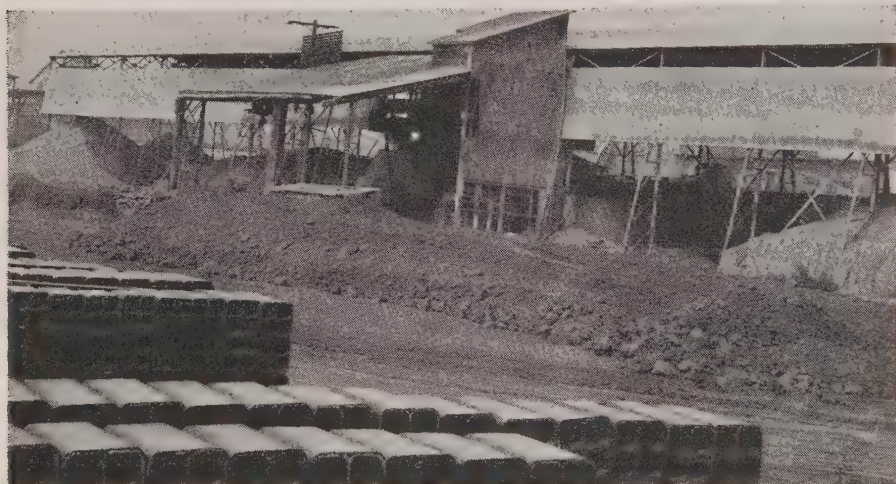
THE HUGE CRANEWAY, almost 1/4 mi. long, that is used for production blending of the clays, is shown in the background above. Below, a stack of finished pipe ready for shipment, left, and a series of the periodic kilns in which the pipe products are fused, right.
