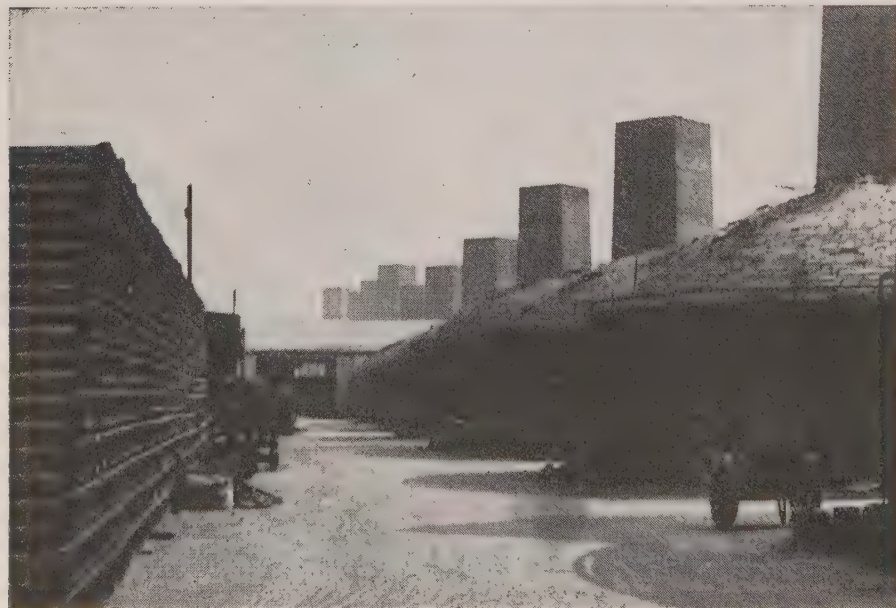
THE HUGE CRANEWAY, almost 1/4 mi. long, that is used for production blending of the clays, is shown in the background above. Below, a stack of finished pipe ready for shipment, left, and a series of the periodic kilns in which the pipe products are fused, right.
