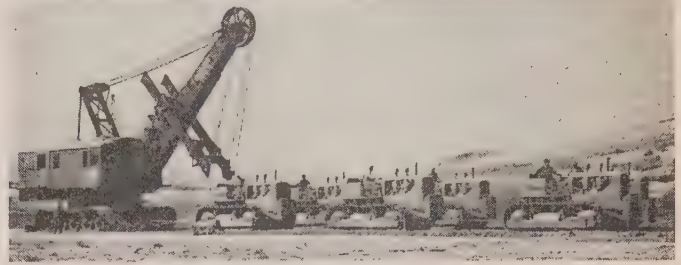
SIX ALLIS-CHALMERS HD-19 tractors teamed up recently to move this 400,000-lb. Bucyrus-Erie shovel into place on construction of river embankments at the Garrison Dam Project on the Missouri River in North Dakota. Contractors for this portion of the job, Peter Kiewit Sons' Co. and Morrison-Knudsen Co., Inc., have three of the big shovels on the job. The dam's embankment will be the world's largest rolled earthfill.
