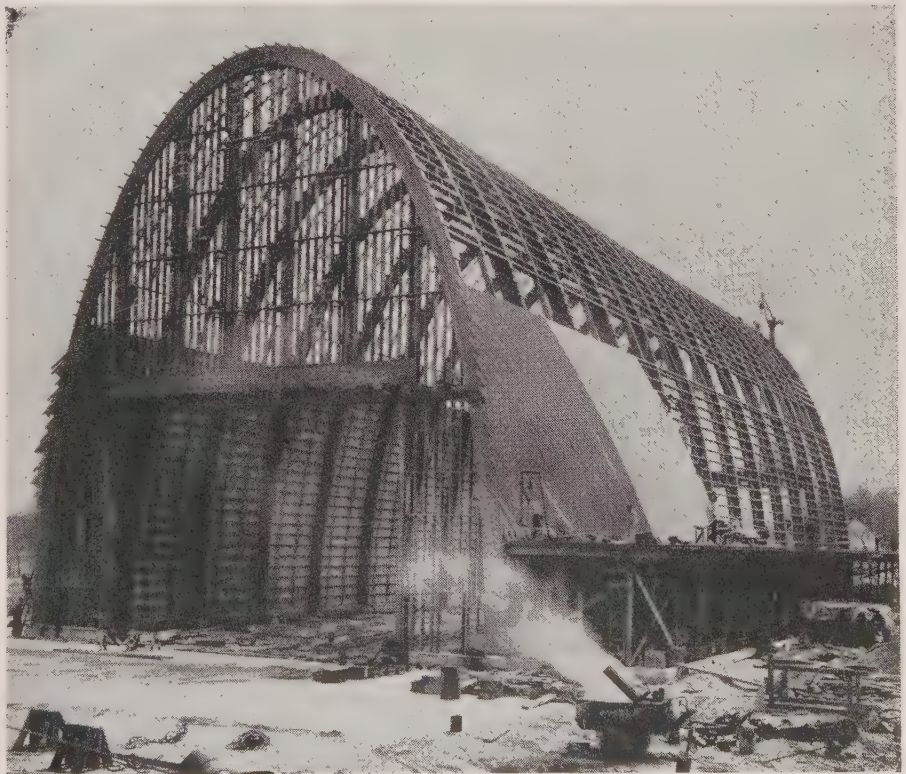
ELLIPTICAL GLULAM ARCHES of the Radar Research Laboratory at Dayton, Ohio, have an 80-ft. span and an 80-ft. rise. Unobstructed space within is the desirable result.
