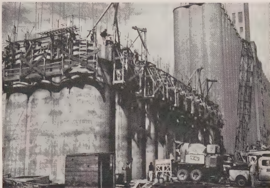
THE ELEVATOR BINS, 52 in number and looking like a series of parallel tubes, are shown half completed. Transit-mixed concrete was being delivered at this stage at the bottom of the bins.
