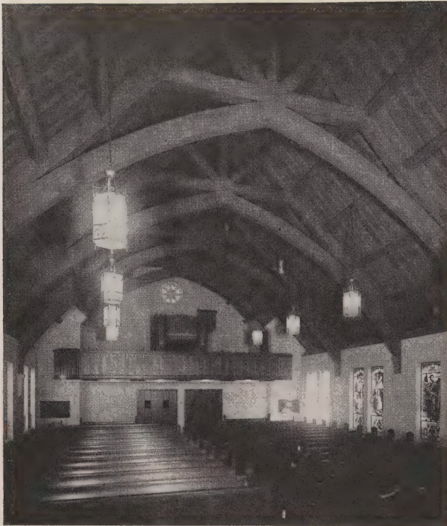
TRUSSES AND PURLINS of glulam give a pleasing effect at St. Paulus Evangelical Lutheran Church, Oakland, Calif. The timbers enabled design of a steep pitched roof.
