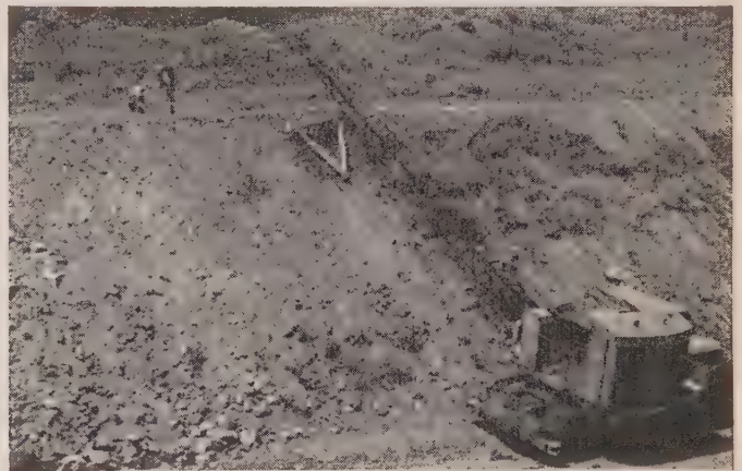
A HEAVY ROCK RAKE is being used by Western Contracting Corp. of Westley, Calif., to finish to rough grade canal banks on the Columbia Basin Project near Ephrata, Wash. A Bucyrus-Erie mobile crane casts the rake somewhat in the way a dragline bucket is handled. Spike teeth on upper bar of the triangle pull rocks and earth to where they can be loaded into trucks. The excavation is then ready for the trimmer jumbo which follows to excavate to fine grade preliminary to placement of the concrete lining.
