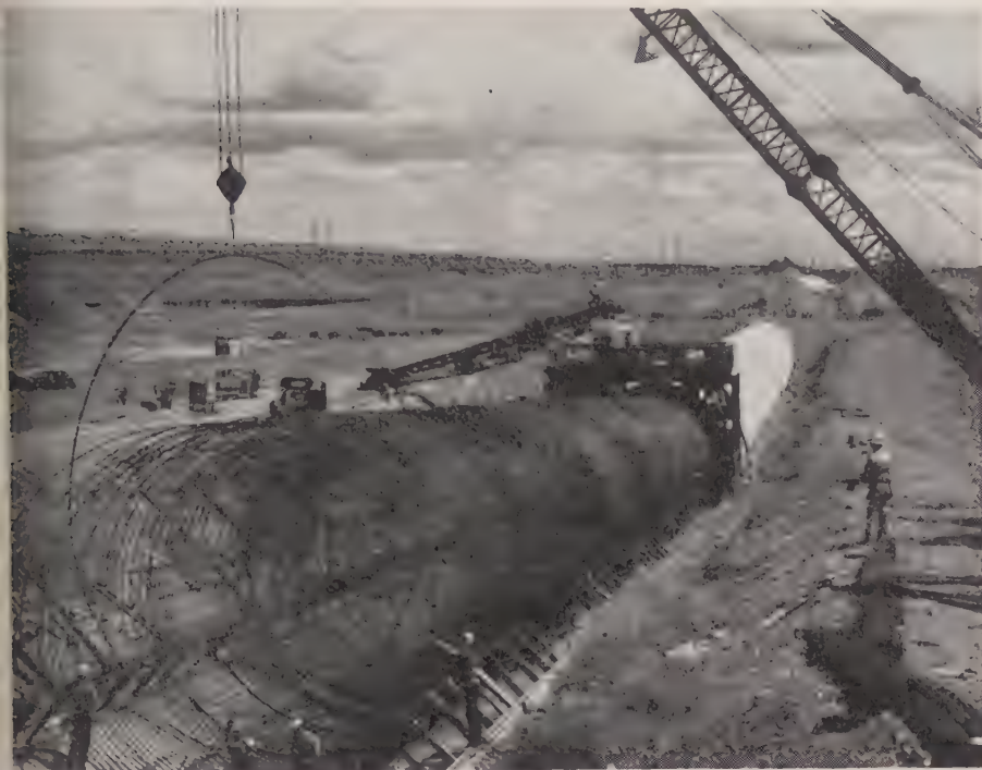
Part of nearly five miles of siphons for Columbia basin
