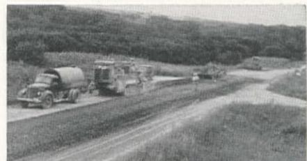
IOWA . . . soil-cement . . . a P&H Stabilizer completed a 10-mile, 24-foot road in only 20 days.
