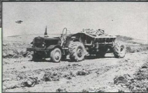
High speed is maintained with a load of 12.8 bank yards of heavy excavation at an airport job in Tennessee.
