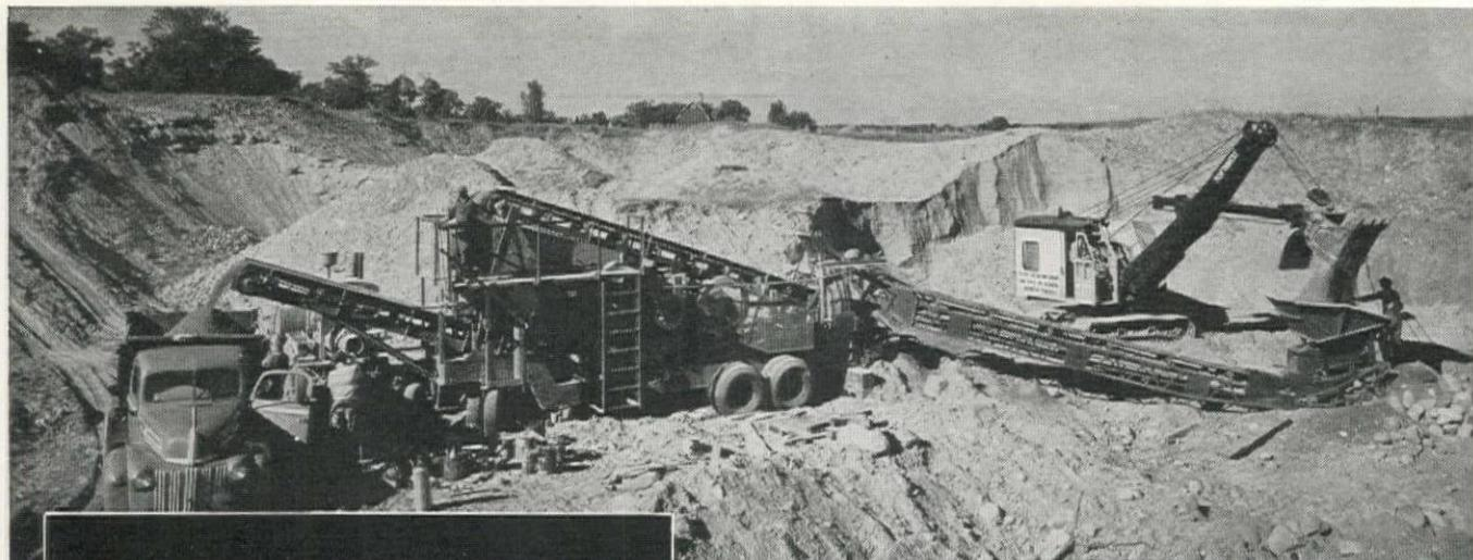
Fisher Bros. Construction Co., Farmington, Minn., using Telsmith Dual Portable with standard truck-loader and field conveyor.
