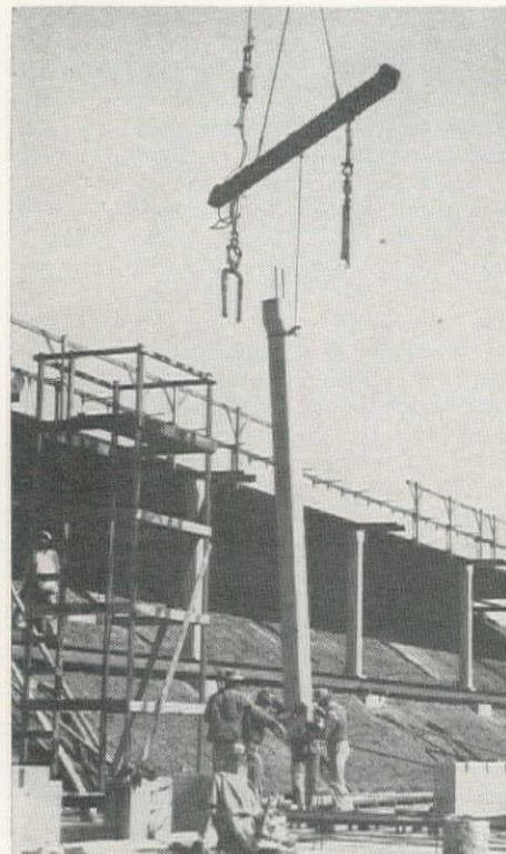
A PRE-CAST COLUMN is lowered into place, left. At right, a girder is guided into position by means of two dowels left projecting from the column tops (visible at left).
