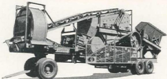
Featuring three stages of reduction with jaw crusher for primary crushing and Universal's exclusive TwinDual rolls for two stages of secondary crushing. Produces money-making volume of finished aggregate for road surfacing, concrete work, etc. Also used with great success in gravel pits containing material which requires a large opening primary. The 293-Q has proved its performance over the years. Capacity—125 t.p.h. 1".
