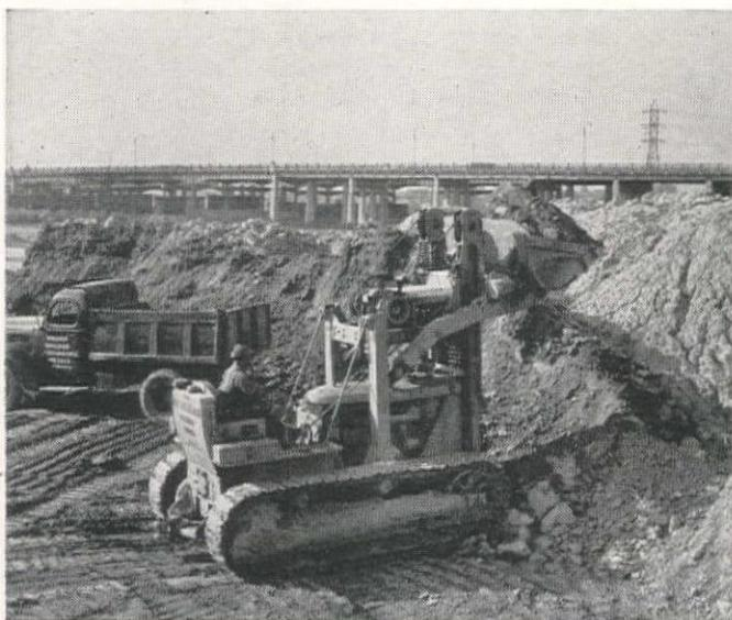
**T6 TRAXCAVATOR** loading "fill" material on Toronto, Ont., Can. project. The power in the "Caterpillar" D6 insures ample digging and loading push.
