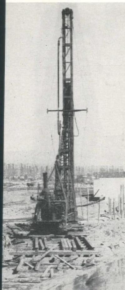
HIS 100-FT. TALL Raymond Universal Pile river is being used to place the step-taper, cast-in-place piles, about 95% being battered.
