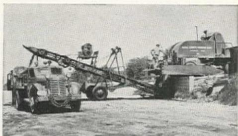
The Moto-Paver is a very flexible as well as a mobile unit. The illustration shows it being used as a stationary mixing plant.
