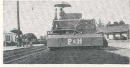
CALIFORNIA . . . bituminous . . . a P&H Stabilizer reprocessed a 10-year old "oil-mat" to a 3-inch depth at a rate of 1000 sq. yds. per hour.
