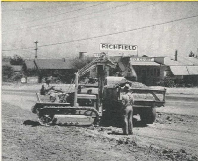
**T2 TRAXCAVATOR** on road widening job in Walnut Creek, Cal. Smallest size in the TRAXCAVATOR family—powered by "Caterpillar" D2 tractor.
