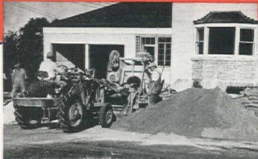
Model "SI," above, loading cinders from stockpile. Model "VAI," at left, is used to charge mixer, fill and level sub-grade for sidewalks, etc.
