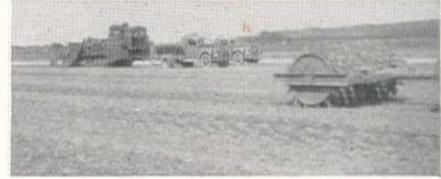
NEBRASKA . . . clay-gravel . . . the sub-base of this airport was processed at 1900 sq. yds. per hour with a P&H Stabilizer.
