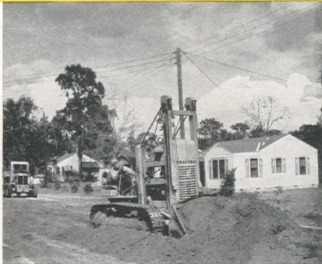
**T4 TRAXCAVATOR** on "Caterpillar"-D4 tractor street grading in Orlando, Fla. Note amount of dirt bucket is pushing ahead and easily handles.
