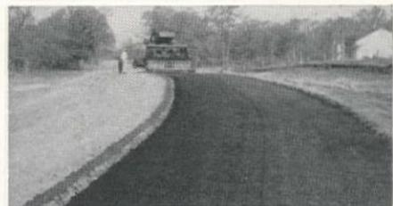
TEXAS . . . bituminous . . . a P&H Stabilizer processed a state highway project at a rate of 8000 sq. yds. per day.
