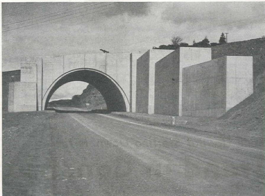
PLEASING LINES were the result of using a reinforced concrete earthfilled arch structure for this underpass. Chief competitor in preliminary design was a three-span steel girder.
