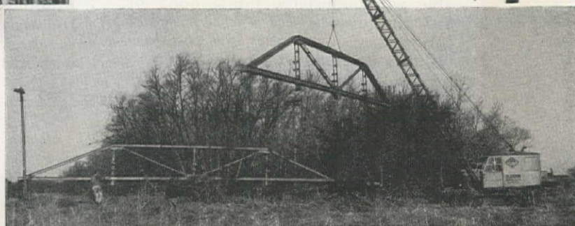
Placing 75 ft. Trusses weighing about 7500 lbs. each. Trusses had to be lifted over telephone-wires.
