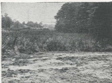
Mud wave pushed out by settlement of fill
