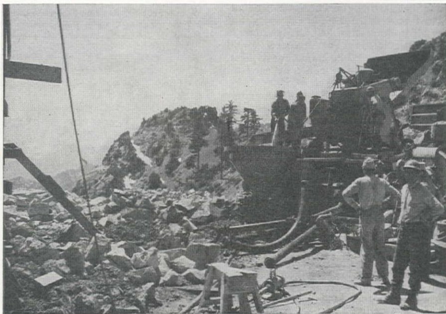
INMATES hose out Pumpcrete unit for cleaning between pours on the tunnel lining. Tunnel portals are made of shaped rubble masonry. At left, HARRY D. JOHNSON, construction superintendent.
