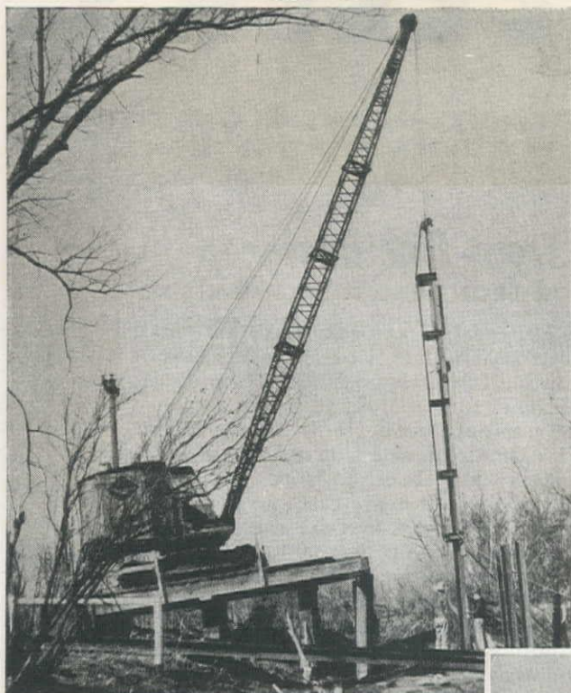
Driving 50 ft. Piling (10" H Beams) for the piers. 55 ft. Boom, 32 ft. Leads. 3300 lb. Drop Hammer, 700 lb. Pile Cap.
