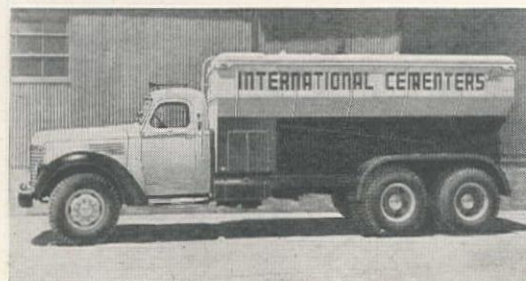
Direct truck chassis mounted aerated units used by International Cementers, Inc., Long Beach, Calif., as front unit of 4-wheel trailer train.
