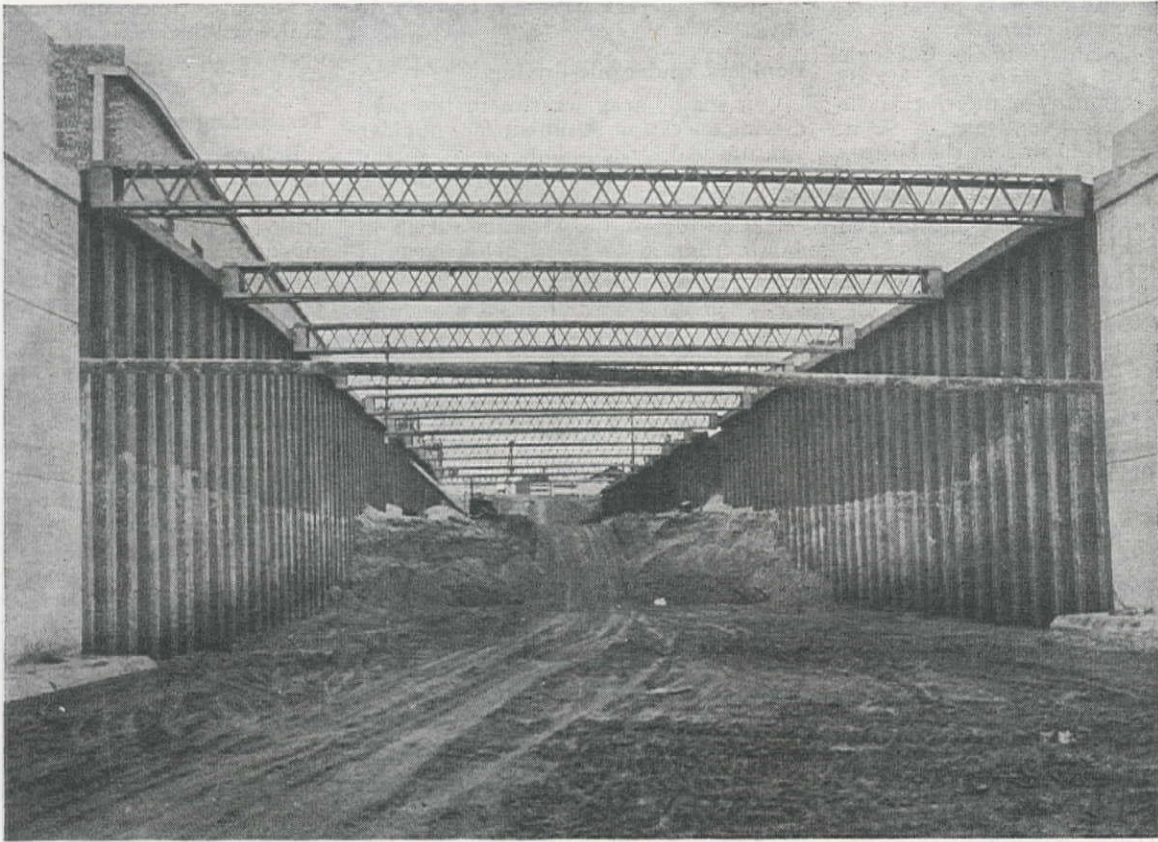
STRUTS begin where steel walls meet concrete in foreground. Visible 8-in. gas main has yet to be moved.
