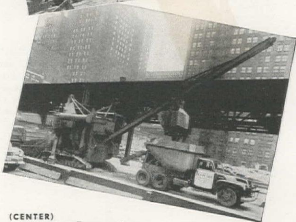
(CENTER) Feeding two Pumpcretes on a sewer job.
