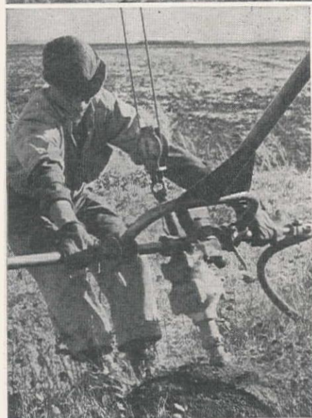
THE COMPRESSOR-AUGER team, above, operated by two men, has stepped up production of anchor holes from 8 to 42 in an 8-hr. working day.
