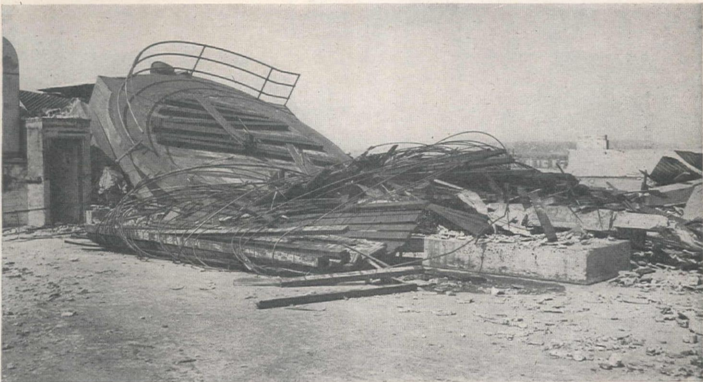
WOODEN water tank above cold storage warehouse collapsed when its 18-ft. reinforced concrete columns failed. One of the columns was hurled 50 ft. Water ruined material stored below.
