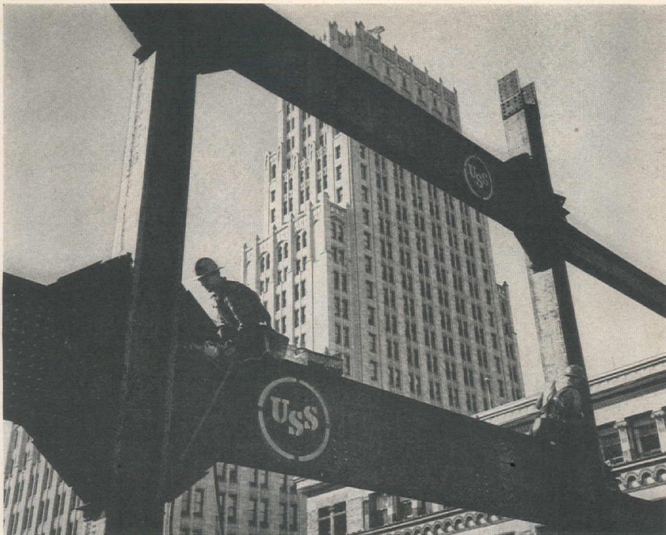
Special shock-resistant wind-braced girders—weighing 3\frac{1}{2} tons each—are being riveted into the new building of the Standard Oil Company of California now going up in San Francisco. Shaped from U·S·S steel, they will give the 22-story frame added toughness and strength.
