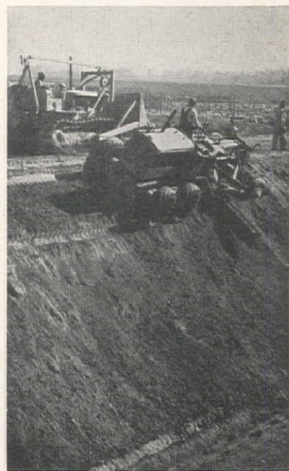
GRADING the 1½:1 channel banks looked like a profit-eating job until the idea of suspending a motor grader on the slope by steel cable from a dozer on the bank was devised.
