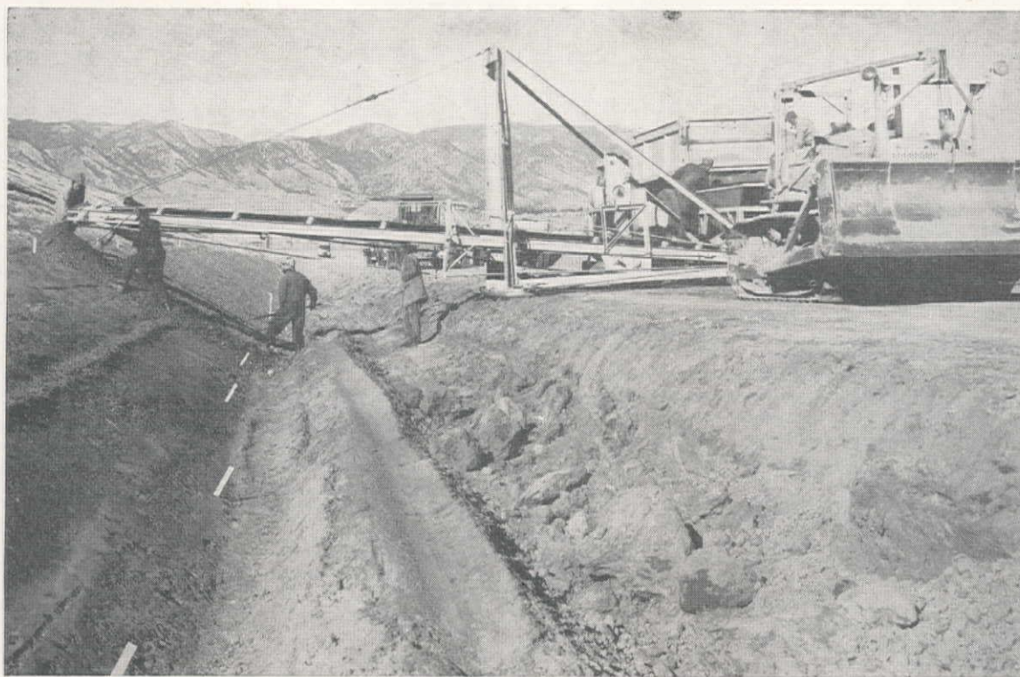
FILTER MATERIAL is being placed on the floodway's side slopes by a unique machine designed expressly for the job.
