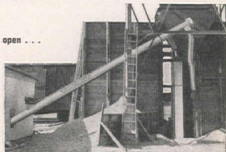
MODEL "Q" HI-SPEED Screw Conveyor
