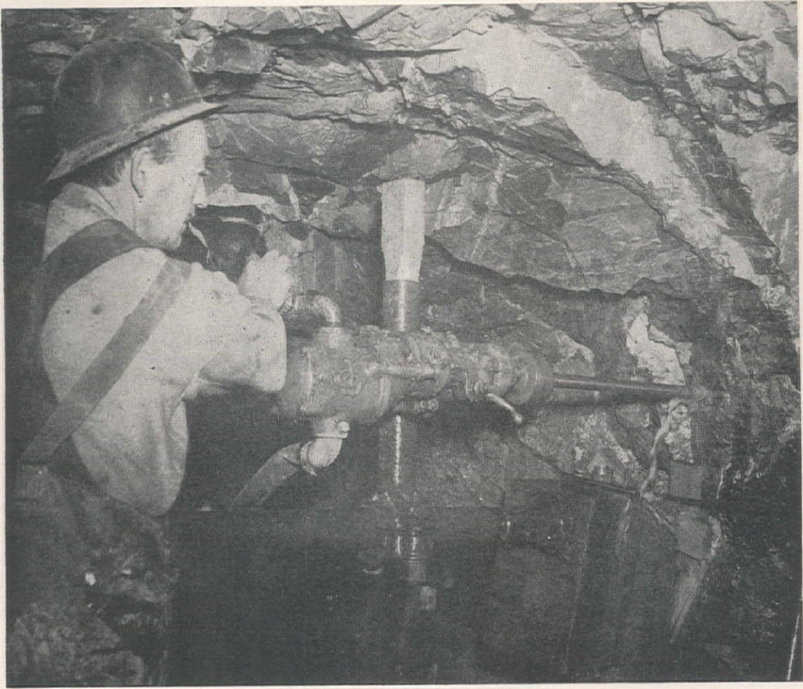
FROM A "SLOT" excavated beyond full tunnel diameter, a diamond drill bites a hole 60 ft. deep parallel to tunnel centerline.
