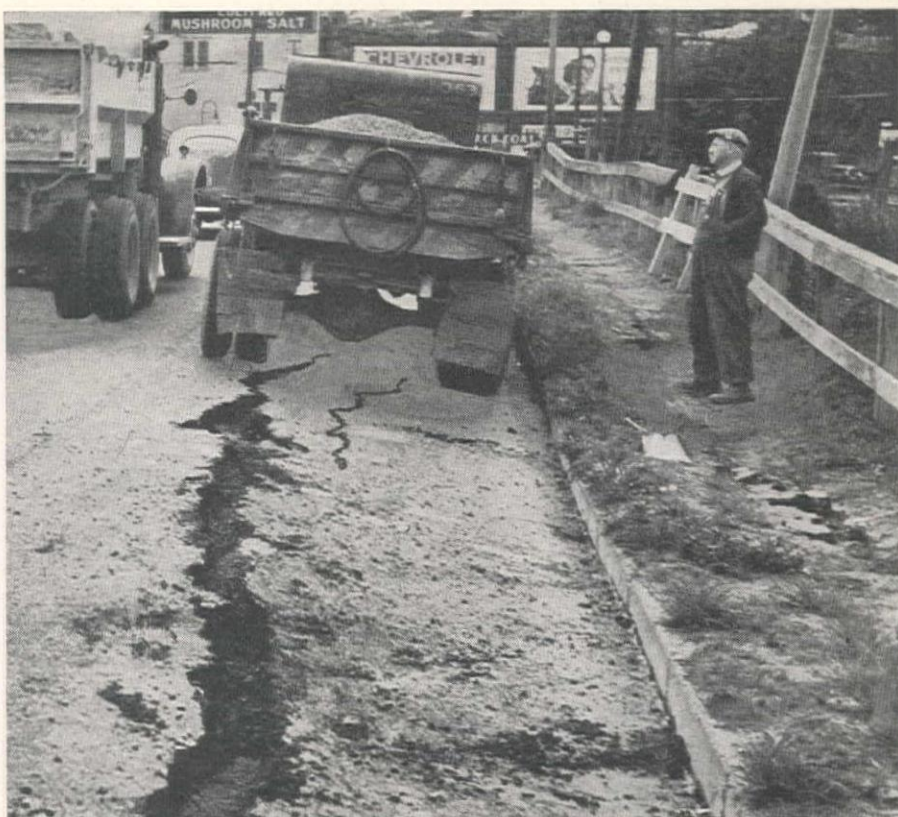
PAVEMENT FAILURE on a fill along Spokane St. approach to West Seattle, was followed two days later by failure of a water main beneath the pavement, which sent water gushing 100 ft. into the air and washed out a considerable portion of road.
