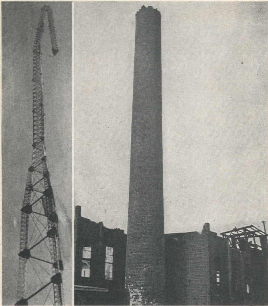
HIGH DAMAGE is illustrated by the 573-ft. steel tower of Radio Station KJR in Seattle, left, and the stack of an abandoned mill building on the tideflats near Tacoma. Despite the odd twist to the top 40 ft. of the radio tower, the station stayed on the air.
