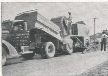
Showing aggregate being dumped directly from truck into front hopper of the Moto-Paver.
