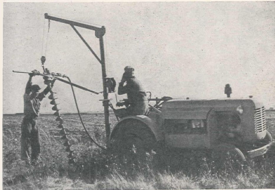
THE COMPRESSOR-AUGER team, above, operated by two men, has stepped up production of anchor holes from 8 to 42 in an 8-hr. working day.
