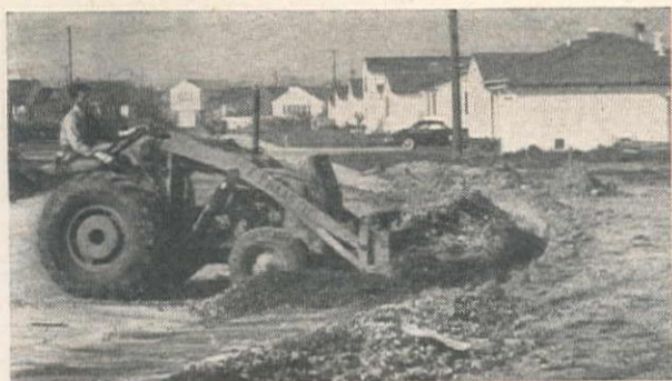
Model "DI" Case Tractor with hydraulically operated dozer, backfilling utility trenches in a Pacific Coast housing project.
