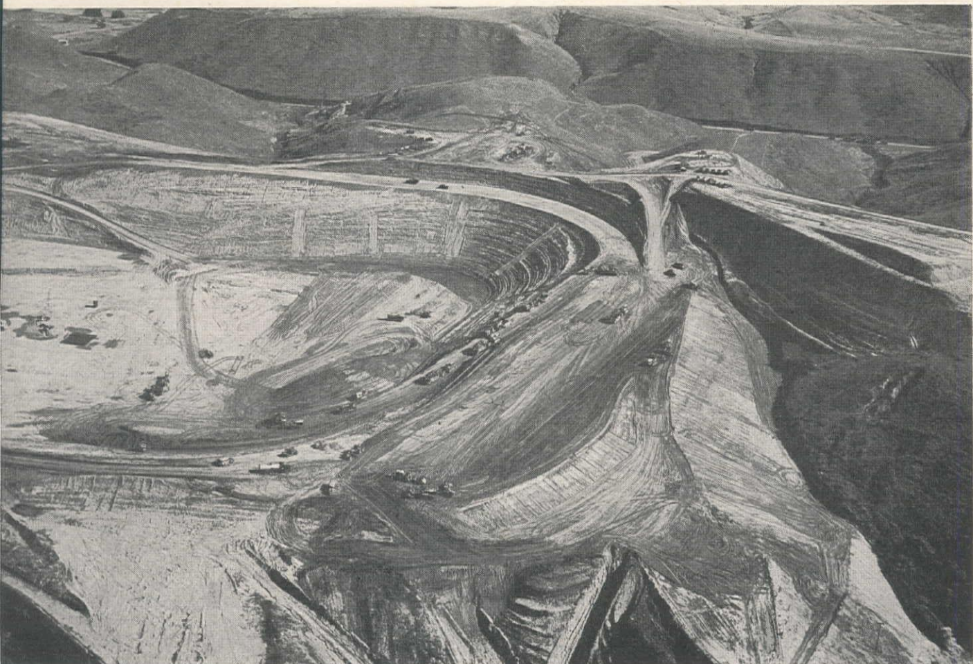
CRATER-LIKE reservoir is being built by reinforcing topography with Proctor-compacted earthfill.
