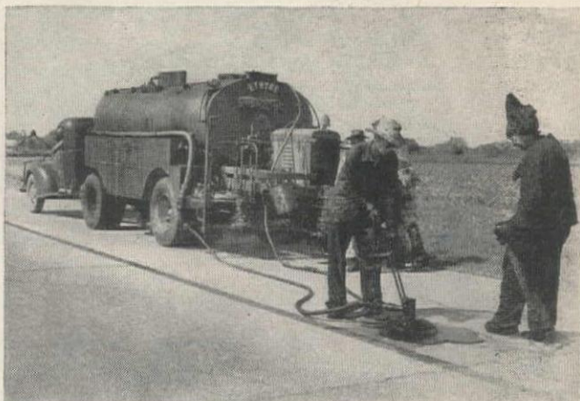
"Black-Topper" being used for underseal work to lift pavement by pumping Bituminous Material into weakened base.
