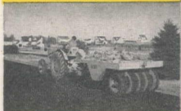
COMPACTING road surfacing material. A typical drawbar operation.
