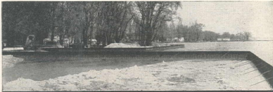
Filled earth inside a sea wall of ARMCO Steel Sheeting restores valuable lake frontage, provides additional lawn space and better docking facilities.
