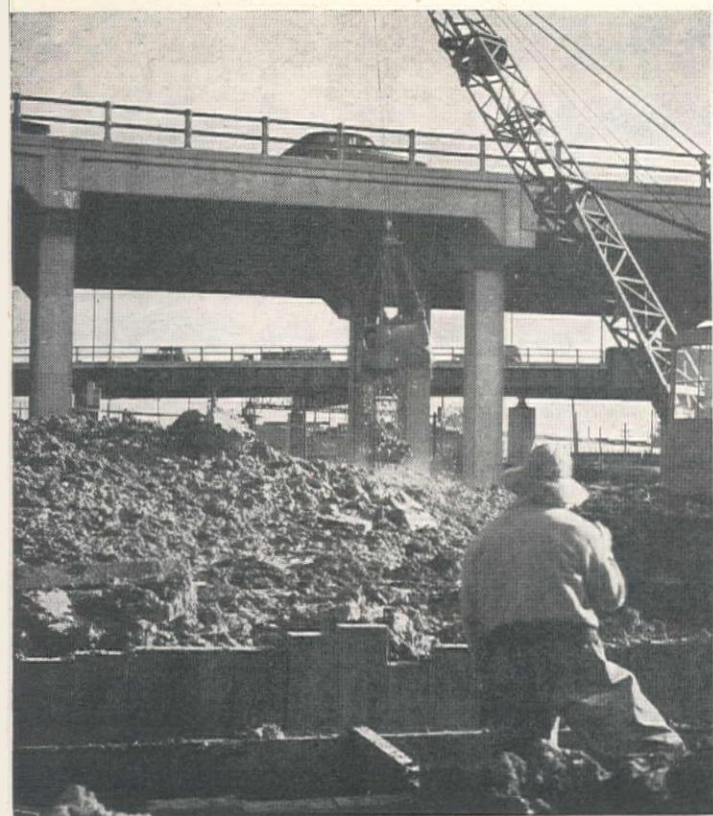
PLENTY OF MUD of the same type that plagued constructors of San Francisco's Bay Bridge is making excavation for the South Interceptor a tough job. At left, with spotter in foreground, a Lorain Moto-Crane equipped with a \frac{3}{4} -cu. yd. clamshell bucket, drops another load of mud alongside the sewer trench. Trench walls of timber, driven vertically and heavily shored, allowed just enough room for the clamshell bucket, right.
