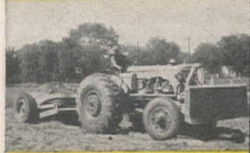
EARTH-MOVING with pull-behind scraper and front-end dozer.
