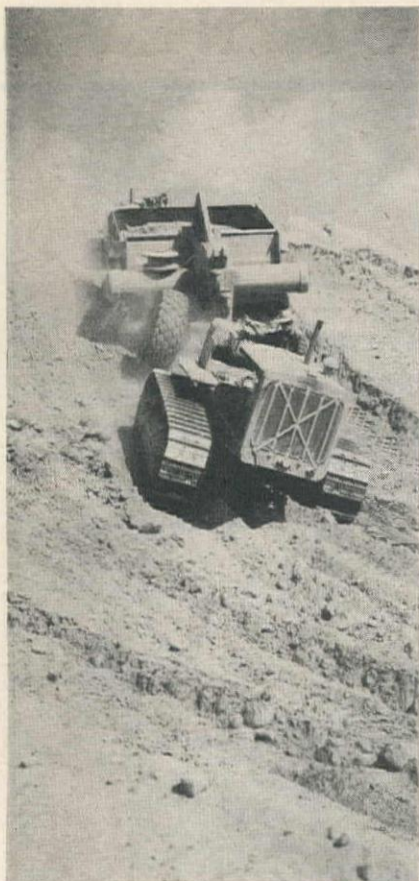
FILL MATERIAL was excavated from the cliff-side and carried to . . .
