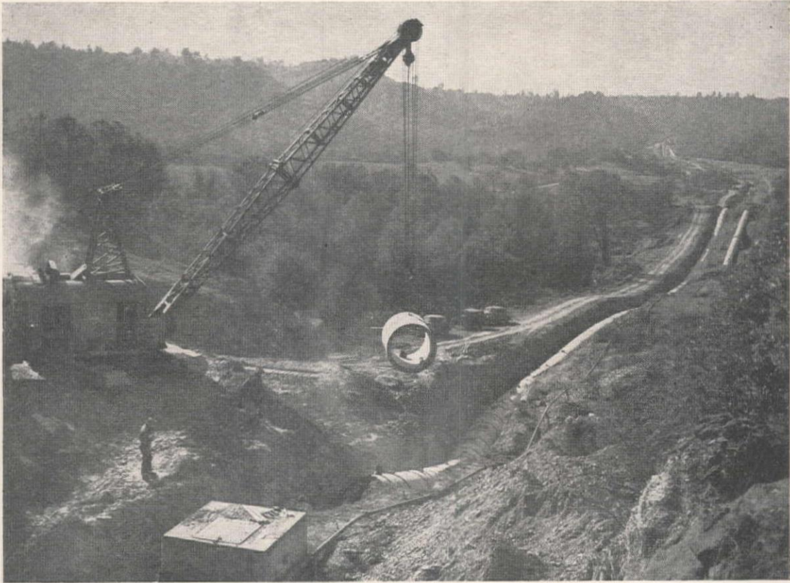
AMIDST FOG and Sierra Nevada foothills, another 24 ft. of the new aqueduct is lowered into place. Slopes were mild here.
