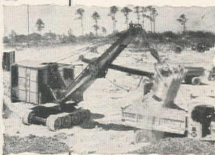
Almost a quarter of a century ago, this Lorain-75—equipped with a Twin Disc Clutch—worked for Highway Construction Company, Inc., on public-road jobs.
