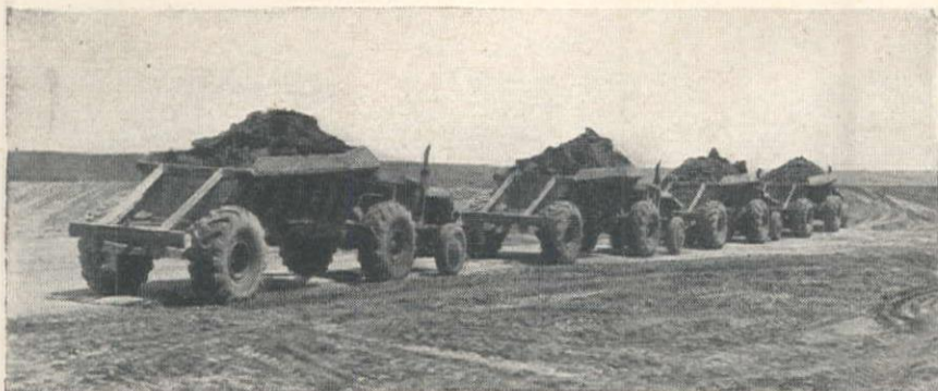
Garrison Builders, Inc., operators of this equipment, are working on the 14 million yard stage-one contract on the west side of the river. Shown is a convoy of four Euclid Bottom Dumps approaching the embankment fill area.
