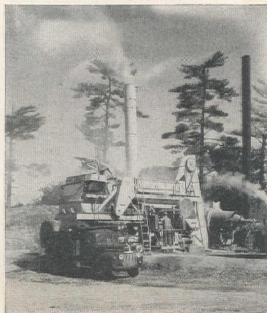
As much as 350 TONS per day of bituminous materials, thoroughly mixed, were produced by this Cedarapids Super-Portable Model "FA" in Ohio. {above}
