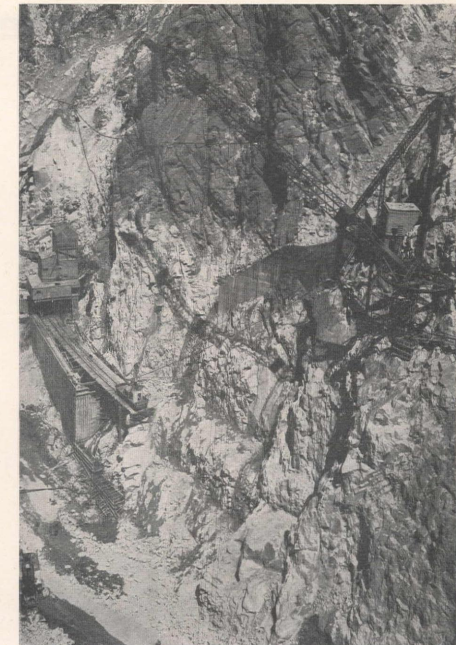
STIFF-LEG DERRICK is perched precariously above the powerhouse excavation. Note the completed deflector wall for protection against falling rock. Mixing plant, far left.
