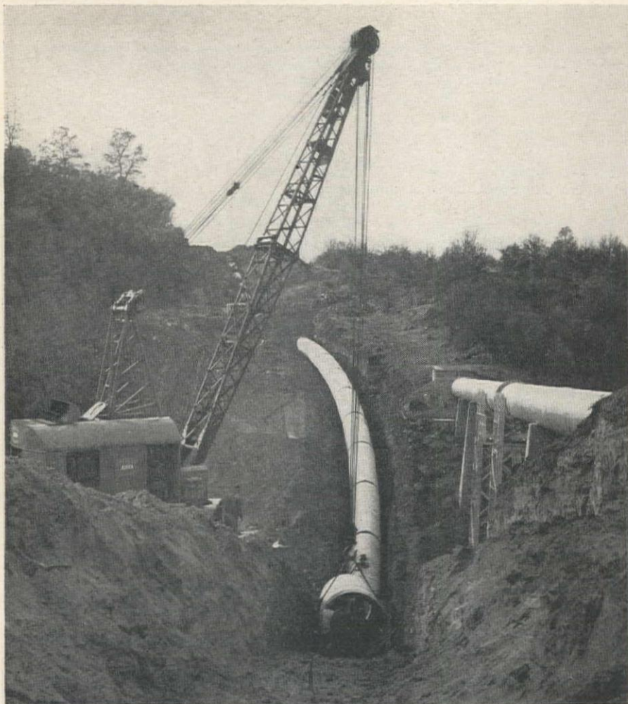
STEEL SHELL concrete pipe being placed to grade in the foothills of the Sierra-Nevada range. Steep slopes and wet weather were the toughest problems encountered in trenching and pipe-laying.
