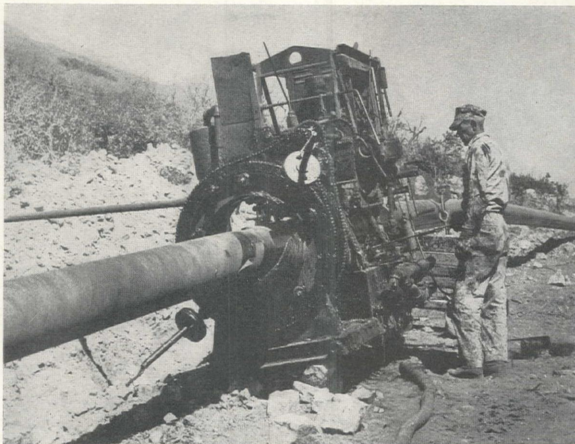
WRAPPING of asphalt, fibre-glass and felt was applied by machines, where level terrain allowed, as corrosion protection.
