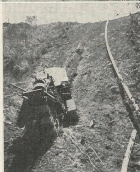
X-RAY MACHINE mounted on a jeep, left, examined welds while they were fresh. Blasting and a backhoe , upper right, excavated trench through hard rock, while a Buckeye ditcher dug trench elsewhere. On steep grades, the ditcher had some help, right.
