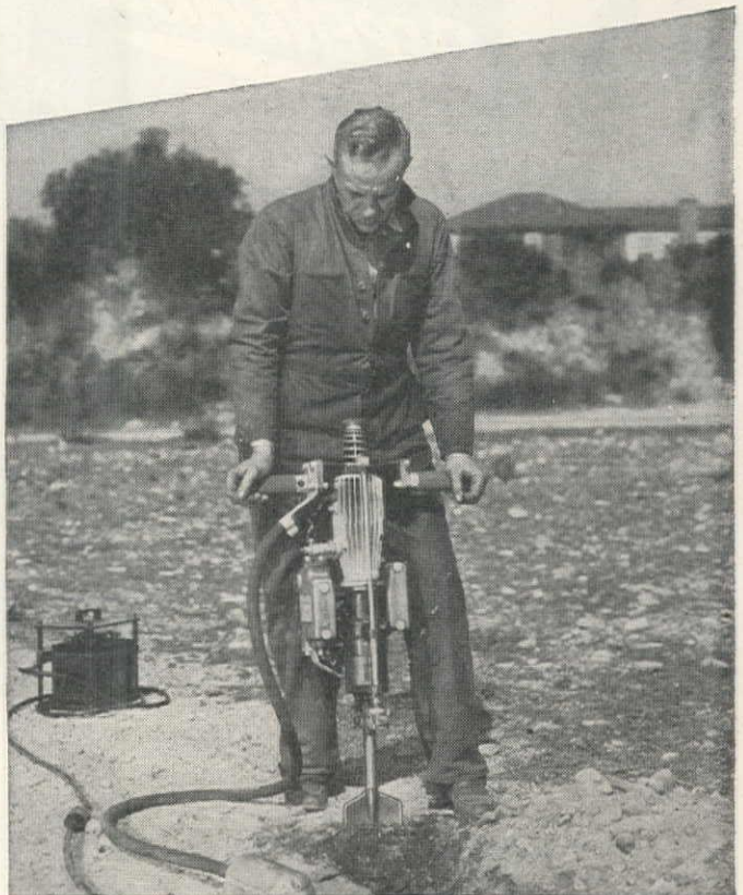
The Barco Model J-2, is ideal for hard ground or for digging in rock which can be broken out without blasting.
