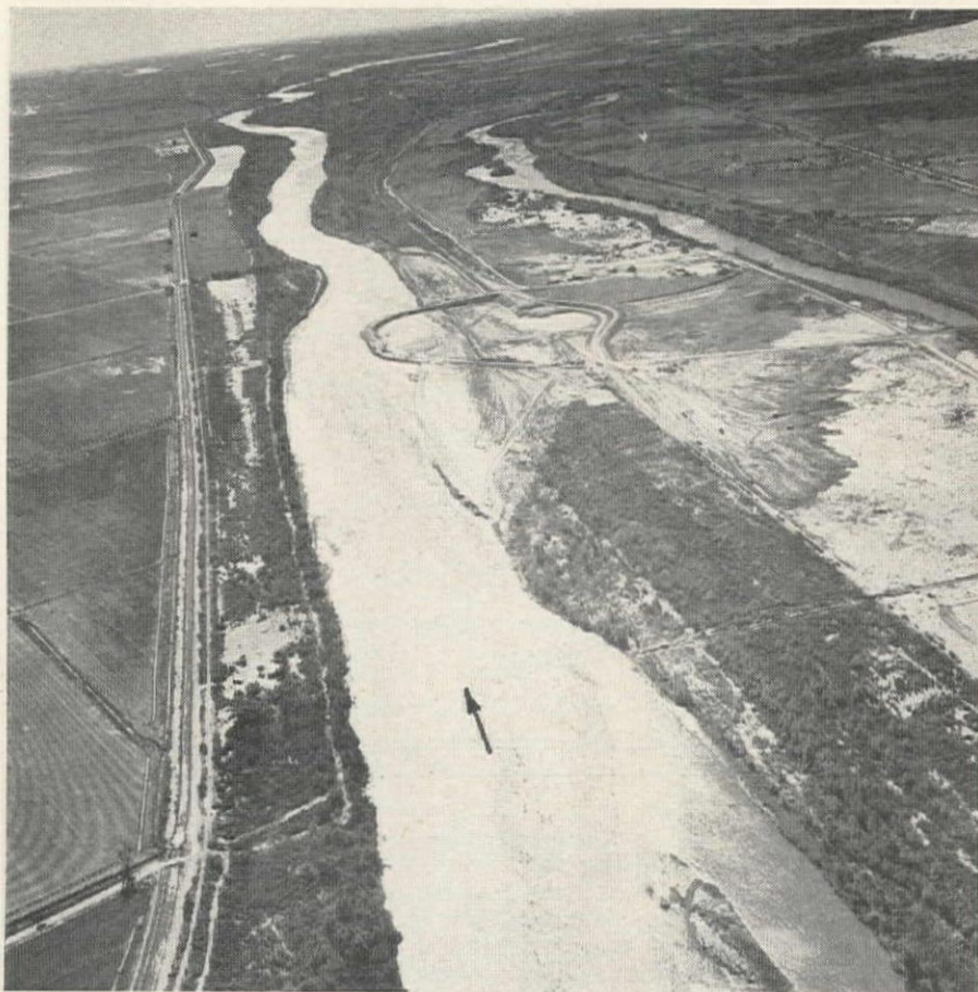
ARROW points downstream toward Morelos Dam site, where river cofferdam for the structure's west half and stripping operations on the right bank are completed.
