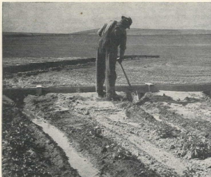
THE RIGHT WAY. Farmer at left has a well designed step flume. A canvass dam with gate is being used in irrigation ditch at right. The portable dam prevents too swift movement of water and keeps the level up.
