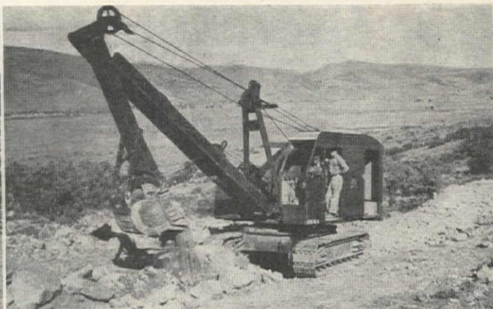
X-RAY MACHINE mounted on a jeep, left, examined welds while they were fresh. Blasting and a backhoe , upper right, excavated trench through hard rock, while a Buckeye ditcher dug trench elsewhere. On steep grades, the ditcher had some help, right.
