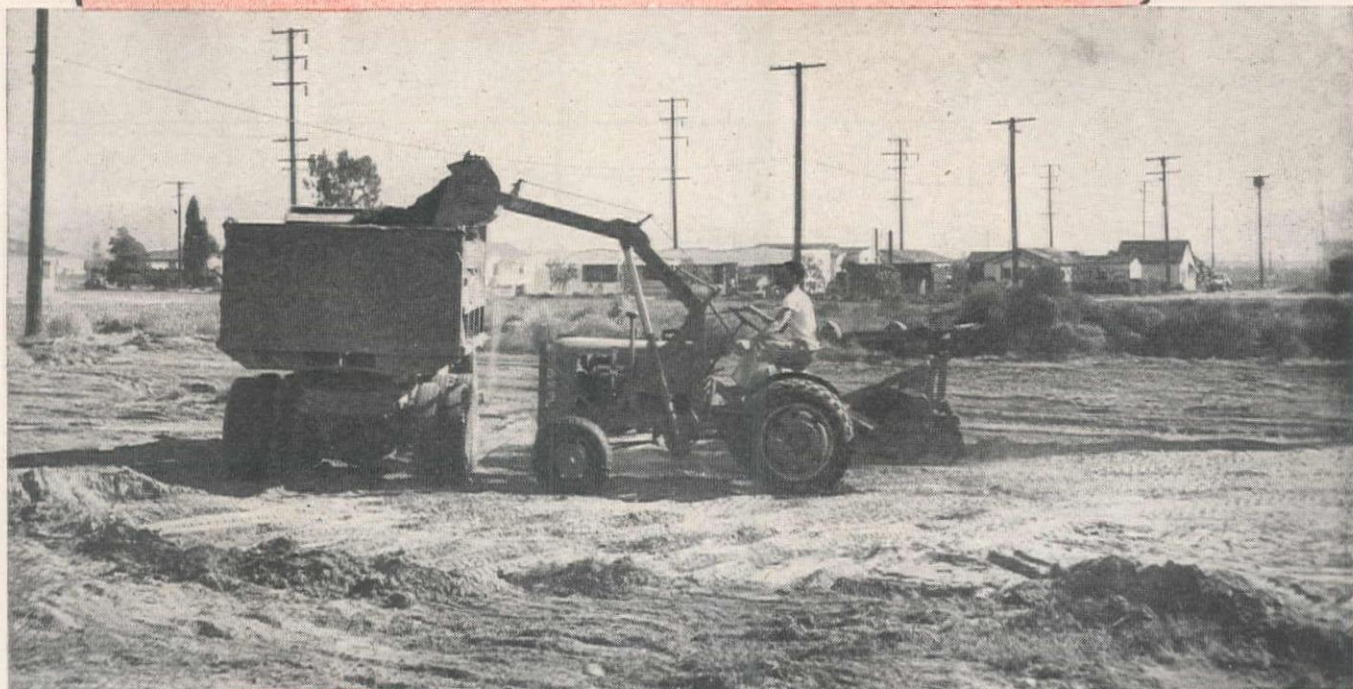
This "VAI" tractor is equipped with scarifier, scraper, and loader—a complete earth-working outfit.
