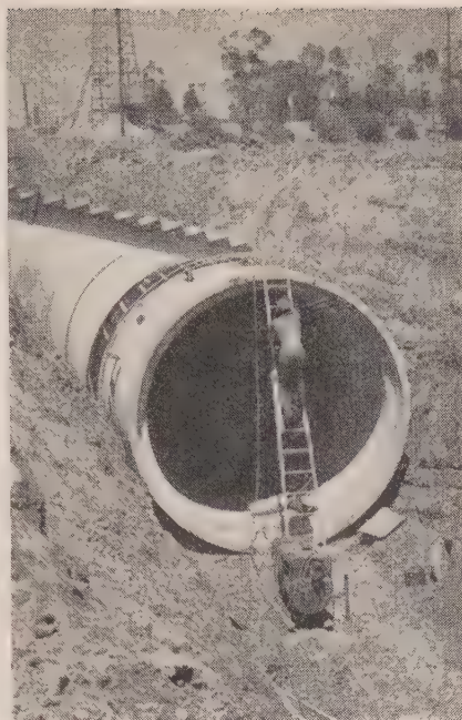
NEW FACILITIES for sewage disposal are a "must" in many of the West's municipalities. Los Angeles County's 12-ft. diameter outfall line is their answer.
