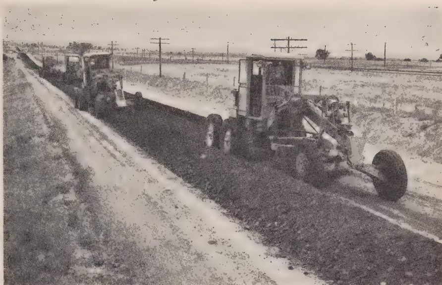
SEVERAL MOTOR GRADERS on one job typify the trend in Western road-building methods whereby increasing equipment investments are made to speed construction.
