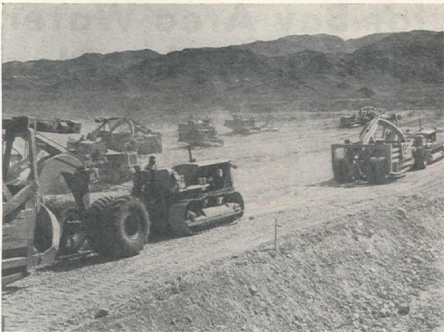
2,000,000 CU. YD. of natural rock and sand along the route was moved into place by dragline cranes, bulldozers and earthmovers for the roadbed fill and ballast.
