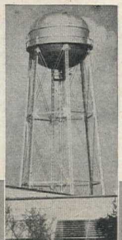
Double ellipsoidal 150,000-gal. tank on 100 ft. tower. Walt Disney Studios.
