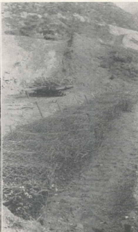
PART CIRCLE down drains, above, consisting of half sections of pipe laid on the surface, are adequate to carry run-off and will not fill up with debris. Improved machine at left below was used to crush brush into mats, center, which were placed on slopes above the roadbed as erosion protection, right. Old City Creek Road is visible at top of this view.
