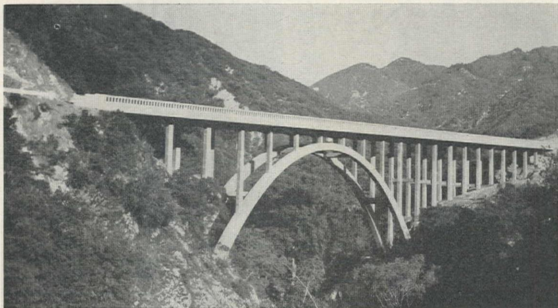
ARCH BRIDGE over City Creek, 430 ft. long and 130 ft. above the stream, blends well with the mountain locale.
