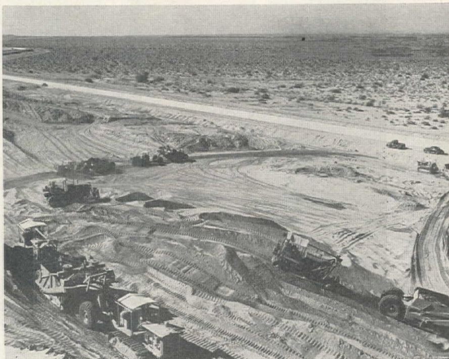
TYPICAL VIEW of dike construction shows the tractors and cable-controlled scrapers of 14 and 18-cu. yd. struck capacity loading in a through cut. In the desert, sand was deposited in 8-in. layers with only compaction being by the weight of heavy equipment rolling over it. Section of dike in background is parallel to main canal.
