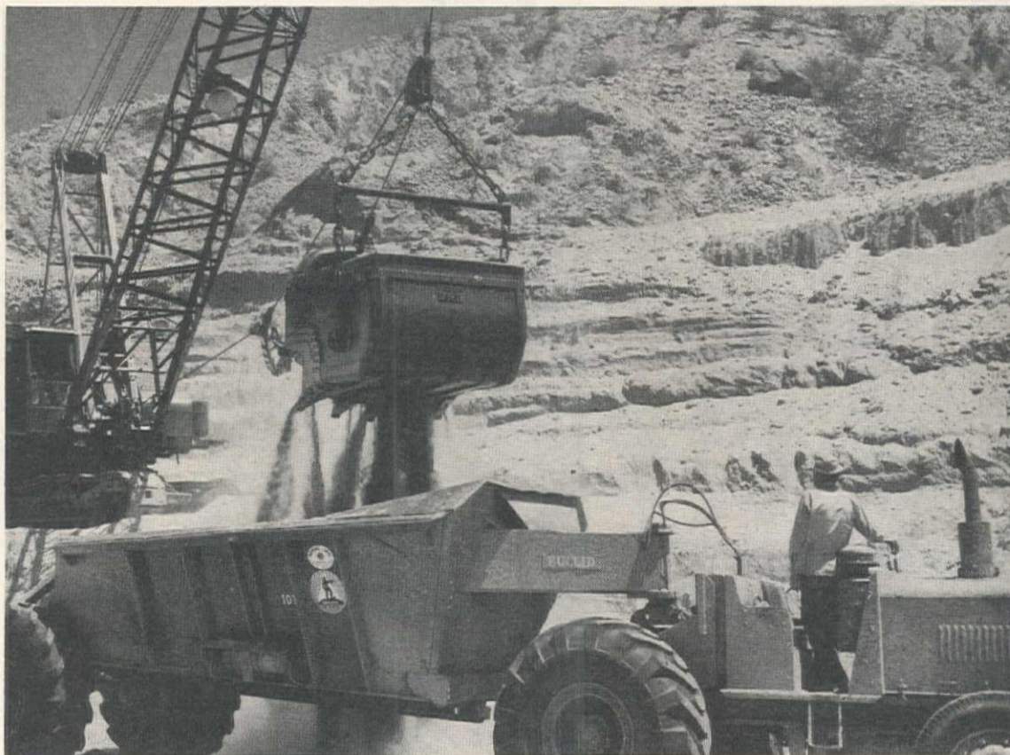
DRAGLINE with a 4-cu. yd. bucket loads a bottom dump Euclid wagon working along the base of the San Bernardino Mountains where cuts were up to 150 ft. The dragline-wagon team was used for completing the upper 10 ft. of the dike.
