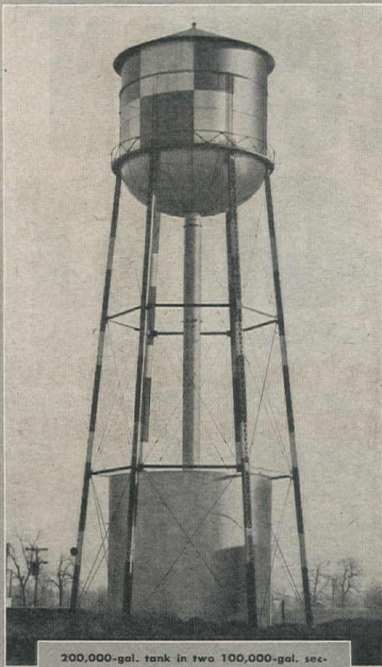
200,000-gal. tank in two 100,000-gal. sections, with 200,000-gal. standpipe at base, for fire protection at large assembly plant.
