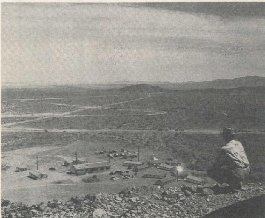
LAST PORTION of the railroad was designed in a giant "S" curve, visible from this vantage point above the mining camp. The curve was necessary to keep grade within the maximum limit. Deepest cut along the route, lower left, required blasting and excavating of 33,000 cu. yd. of solid rock. Right below, the 550-ft. long trestle over Salt Creek Wash is longest of eighteen such structures along the route.
