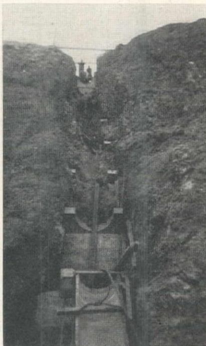
PART CIRCLE down drains, above, consisting of half sections of pipe laid on the surface, are adequate to carry run-off and will not fill up with debris. Improved machine at left below was used to crush brush into mats, center, which were placed on slopes above the roadbed as erosion protection, right. Old City Creek Road is visible at top of this view.
