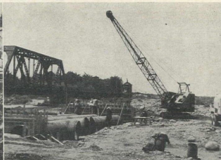
INITIAL construction of the stop-log structure, left, which is being provided to allow a railroad branch to cross the levee and will block flow under extreme flood conditions. Drainage structure providing outlet from Ventura under construction, right.
