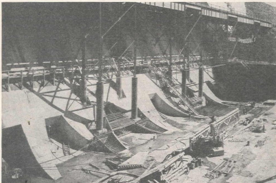
Cherokee Tennessee Valley Project. Spillway and Apron looking upstream from Training Wall.
