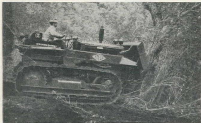
New ATECO Dozer clearing brush and trees on Rancho Del Carlos near Carmel, Calif. Note high lift of bowl.
