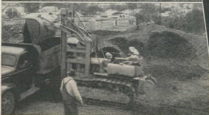
The D4 Traxcavator unit moves fast, loads fast to pile up yardage.
