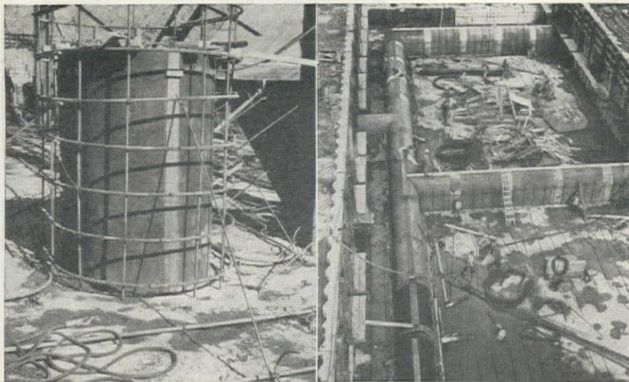
INSPECTION GALLERIES are installed throughout the spillway-outlet structure. Shown here are forms in place for pouring concrete around these galleries; a man-hole shaft form at left and part of the horizontal system forms at the right.
