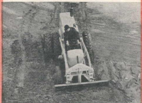
BULLDOZER Blade attachments, easily attached, increase Payloader usefulness.
