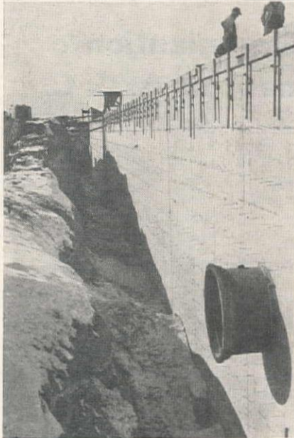
WALL AND ROOF construction, top, looking along the south side of Basin No. 1. The entire 24-ft. height of the walls was poured in one lift using a string of tremies and a bucket and crane. Bottom, completed south wall with forms removed. Inflow of water is from the south end.
