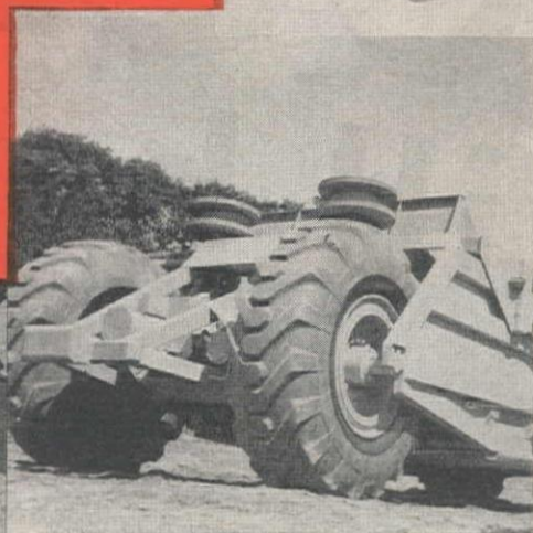
Big tires for more flotation and traction
