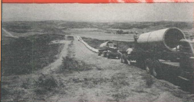
Route extends over hills and valleys. Pipe diameters range from 48" to 96", operating under heads up to 550'.
