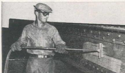
Scrubbing steel with a brush of flame removes scale, rust, and surface moisture prior to painting. This is flame-priming, a LINDE development.
