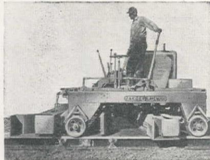
When finishing super-elevated curves, the angle of the rear screed causes it to carry the desired amount of material uphill to compact solidly against the higher form. Gradual adjustments of the screed angle can be made without stopping as the machine approaches and leaves super-elevated curves.
