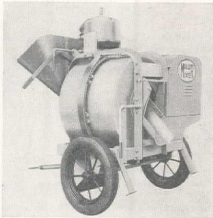
Features claimed: The machine is carefully balanced for easy handling and is built along the same lines as a big mixer. The drum and drumheads are made of heavy steel plate and revolve on wide solid rubber tires.
