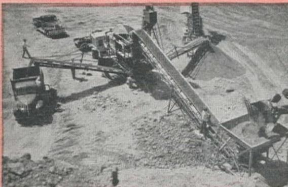
"81" Portable Crushing and Screening Plant
