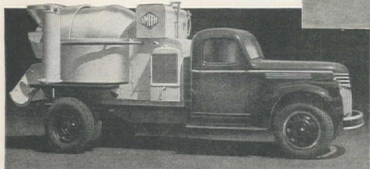
No. 2 Smith-Mobile with separate engine drive, mounted on Chevrolet Truck.
