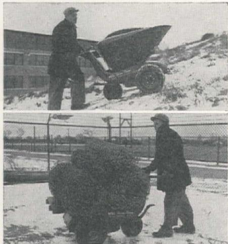
Features claimed: The device has a 1000-lb. capacity and is geared and powered to climb a 20 per cent grade with a full load. It is powered by a 3 h.p. air-cooled engine and operates for eight hours on three gallons of fuel. Transmission, clutch and gears are completely enclosed and no belts or chains are used to transmit power from the engine. The bucket has a capacity of 10 cu. ft. and the addition of sideboards raises the
