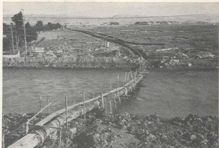
**THE PUMP LINE** from the dredge "Olympia" was 5 mi. long, most of it across Bay Farm Island. A booster pump on the dredge "Papoose" was used to facilitate movement of the material in the pipe. The "Papoose" dredged channel to reach pipe.
