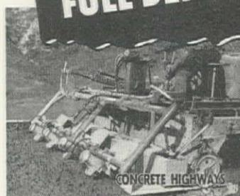
Write today for complete details on the VIBER method of full depth vibration
