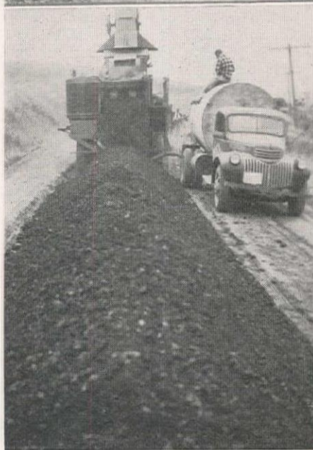
WINDROW MATERIAL to which cement has been previously added is picked up by loader and deposited in 8-ft. pugmill of the mixer, top. Loading augers distribute cement evenly through the soil. Mixed material, with slightly more than optimum water content, is discharged from the mixer into a windrow at side of trench, above left. Compaction by sheepsfoot roller, above right, with finger weeder following to remove equipment tracks. Personnel included, l. to r.: J. A. LIEDEBRAND, Portland Cement Assn., Chicago; R. E. TOBIN, Portland Cement Assn., Spokane; P. G. HAHN, Lehigh Portland Cement Co., Spokane; F. L. McATEE, McAtee & Heathe, Spokane.
