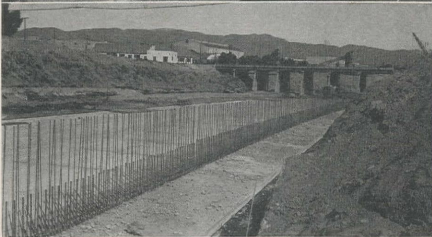
BARHAM BLVD. bridge was the only major crossing structure on the project. Its concrete piling was not disturbed, but a heavy concrete footing block was poured around the bottom of each bent, and diaphragm sections (first units poured in picture) are to be built to height of channel wall, top. Cantilever toe of wall section was poured before the wall, with dowels and reinforcing steel left protruding upward, bottom.
