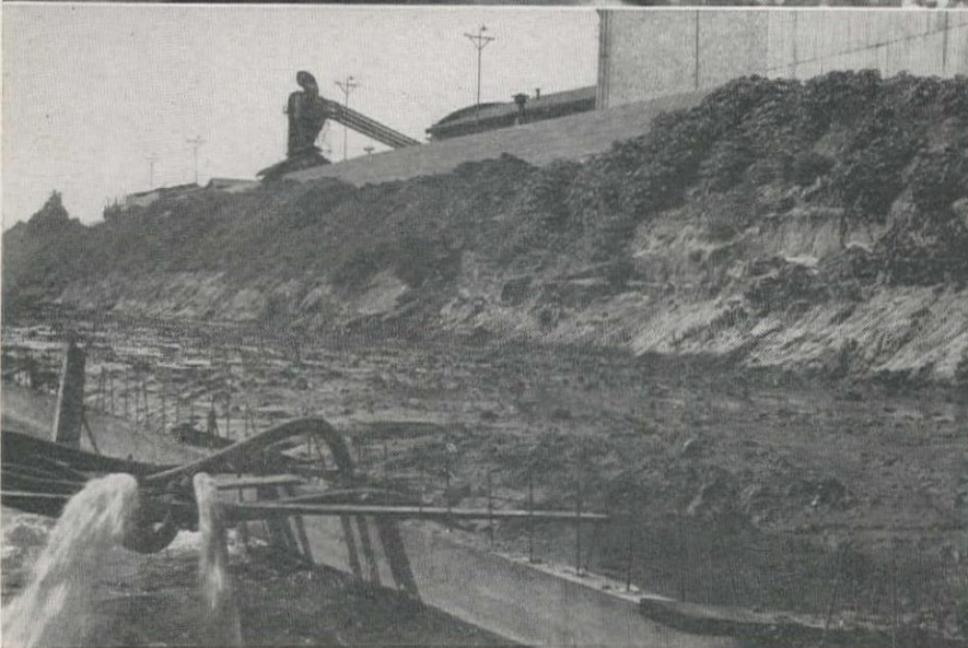
FLOWING SPRINGS were a major problem to the contractor on the L. A. River job, with about 13 cu. ft. per sec. of water bubbling up in the working area. First operation of the contractors was to construct a diversion ditch to carry normal summer flow of the river, top. Typical spring in the bottom of the river, partly bubbling, partly flowing, center. Water from spring area is removed from the spring area by pumps discharging into the low water channel, which was the first completed part of the job.
