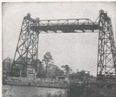
Fig. 2. Modern all-welded construction lift span bridge.
