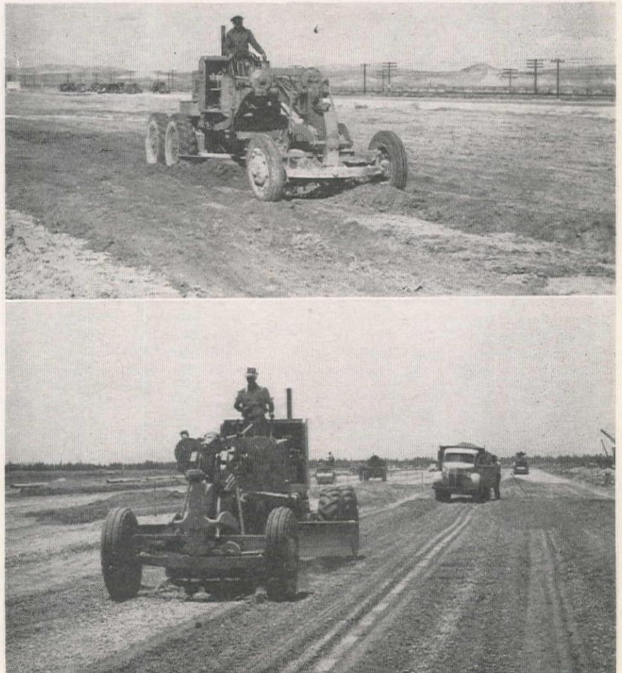
BASE CONSTRUCTION on an airport is illustrated by Lancaster, Calif., airfield, built during the war. Unsuitable clayey soil is removed, top, replaced with sand and gravel. Above this, bottom, was placed a base course of crushed rock, compacted by rolling.
