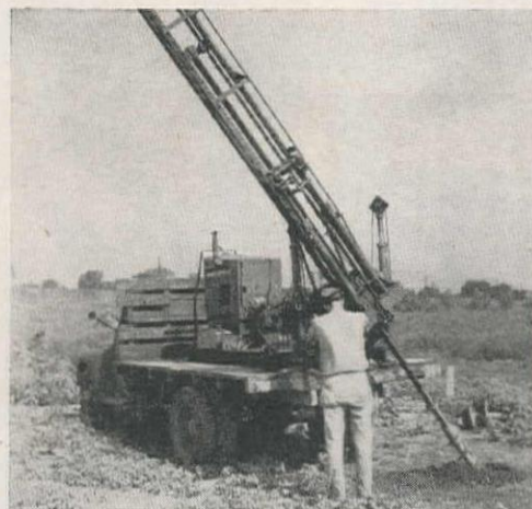
Model HBJ drills angle holes to 45° from vertical.
