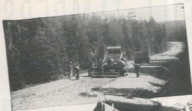
ABOVE—Laying a four-inch course of No. 1 rock with an Adnun. Rock passes 4-inch screen, retained on 2-inch... An extra, profitable job for any Adnun!
