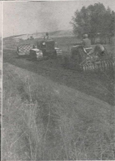
WINDROW MATERIAL to which cement has been previously added is picked up by loader and deposited in 8-ft. pugmill of the mixer, top. Loading augers distribute cement evenly through the soil. Mixed material, with slightly more than optimum water content, is discharged from the mixer into a windrow at side of trench, above left. Compaction by sheepsfoot roller, above right, with finger weeder following to remove equipment tracks. Personnel included, l. to r.: J. A. LIEDEBRAND, Portland Cement Assn., Chicago; R. E. TOBIN, Portland Cement Assn., Spokane; P. G. HAHN, Lehigh Portland Cement Co., Spokane; F. L. McATEE, McAtee & Heathe, Spokane.
