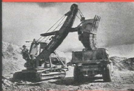
BADGER SHOVEL—Convertible to crane, dragline, piledriver, trench hoe, and skimmer. \frac{3}{4} -swing design has many operating advantages.
