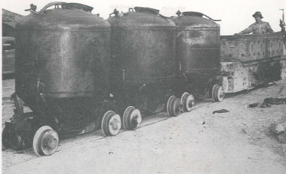
KEMPER PNEUMATIC concrete placers, manufactured by M. F. Kemper Construction Co., of Los Angeles, employ new and simplified principles of pneumatic concrete handling to make tunnel lining, particularly holes of small diameter, easy and fast. At Grossmont Tunnel, being lined by the company for City of San Diego, trains of three 1½-cu. yd. placers are used.
