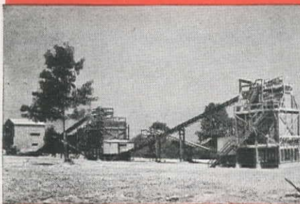
STATIONARY CRUSHING AND SCREENING PLANTS—Each, like this "agstone" and road rock plant, engineered especially for the job it has to do.
