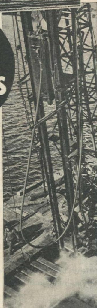
McKiernan-Terry Double-Acting Hammer driving timber piles to strengthen a pier at the U. S. Navy Submarine Base, New London, Conn.
