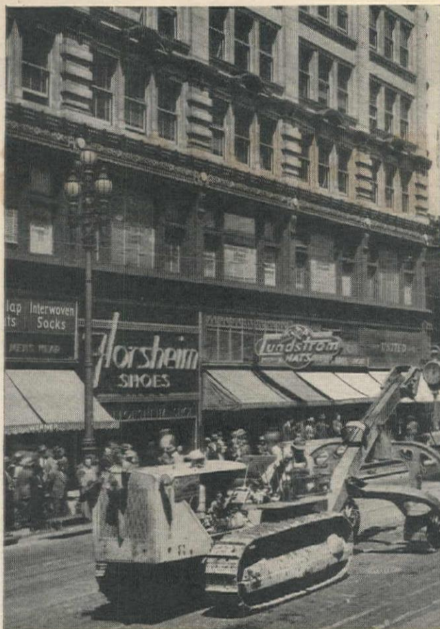
A "Caterpillar" Diesel D8 with Hyster arch makes an ideal tool for rail removal, lifting one 62-foot section at a time.
