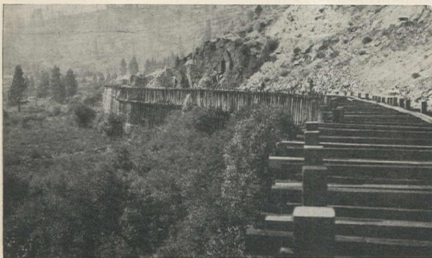
OLD WOOD box flume 10 ft. wide and 8 ft. high conveying Truckee River water to the Farad power plant, one of five plants in the system. Leaks in the flume are frequent.
