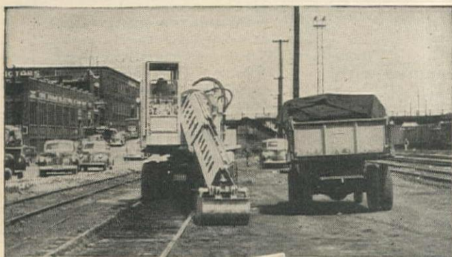
Cleaning cinders between and outside track is usually a manual job to avoid damage to ties, rods, tie plates, etc. The amazing dexterity and precision of Gradall now permit this job to be done by machine.
