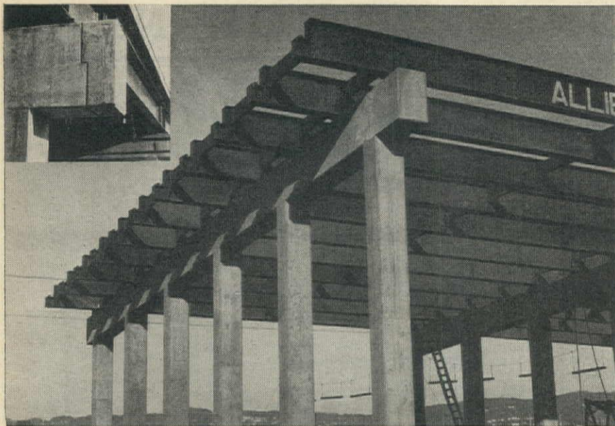
SYSTEM OF cantilevered 36-in. I-beams to carry deck shown in position. Joints can be seen where shorter stringers will be suspended between alternate bents. Inset shows construction joints included at cap extremities as future widening provision.
