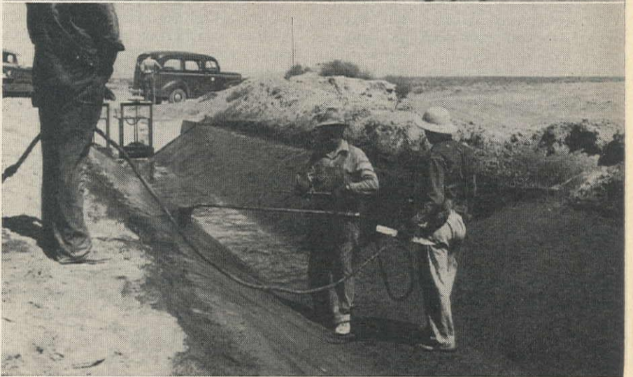
FINISHING sections of asphaltic-lined canal. Top, hand-placed areas adjacent to structures were sealed by handspray and squeegee; center, cleaning a section of lining preparatory to sealing with 50-60 penetration asphalt cement—air-blast was necessary to remove fine sand and dust in this area which had been badly scuffed during initial operation of paver; bottom, membrane-type lining (see picture on next page).
