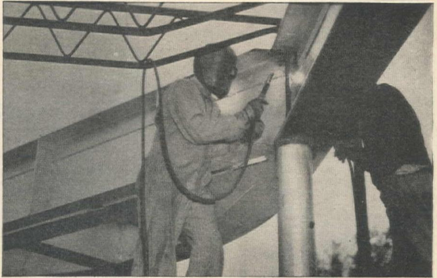
Fig. 2. Two welders weld heavy beams simultaneously to avoid distortion.
