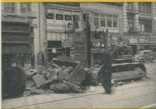
Loading trucks with broken concrete, a "Caterpillar" Diesel D7 and Traxcavator work fast without disturbing traffic.
