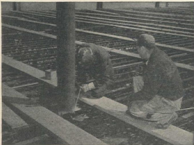
Fig. 1. Welding pipe column to first floor I beam. Column has a smaller pipe and concrete inside.
