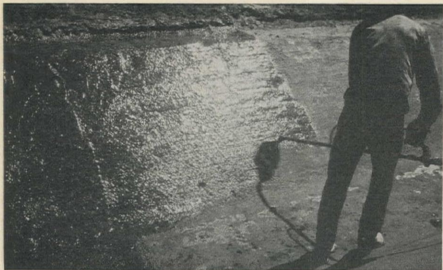
CONSTRUCTION of test section of prime-membrane type lining; diatomaceous earth is being sprayed at 425 deg. F. on surface primed with Diesel fuel and RC-O.
