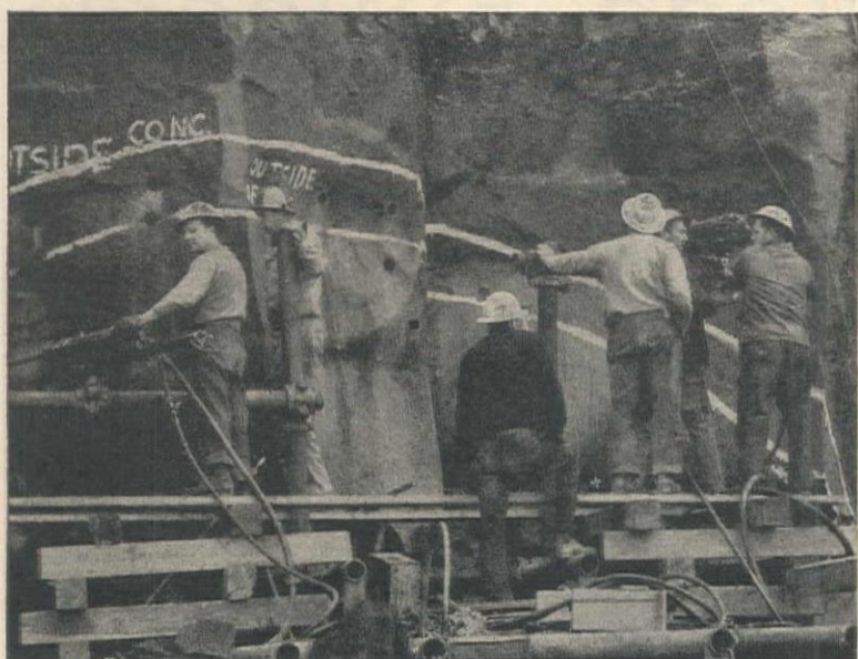
Jumbo set-up with drifters using Bethlehem Hollow Drill Steel in the first round of drilling on the 2-mile Bacon tunnel. Contractor: T. E. Connolly, Inc., San Francisco.
