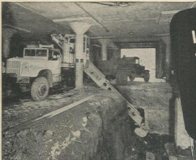
Low head room and numerous pillars and bases only 20 feet apart made excavating for a sub-basement in a complete building a tricky job. Gradall fitted perfectly on this job, eliminated need for costly manual labor.
