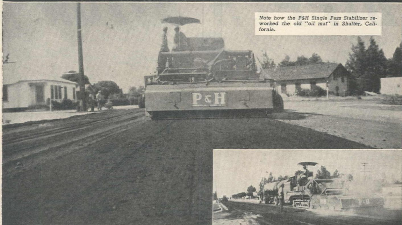
Here the processing went to a depth of 3\frac{1}{2} inches at a rate of 1000 sq. yds. per hr. Many days the rate increased to 1200 sq. yds. per hr.
