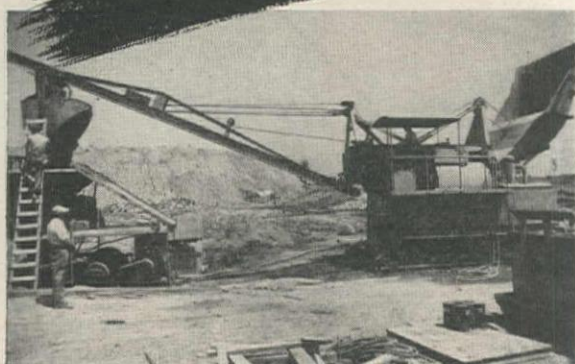
MultiFoote 34-E Duo Mix (Dual Drum) Paver with elevating boom loading to a pumpcrete.
