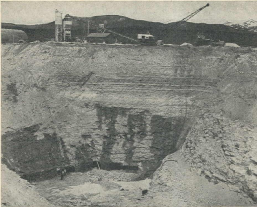
EXCAVATION for Granby Pump Plant is in sandstone on the left bank of Soda Creek, about 115 ft. deep and 700 ft. in from the stream. When building and intake structures are built in this excavation, they will be backfilled with excavated material which has been stockpiled for the purpose. Contractor's yard is on top of hill.
