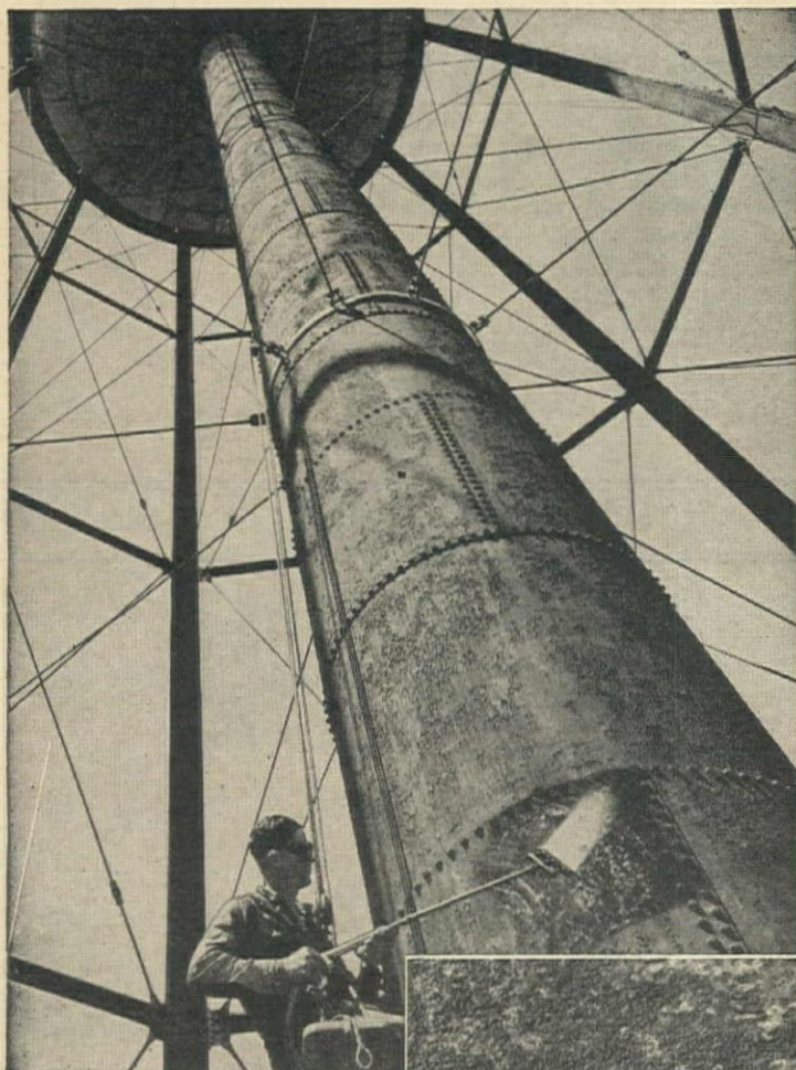
Start of flame-cleaning operation on water tower structure
