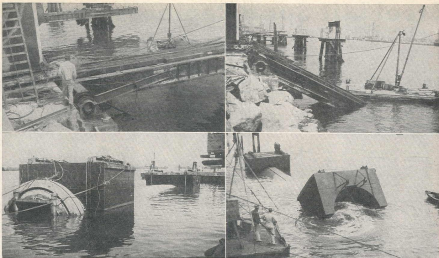
LAUNCHING RAMP for 100-ft. pipe is in raised position with pipe ready to be moved onto ramp, upper left, and in lowered position, right. Lower left, the pipe launched with flotation tanks in place ready for the tow, and right, tanks, being removed at the job site. Pipes were launched at the casting yard in the Long Beach harbor area since gradually sloping beach and heavy surf conditions made the job site unsuitable.
