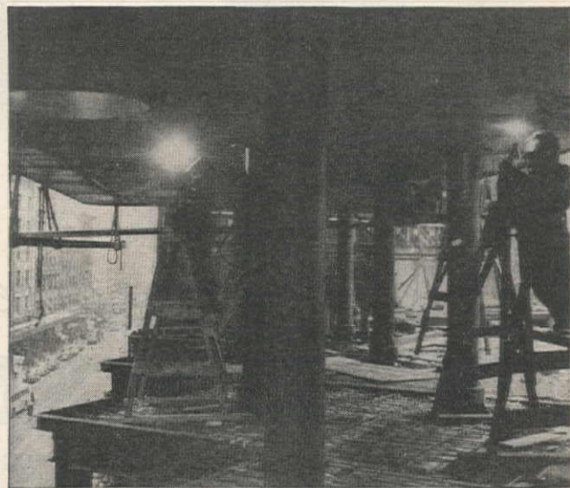
Fig. 5. Finish-welding underside of the canopy.
