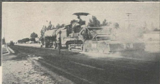
Here the processing went to a depth of 3\frac{1}{2} inches at a rate of 1000 sq. yds. per hr. Many days the rate increased to 1200 sq. yds. per hr.
