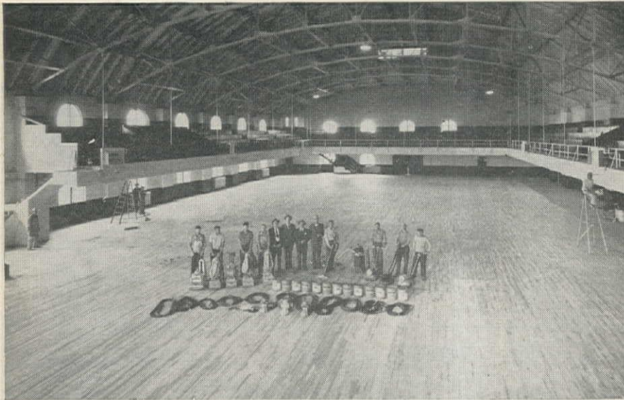
EXTENT OF RECONDITIONING required is indicated by this view of the drill hall after completion. The new flooring patch in left foreground is 91 ft. wide by 70 ft. long. The flooring crew with equipment shown worked on a 24-hr. schedule to complete the work within the time limit. Interior was sand-blasted before painting.
