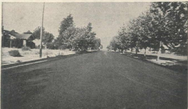
Completed street after shaping and rolling. The only equipment used was the P&H Stabilizer, tank truck, roller and grader.
