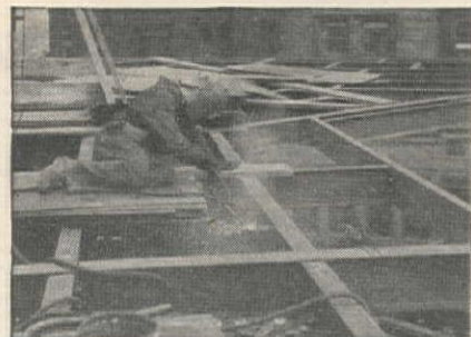
Fig. 4. Welding soffit plates of the canopy.
