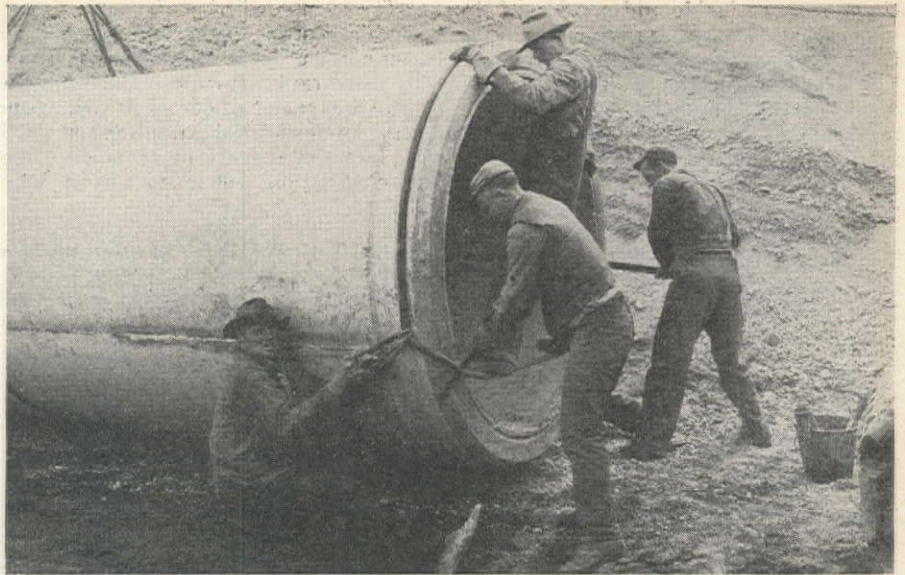
PLACING RUBBER gasket on spigot end of a 20-ft. section of 69-in. precast concrete pipe prior to placing in the siphon. The gaskets are prefabricated to exact size and must be stretched to fit into their proper place by strenuous manual labor.
