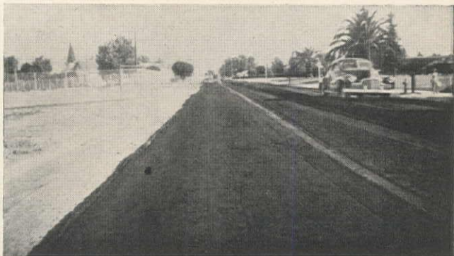
Note the thorough pulverization of the old "oil mat"—the accurate application of asphalt and complete mixing. Traffic does not have to be re-routed with this new method.
