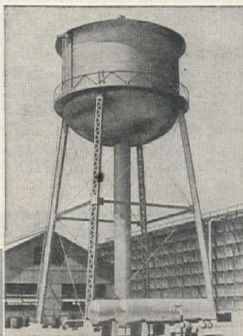
Hemi-ellipsoidal bottom 100,000-gal. tank on 44 ft. tower, El Paso Natural Gas Co.
