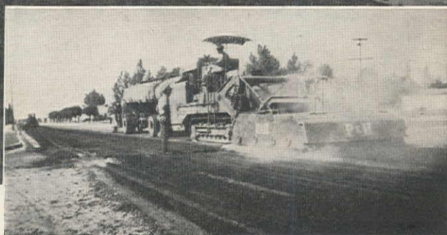
Here the processing went to a depth of 3½ inches at a rate of 1000 sq. yds. per hr. Many days the rate increased to 1200 sq. yds. per hr.
