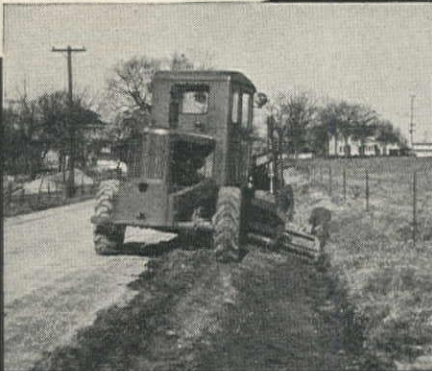
DITCH CLEANING. Rear steer places the rear truck up on the road where there is good footing.
