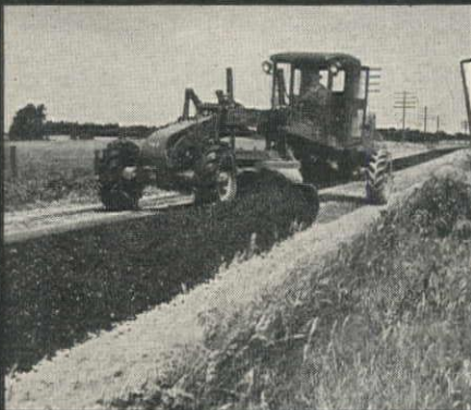
BLACK-TOP RESURFACING. All wheels miss the windrow.
