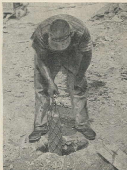
▲ Shooter preparing to load 5"x24" cartridge of "Gelex" into well drill hole.
