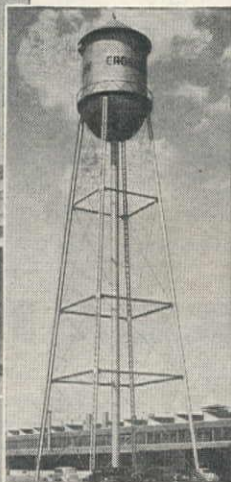
Hemispherical bottom 100,000-gal. tank on 116 ft. tower, Crosley Radio Corporation.
