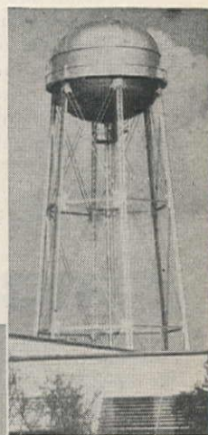
Double ellipsoidal 150,000-gal. tank on 100 ft. tower, Walt Disney Studios.
