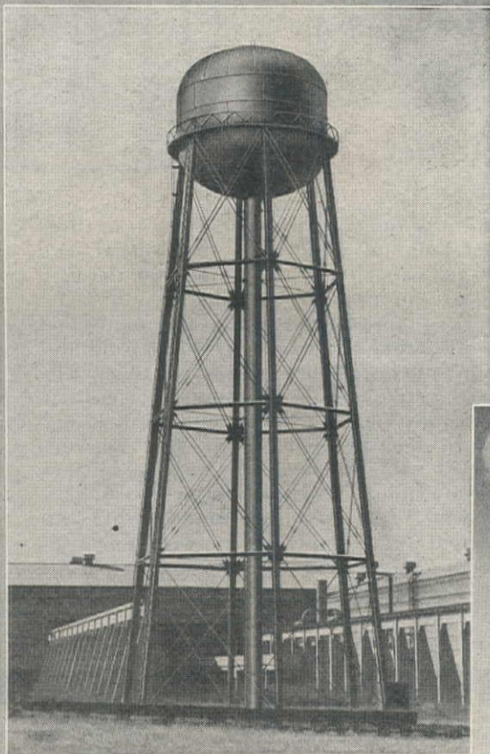
200,000-gal. Double Ellipsoidal Tank on 125 ft. tower, Columbia Steel Co.
