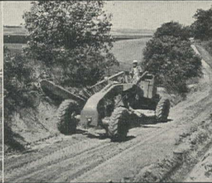
ROAD WIDENING. The High-Lift Blade handles any degree of slope from flat to vertical.
