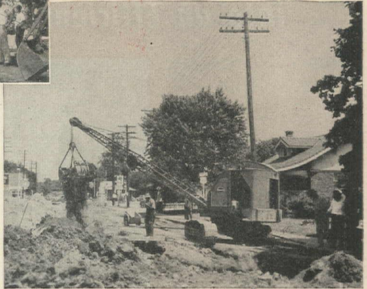
As a CRANE . . . setting concrete tile on a storm sewer project. Note clamshell bucket set aside for this operation.
