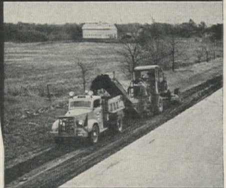
LOADER ATTACHMENT. Removing excess material from ditch and shoulder.
