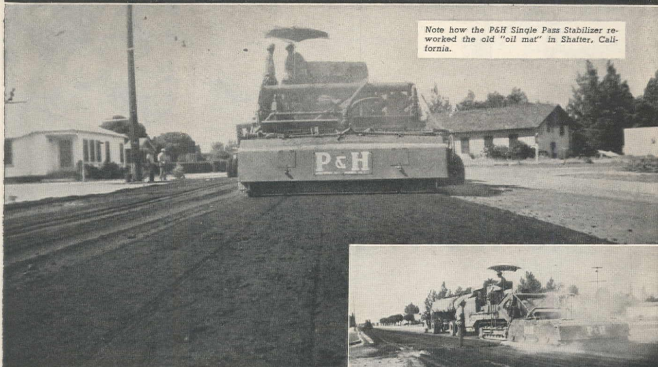
Here the processing went to a depth of 3½ inches at a rate of 1000 sq. yds. per hr. Many days the rate increased to 1200 sq. yds. per hr.
