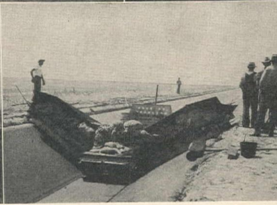
SLIP FORM used in placing the 3-in. concrete lining in the lateral system is shown, upper left. Method and machine for trimming laterals for the lining are shown in picture at upper right, while picture middle left shows gunite equipment for placing of 1½-in. thick pneumatically applied mortar lining on system. Placing and finishing of the mortar lining on lateral is shown in picture at middle right. Below, left, shows a general view of asphaltic lining operations. Hot mix is placed in paver by a ¾-cu. yd. clamshell. Paver is shown laying and finishing lining (middle) and being lifted over canal structure (right).
