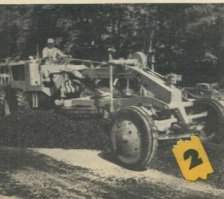
1 A "Caterpillar" Diesel No. 12 Motor Grader shapes ditches on a county road in Crawford County, Mich. The big tires give excellent control in sandy soil.
