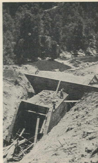
CONCRETE CULVERT through which West Point penstock will pass underneath a new state highway. Intricate design was required, as the culvert is both on a skew and steep grade of penstock.
