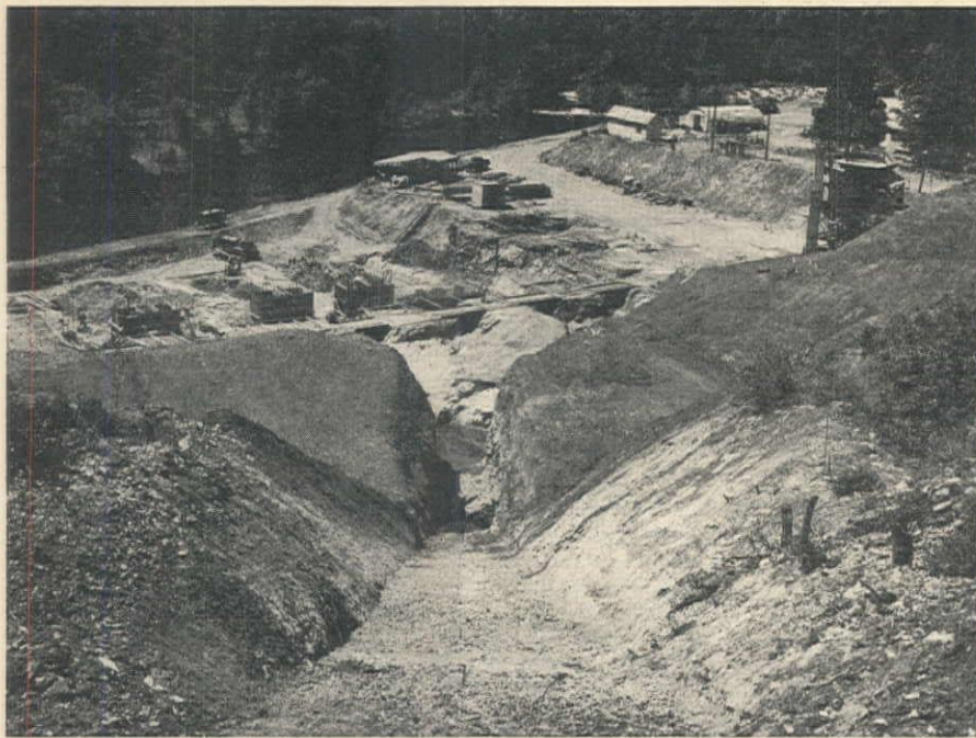
EXCAVATION for penstock and powerhouse at Electra power plant site. Some of the excavation for the interesting forked penstock installation can be seen through the deep cut. Powerhouse switching yard will be located on the level bank at center.
