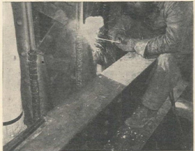
Fig. 3. Brackets from 21-inch I-beam are welded to existing column.
