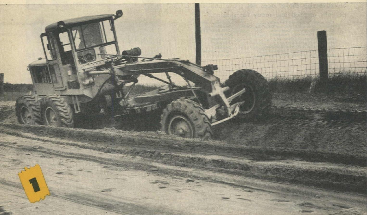
1 A "Caterpillar" Diesel No. 12 Motor Grader shapes ditches on a county road in Crawford County, Mich. The big tires give excellent control in sandy soil.
