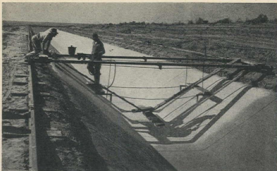
CURING COMPOUND is being applied to the newly placed 3-in. concrete lining on the Pasco Pump Lateral system. The rails along the berms are used for trimming machine, concrete placing and finishing machine and compound sprayer.
