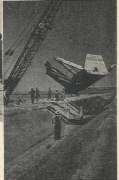
SLIP FORM used in placing the 3-in. concrete lining in the lateral system is shown, upper left. Method and machine for trimming laterals for the lining are shown in picture at upper right, while picture middle left shows gunite equipment for placing of 1½-in. thick pneumatically applied mortar lining on system. Placing and finishing of the mortar lining on lateral is shown in picture at middle right. Below, left, shows a general view of asphaltic lining operations. Hot mix is placed in paver by a ¾-cu. yd. clamshell. Paver is shown laying and finishing lining (middle) and being lifted over canal structure (right).
