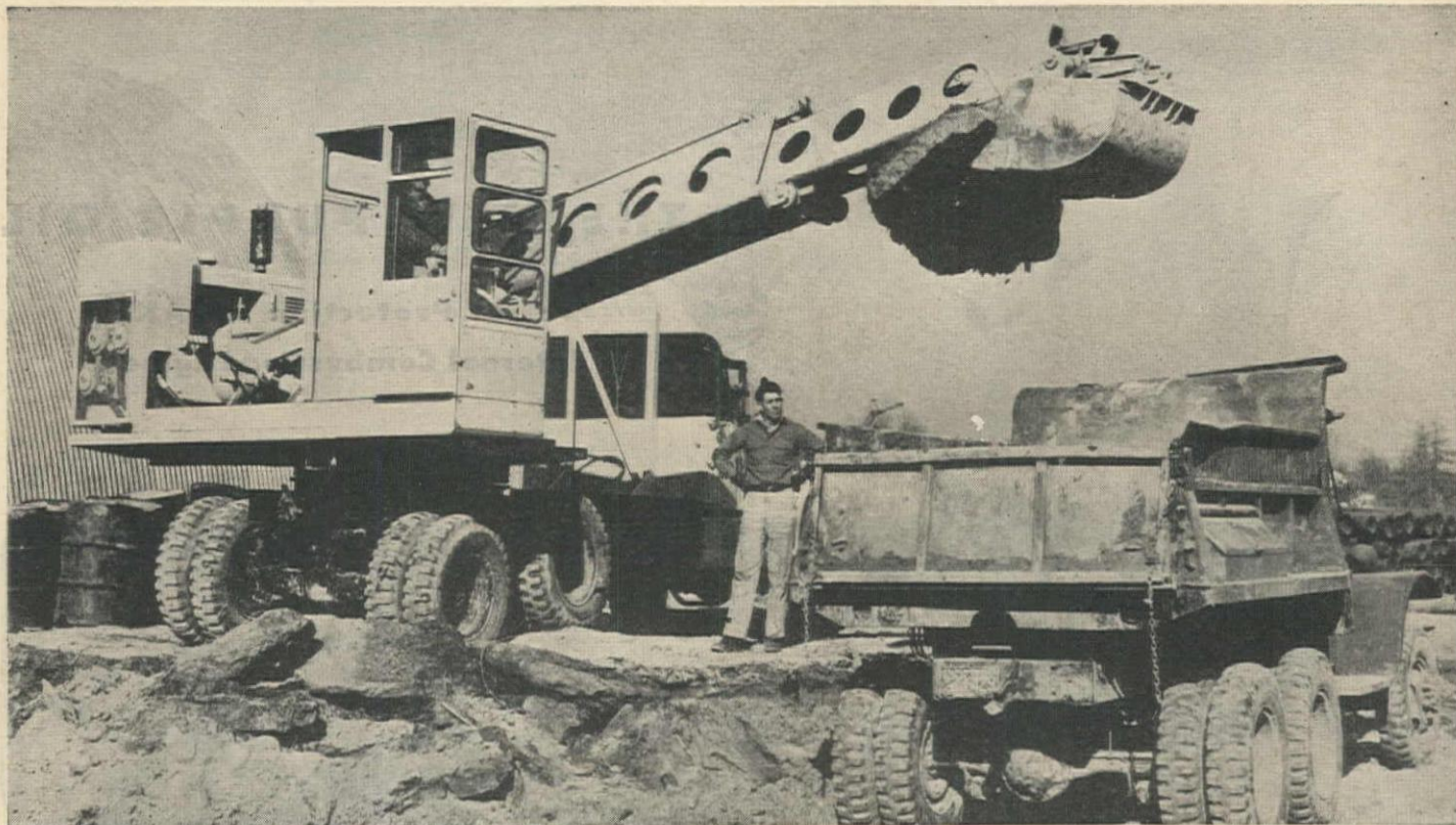
Gradall's powerful telescoping boom loads big chunks of frozen earth into trucks in the first phase of the Maryland job. By fast, positive, hydraulic action, the boom can be extended to an operating range of 24 feet; swings full 360°.
