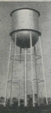
300,000 gal. cone roof, hemispherical bottom tank, 118' to top. Stillwater, Okla.
