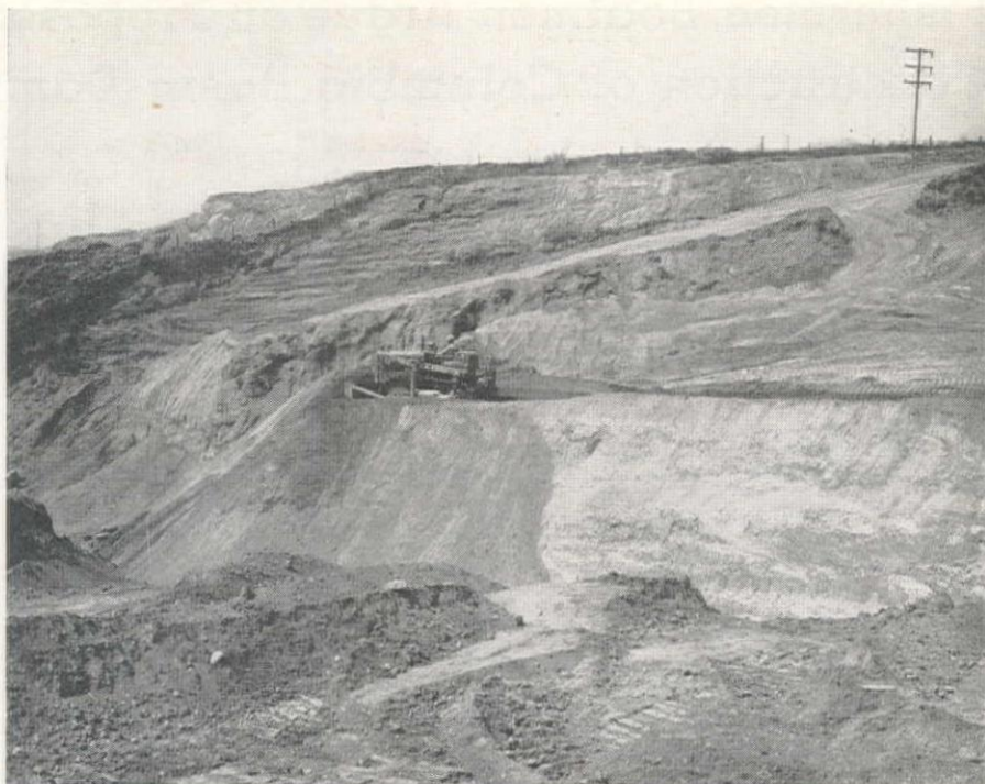
TRACTOR WORKS DECOMPOSED GRANITE PIT FOR ROADWAY SURFACING WORKING ON AN EXTENSIVE deposit of decomposed granite in Monterey Park on the easterly outskirts of Los Angeles, is an International tractor and bullgrader owned and operated by J. A. COOK. Tractor works material to edge of deposit and down to valley where it is picked up by loader. V. O. Kiger Co. works the granite deposit. The material cements firmly when rolled, and gives a non-muddy surface.
