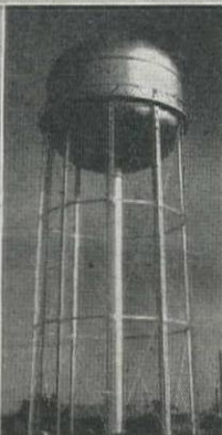
500,000 gal. double ellipsoidal tank, on 100' tower. Mission, Texas.
