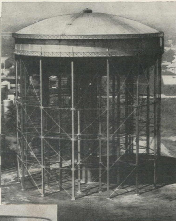
1,500,000 gal. toroidal bottom tank; structural tower. Diameter 103'4", head range 25'; height to bottom 85'. Fort Dodge, Iowa.
