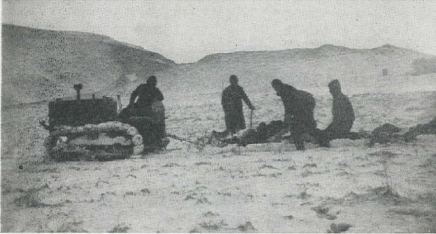
MATERIAL and equipment was unloaded on the beach with the aid of a small Cletrac and auto trailer (upper picture). Getting off the beach and inland was more of a problem than unloading. Improvised plow of timber and corrugated iron (in lower picture) pulled by Cletrac dug 1,200 ft. of 3½-ft. water pipe trench through thick tundra in less than five hours. By hand methods, it would have taken 24 man-days.
