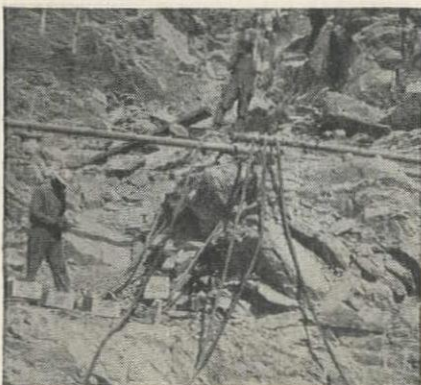
Typical wall of rock being excavated for dam foundation.
