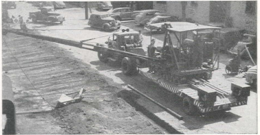
W-W Low-bed with 15 ton dragline working from bed.
