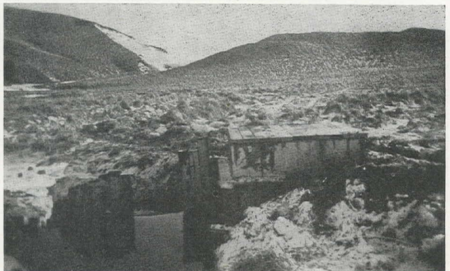
WATER SUPPLY structure at the Kiska outpost was constructed of T & C sheeting driven beside a creek and excavated inside to secure a four-foot water depth. Water was then pumped with a jet pump through 1,200-ft. pipeline.
