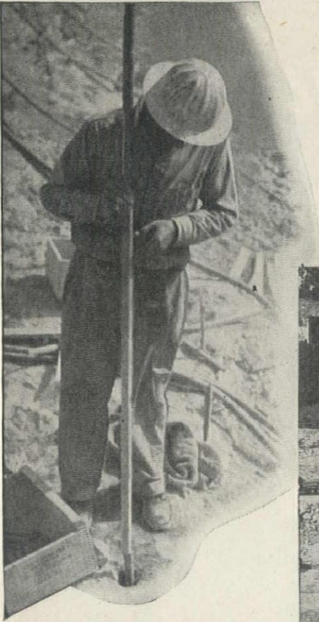
Loading Du Pont Special Gelatin in jack-hammer hole in solid rock at dam site.
