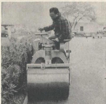
This illustrates a WHEELER TANDEM ROLLER compacting close to curb line.
