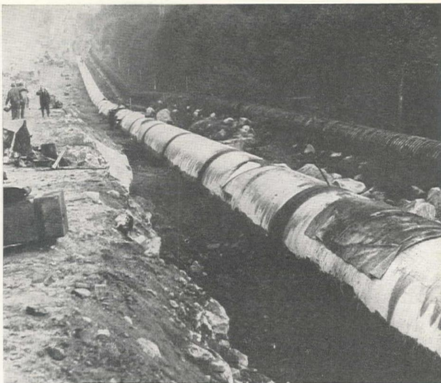
VANCOUVER, B. C., REPLACES WOOD STAVE PIPE LINE WITH STEEL
