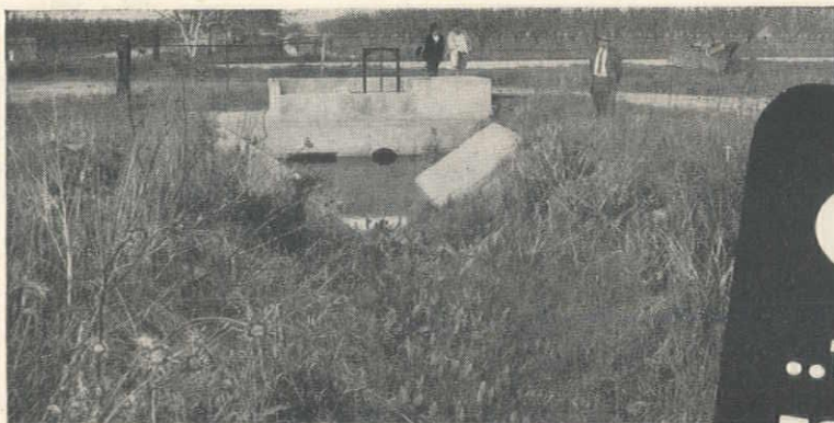
These irrigation ditches become choked by 4 to 15 inches of silt and tangled growth of weeds—must be cleaned yearly.
