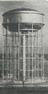
1,000,000 gal. toroidal bottom tank, diameter 76'9", height 127', head range 30'. Keokuk, Iowa.
