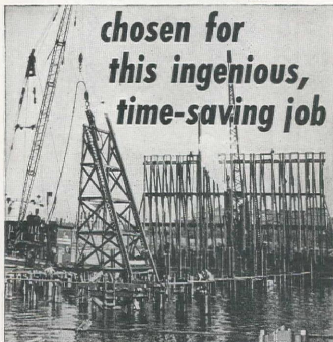
McKiernan-Terry Pile Hammers driving steel H-piles for the new 600-foot pier of Seatrains Lines, Inc. at Edgewater, N. J. The 9-B-3 hammer shown at left is driving batter piles. The 11-B-3 hammer at right is handling vertical piles.
