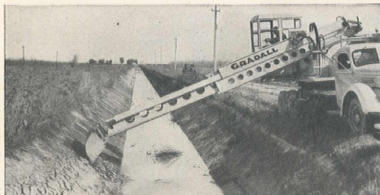
Long, powerful boom of the Gradall reaches across a 22-foot ditch, scrapes hard clay from ditch sides. Precision is a "must" to prevent damaging concrete ditch lining.
