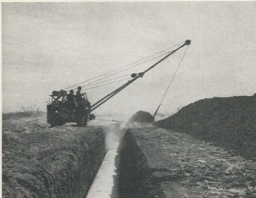
AFTER THE FINISHED pipe has been lowered into the ditch a tractor with drag line attached to the side boom fills the ditch at the speed of 3,000 ft. per hour. Approximately 1\frac{1}{4} to 1\frac{1}{2} miles per day of construction is being completed on the job.
