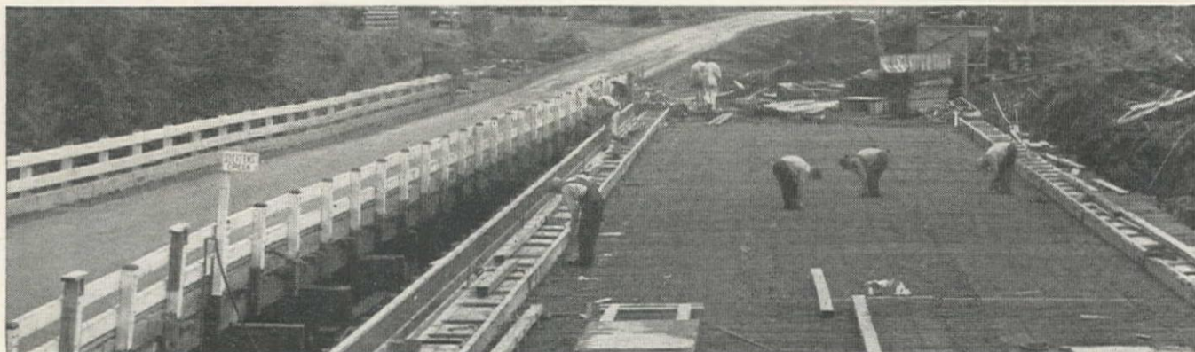
Approximately 90 tons of Bethlehem Pacific reinforcing bars were used in this highway bridge across Steffens Creek in Washington. Contractor: Rumsey and Company, Seattle.
