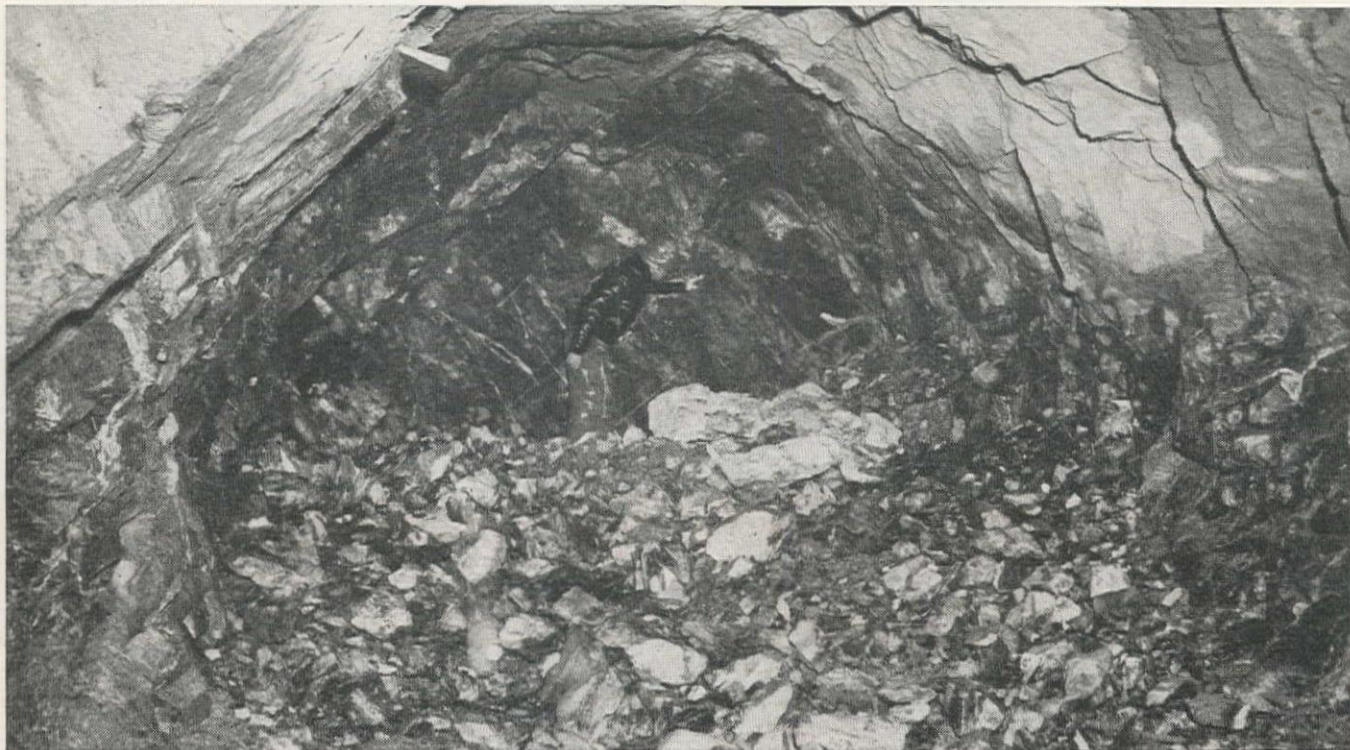
Good fumes permit early return to tunnel heading after "Gelex" shot. Note well-fragmented rock in foreground.
