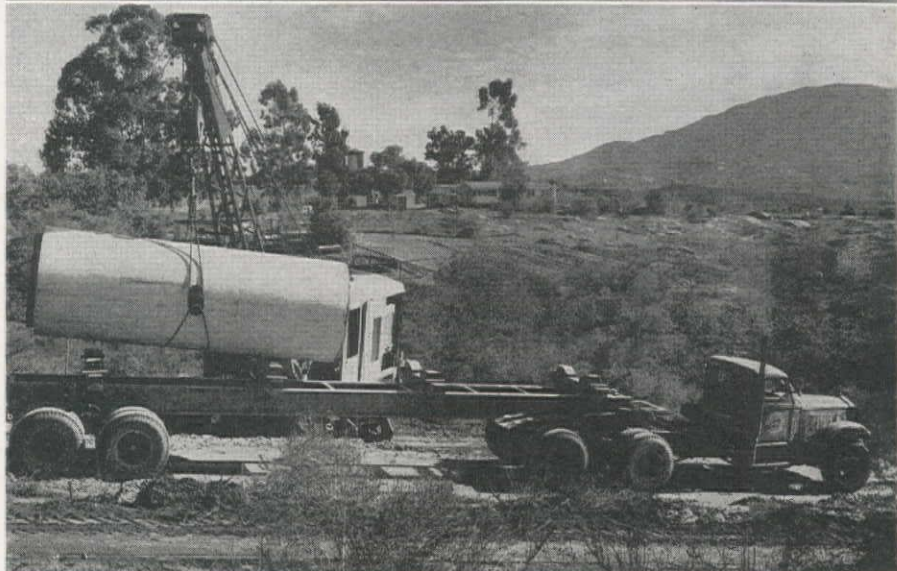
CARAVAN of the specially-constructed trailers carrying pre-cast concrete pipe to the San Diego Aqueduct. The two lengths of pipe on each truck weigh up to 46,000 lb. Below, a section of pipe being lifted onto the 18-wheel, 35-ft. semitrailer.
