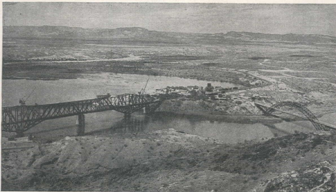
FORMER RAILROAD bridge owned by Santa Fe Railway (left) over Colorado River at Topock, Ariz., has been redecked by State Highway Departments of the two states, to replace the very light steel arch span at right, which will be demolished. When this photo was taken, work was just starting on new rail bridge behind the bridge at left. It is now completed.
