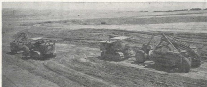
Scraper wagons grading the canal floor. Bethlehem Form-Set Wire Rope is used to rig these machines.
