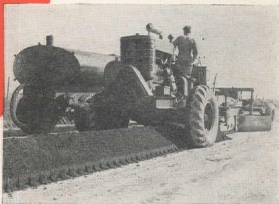
Above: Windrow entering mixing drum. Below: Thoroughly mixed windrow ready for spreading. Mixer takes binder directly from tank truck.
