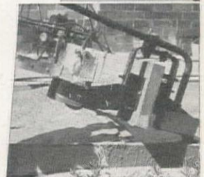
For Second Pass or Transportation Along Forms. The Screed is Elevated Clear of Slab.
