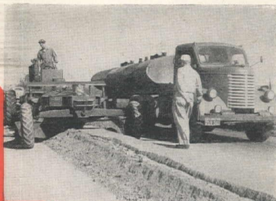
Above: Windrow entering mixing drum. Below: Thoroughly mixed windrow ready for spreading. Mixer takes binder directly from tank truck.
