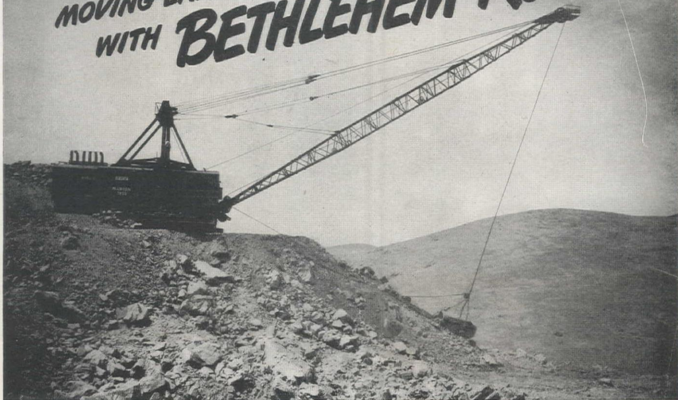
Walking dragline operating on the Friant-Kern Canal project. The 5 cu yd bucket weighs 30,000 lbs loaded. Bethlehem 1½-in Form-Set drag lines and 1⅝-in. hoist lines are used on this equipment.
