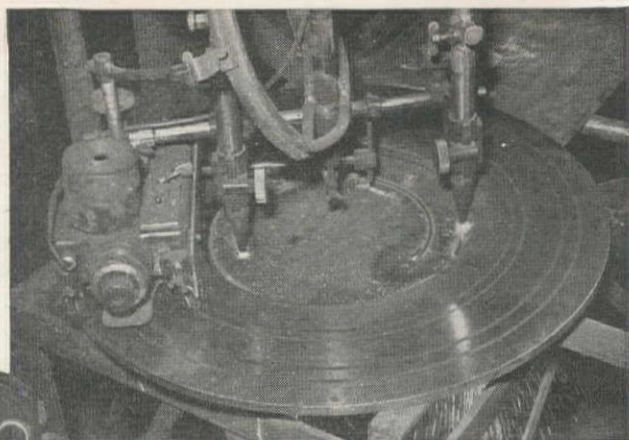
Airco No. 10 Radiagraph set-up for cutting inside and outside circles.
