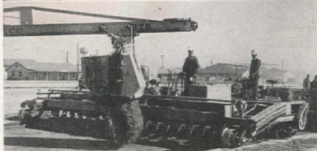
Jaeger Screw Spreader remixing as it places stiff material.
