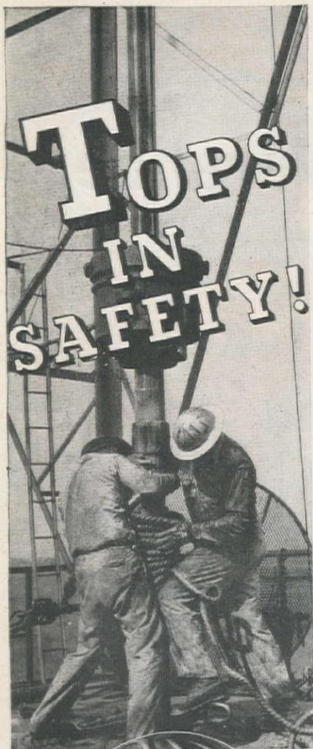
"Stabbing pipe in oil field"
