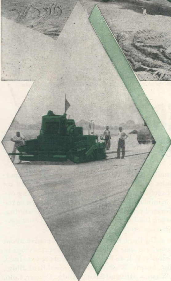
The B-G Tamping-Leveling Finisher will lay any mix, hot or cold. Places a continuous ridge-free surface with each succeeding strip firmly compacted against the previous one.
