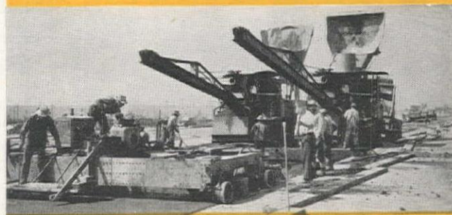
Jaeger High Speed Finisher sets fast pace for two big pavers.
