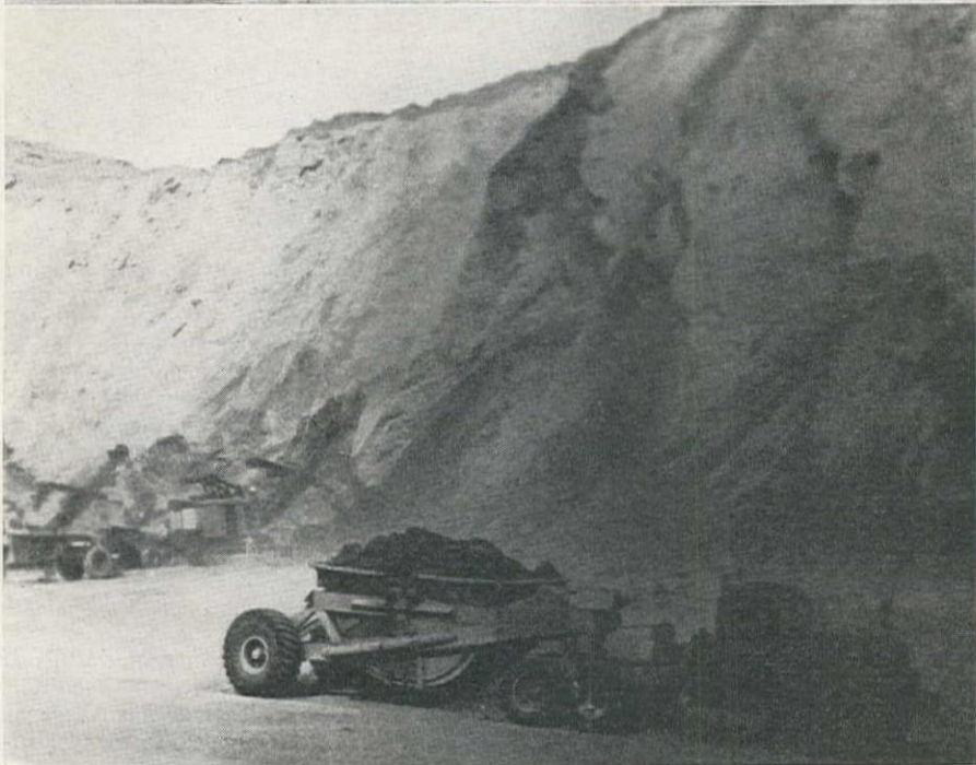
IN THE QUARRY , dirt is loosened on the upper benches by tractor-drawn rippers and bulldozed over the edge to the floor of the pit, top. On the lower level it is loaded by shovels into 13-cu. yd. Euclids, 16.3-cu.yd. Dixon Wagons (foreground) or 27-cu. yd. Peterbilts. They transport the material on an average headway of 26 sec.
