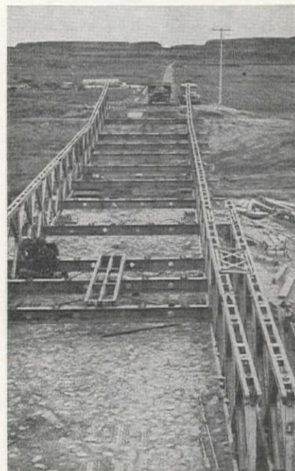
BRIDGES were constructed on the bank, then pushed across the Columbia Basin's main canal. Below, a former army weapons carrier makes a test run over the recently installed bridge.
