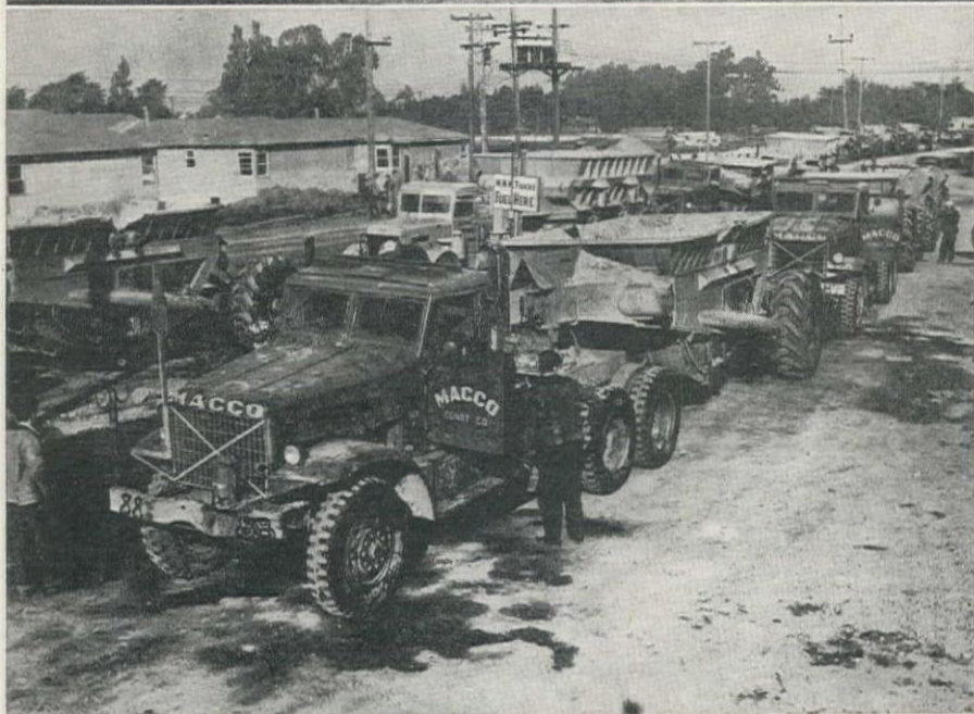
TRUCK YARD of Macco-Morrison-Knudsen on the San Francisco Airport Project. A fleet of 85 trucks is used on the fill. Above, are shown Euclids on the left and Peterbilts with special bodies on the right; below, Dixon Wagons being serviced in yard.
