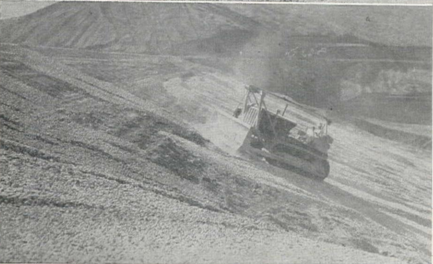
SPILLWAY EXCAVATION , Dos Pueblos Ranch Dam, top. During construction the dam was raised in 6-in. lifts, middle photo. To protect against wave action the upstream slope was covered with a gravel blanket 6 in. deep, bottom photo. The top of the dam is 20 ft. wide with a 6-in. crown and is surfaced with oil for road usage.
