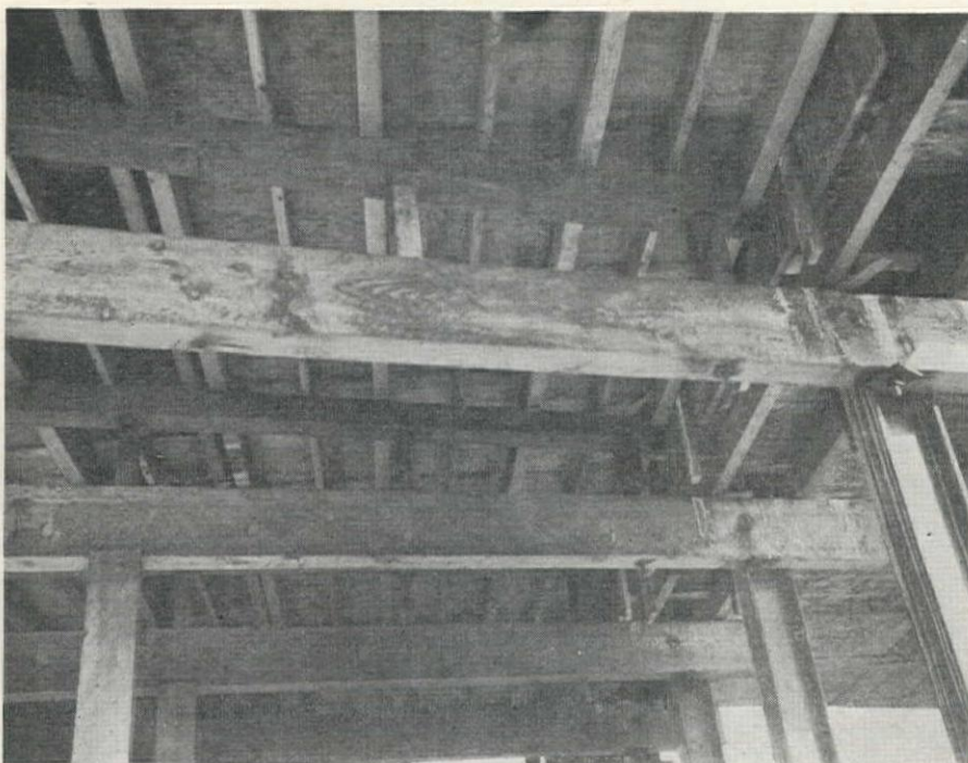
UNDERNEATH construction of the trestle deck forms. The 14-in. steel I-beam pilings are surmounted by a concrete beam and slab deck. J. D. Proctor, Inc., and B. W. Kuhn, contractors, are the first to make a major application of the plastic coating.
