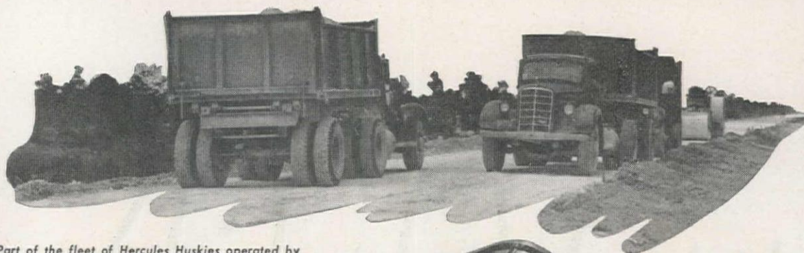
Part of the fleet of Hercules Huskies operated by the R. B. Tyler Company on a road construction project near Miami, Florida. Working 24 hours a day, these semi-trailer dump bodies carry 12 cubic yards per trip over a 44-mile round trip route.
