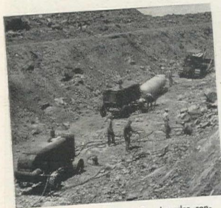
Section of the Friant-Kern Canal under construction by Peter Kiewit Sons' Company. Bethlehem Hollow Drill Steel is used here.
