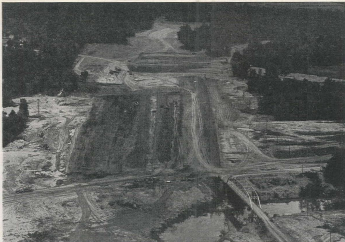
AIR VIEW of the main embankment at Wister Dam site. Tractors and Euclids in center foreground are placing fill at approximate elevation 462. Poteau River is in the foreground, with the observation pavilion in upper center.
