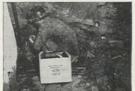
(AT TOP)—"Jumbo" has been drawn back to allow crew to load pyramid-cut round in face of 16 x 18-foot pilot tunnel, later enlarged to 35-foot width.
