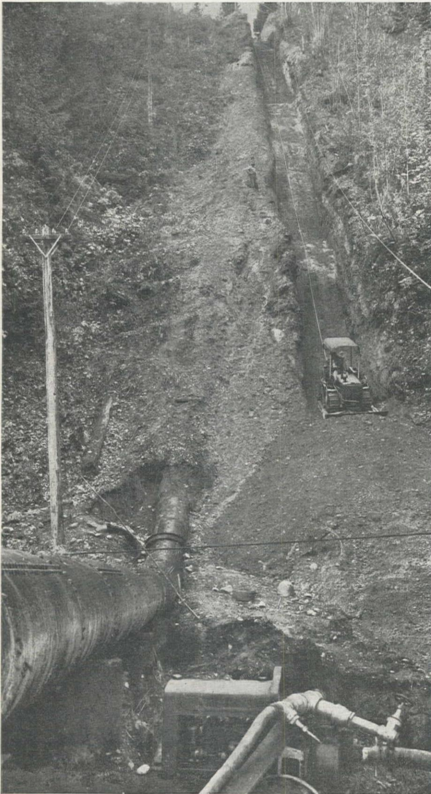
EXCAVATING THE TRENCH on 50 per cent slopes was accomplished by a bulldozer attached to a tractor anchored at the top of the slope. After making each downhill pass, the bulldozer was pulled up by the cable winch on the anchored tractor. The new line parallels the existing pipe crossing the Puyallup Valley, with similar diameter.
