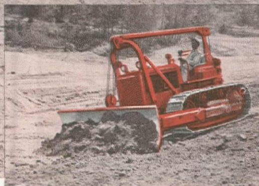
This International TD-14 with Trail-builder is shown leveling a haul road on approach to the levee. It also dressed the levee to grade and leveled off the dirt deposited by the three TD-18's and scoops. This is a fast, powerful and easy-to-handle Diesel Crawler—ideal for this work.
