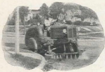
MODEL "40" PATROL SWEEPER —Available with right-hand or left-hand gutter broom, or both. Rear broom throws dirt directly into hopper. May be had with Leaf Broom attachment.
