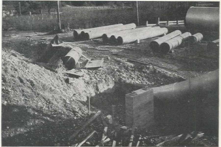
CONCRETE PIER at east end of the Puyallup River bridge will eventually support a hinged strut and permit deflection in the line between the bridge abutment and the sub-surface section. Strut and rollers will eliminate stress on bridge floor beams.
