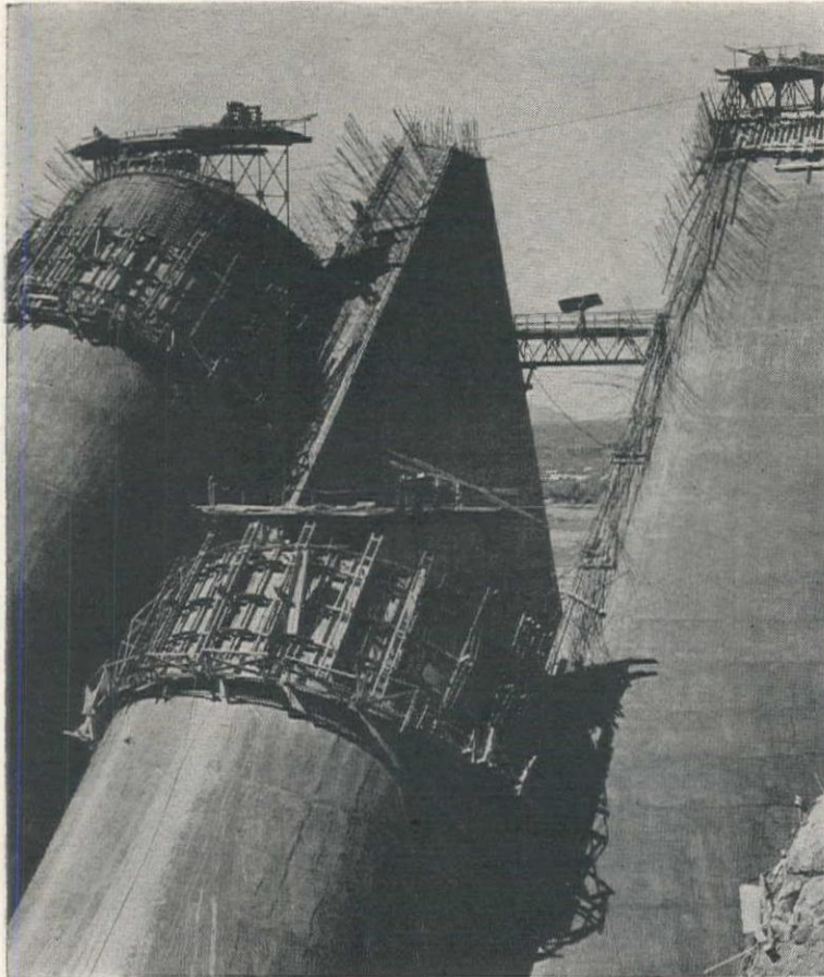
Tapered arch forms used in constructing Arizona dam.
