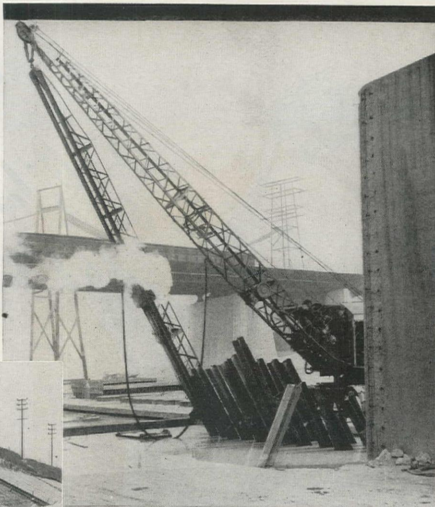
Bethlehem H-Piles being driven for pier extensions in the Los Angeles River Channel Improvement project.
