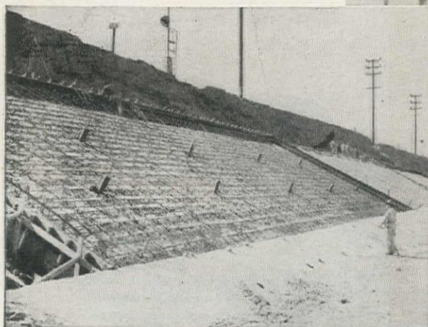
Slope paving operation showing Bethlehem Reinforcing Bars in position. The "weeps" projecting from the slope are to insure drainage from behind the wall.
