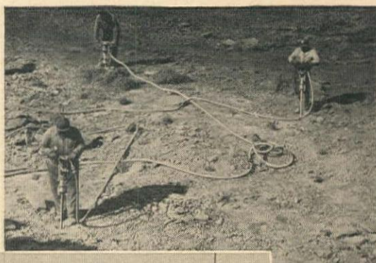
Above—Small, out-of-the-way areas were drilled quickly and efficiently with I-R Jackhamers.
