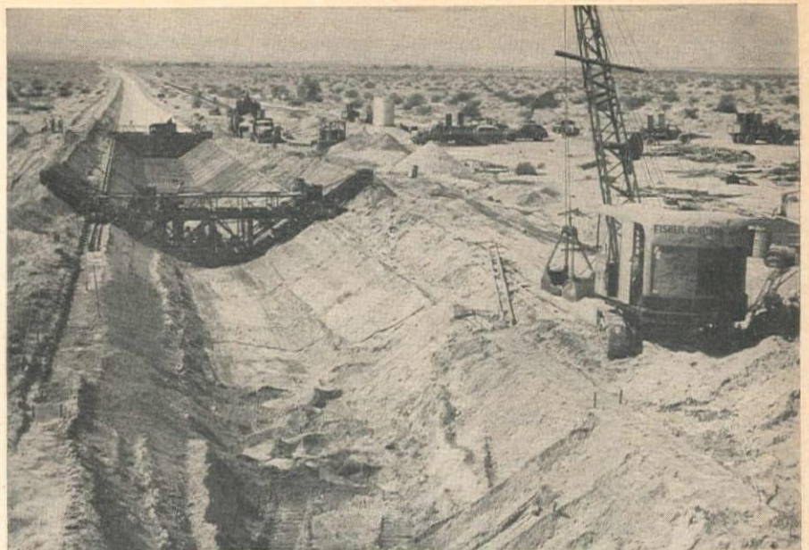
INTEGRATED OPERATION on the Coachella Canal Wasteway; foreground, clamshell owned by Fisher Contracting Co., Phoenix, Ariz., performs rough excavation; center, trimmer finishes excavation, here casting spoil on each bank; next, reinforcement net is laid; finally, paver and lining machine place concrete lining for the canal.
