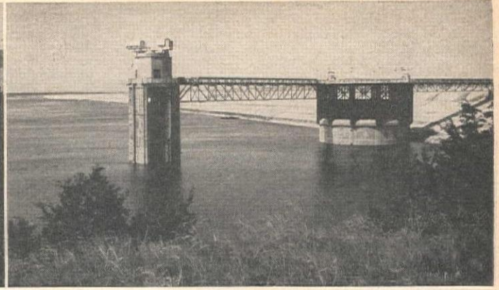
KINGSLEY DAM after completion showing the wave wall and state highway (left), morning glory spillway and outlet control tower (right).
