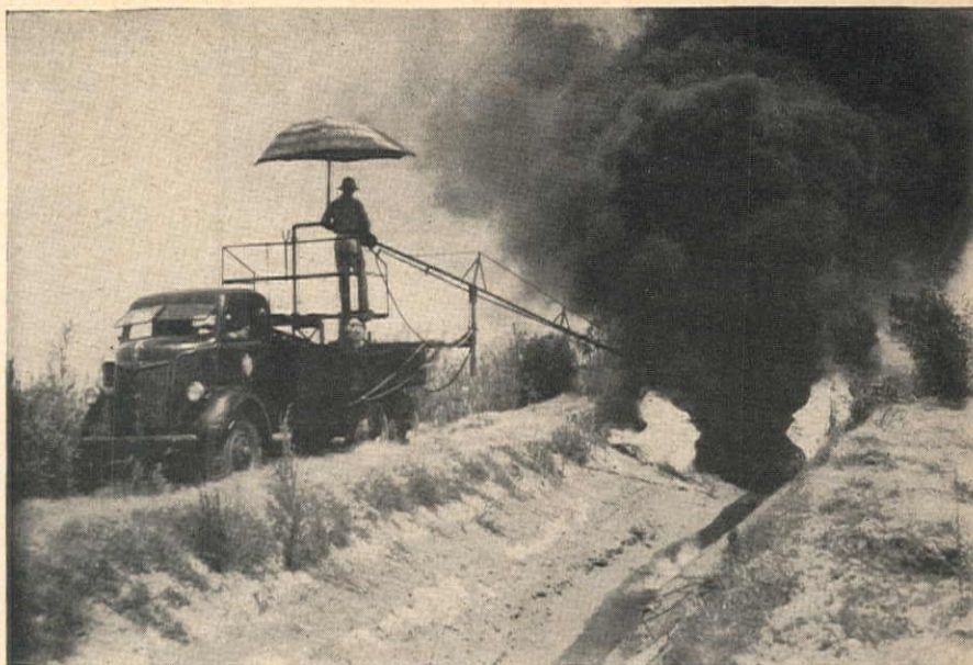
ONE OF the Imperial Irrigation District truck units at work. Cost of the weed burning by this method is about $10 per mi. and is recommended for use by irrigation districts. Approximately 18,000 mi. of ditch bank is burned yearly in a section of the country where weed control is very difficult.
