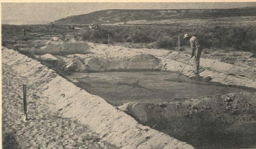
PUDDLED EARTH TO FORM LINING OF PASCO CANALS
