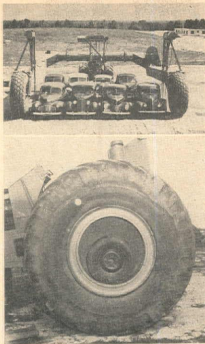
SIZE OF giant machine is seen in these pictures. Top, eight cars are parked in trailer's arms. Below, ordinary 6.00 x 16 automobile tire is dwarfed in comparison to 30x40 9-ft. high pneumatic tires.
