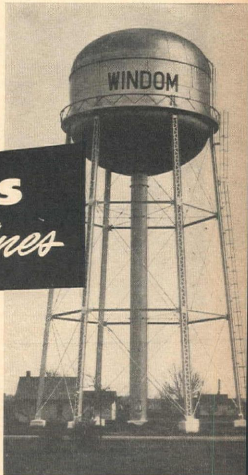
WINDOM, Kan.—300,000 gallon double-ellipsoidal tank, 42' diameter, on 75' tower.
