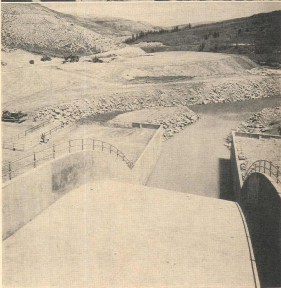
LOOKING UPSTREAM into spillway during construction (top) shows walls in place and forms and reinforcement ready for the floor. Two rows of dentates visible in foreground dissipate energy developed by 46-ft. fall to stilling basin, shown below.
