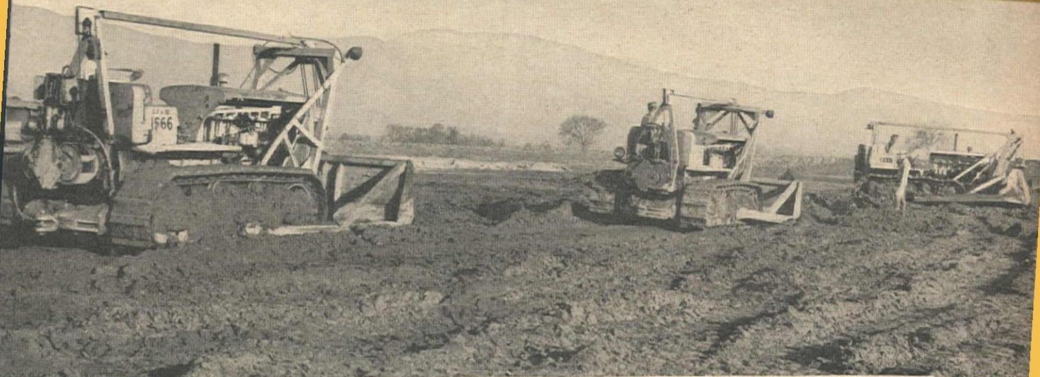
Part of Guy F. Atkinson Co.'s fleet of 18 "Caterpillar" Diesel D8 Tractors at work on the San Jacinto Navy reservoir contract.
