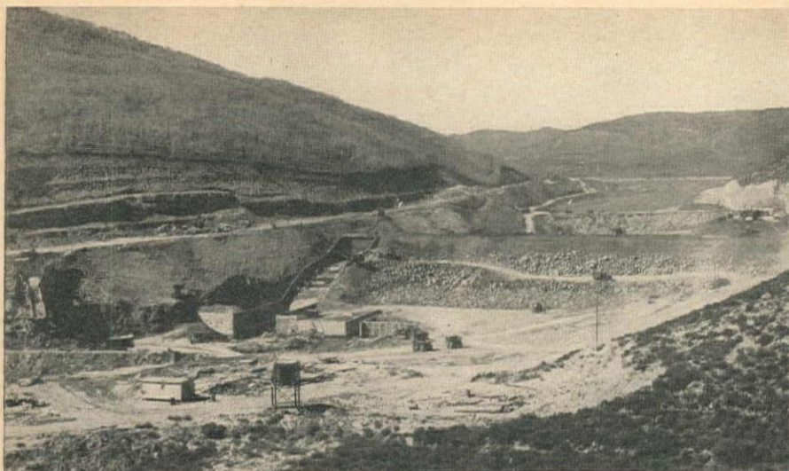
LOOKING UPSTREAM from below the reservoir, the railroad track is on left of the abutment. While construction was still under way the old dam and spillway at the back were still in use. The first Scofield Dam partially failed in 1928 and despite subsequent repairs the storage capacity was cut to less than half original amount.
