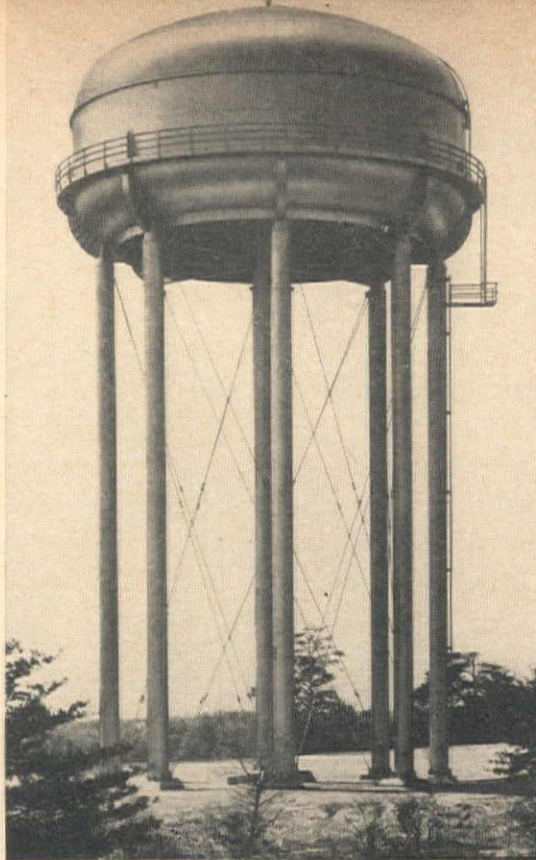
ARLINGTON COUNTY, Va.—500,000 gallon toroidal bottom tank, 60' diameter, on 81' tubular column tower.
