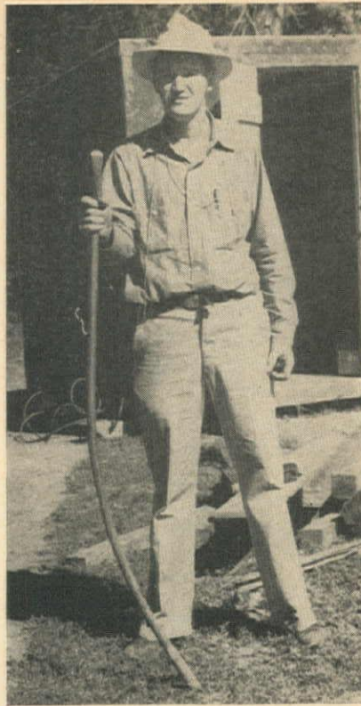
GLEN WILSON , field inspector, holds curved tamping bar which reaches to the bottom of trench. Rod is used for backfilling and hand tamping to the spring line. Backfilling above is done with a small bulldozer, and pneumatic tampers are used to obtain sufficient compaction.
