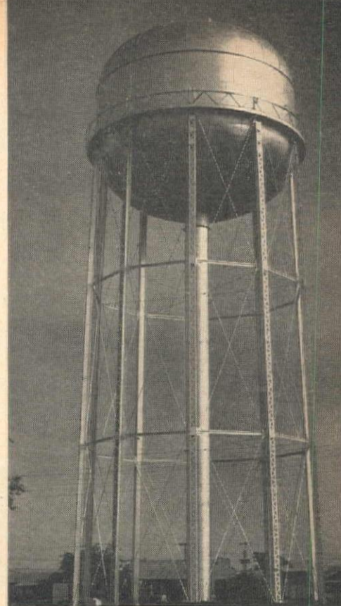
MISSION, Tex.—500,000 gallon double-ellipsoidal tank, 50' diameter, on 100' tower.
