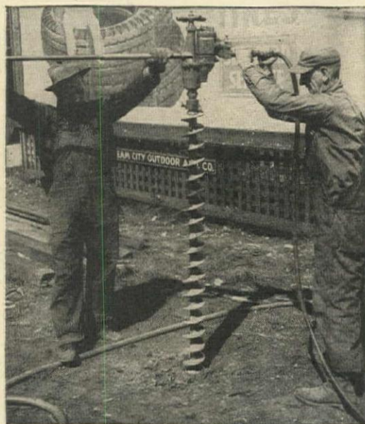
THOR 264RY Air Drill with auger steel: "... a mechanical digger that works wonders. We enjoy freedom from the arduous digging of post holes. We now have uniform depth of holes, which adds increased safety and freedom from 'blowdowns'."
