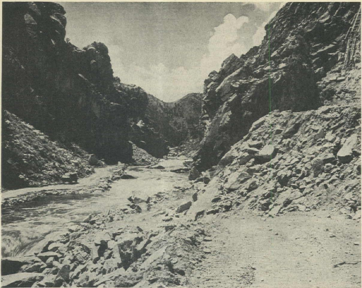
SITE OF Kortes Dam which will harness power for Western development is in this narrow gorge, Black Canyon, cut by the North Platte River. Aggregate from deposits downstream will be hauled to the site over construction road at left.
