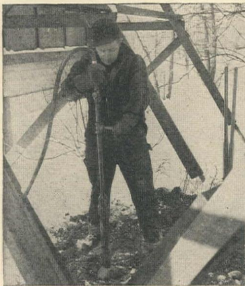
THOR 60BFT Tamper: "Gives immediate, firm support to posts, such as we used to achieve only after the board had been built for years."
