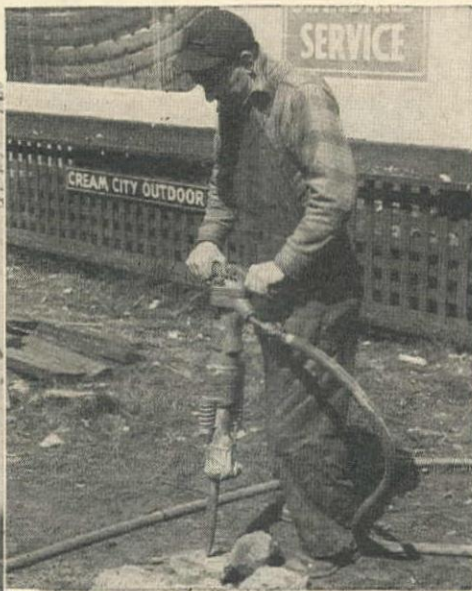
THOR PAVING BREAKERS do fast demolition on pavements, columns, walls, piers, foundations, etc.
