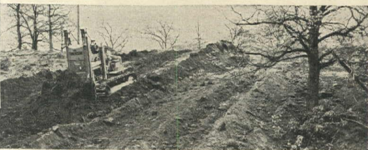
Big T7 TRAXCAVATOR grading and landscaping residential grounds in a Minneapolis suburb
