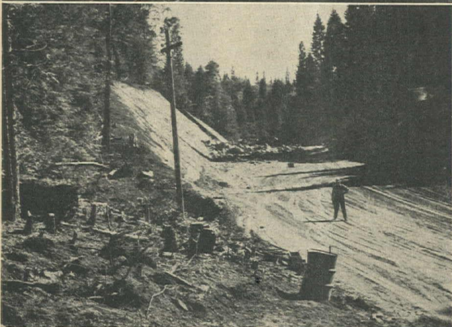
NEW GENTLE curves replace sharp turns of old road, far side at top left. Bottom, Forest Highway 32-K begins to look like a beautiful piece of road, matched only by the scenery, with cuts and fills nicely balanced, despite considerable overhaul yardage.
