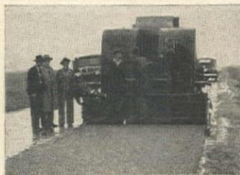
Resurfacing Michigan Road with the Moto-Paver
