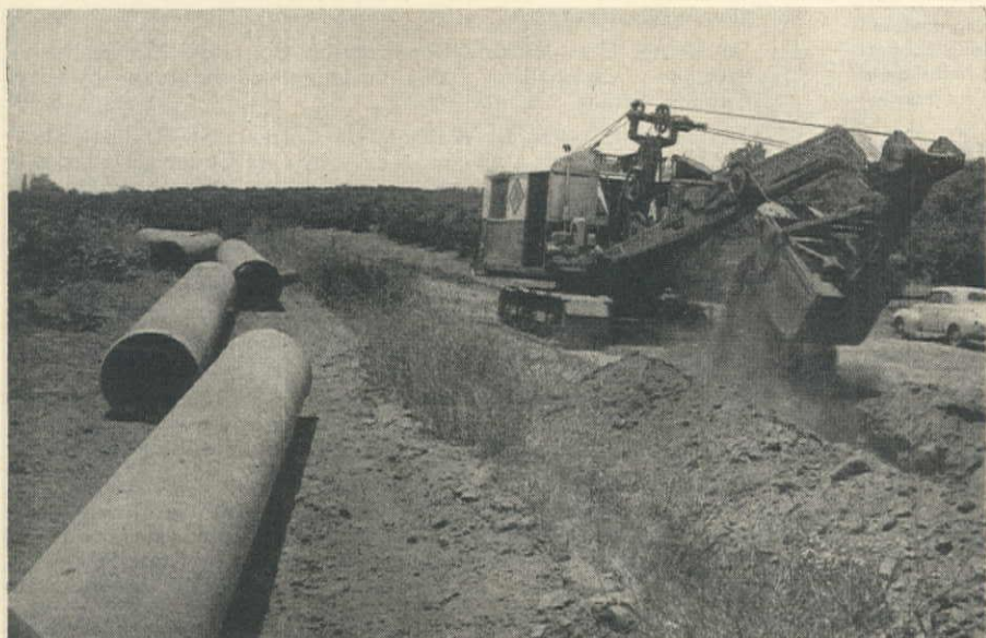
Installation of 17,000 feet of 21", 24" and 27" diameter American Concrete Cylinder Pipe for the Escondido Mutual Water Company, Escondido, California. Maximum operating design pressure on the water supply line—150 pounds.
