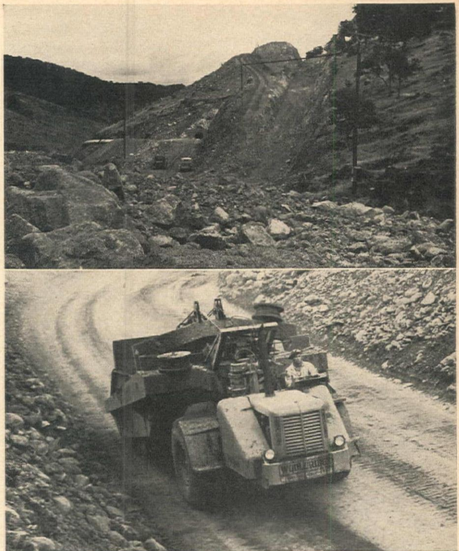
SPILLWAY CUT (top) through solid rock was excavated with tractors and scrapers, after shooting, working up grade to protect workers at the tunnel outlet portal. Roads from the borrow pits (bottom) are two lanes in width and one way in direction to permit both high and low speed equipment to move back and forth without interference.
