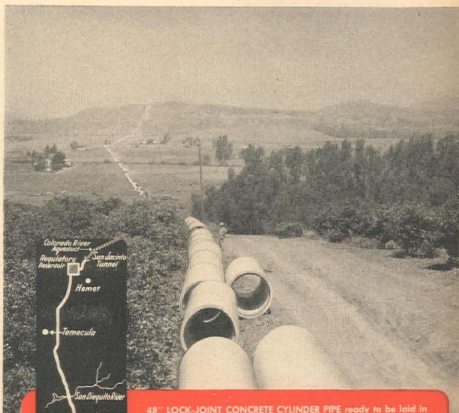
48" LOCK-JOINT CONCRETE CYLINDER PIPE ready to be laid in the southern section of the aqueduct . . . from Oat Hills Tunnel to San Vicente Reservoir . . .
