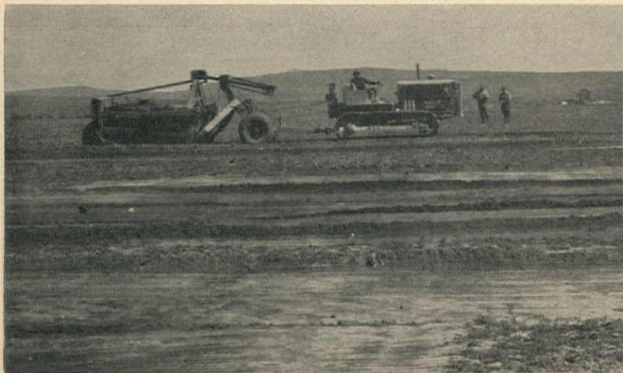
A LARGE carryall scraper is pulled by a heavy tractor on leveling project in Oregon. Water in foreground emphasizes one need for leveling program—farm drainage.
