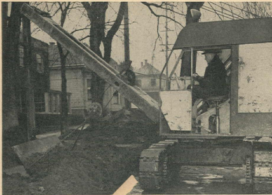
BACKFILLING the pipe trench after testing the individual joint welds was done by a backhoe with the bucket reversed by an open blade. Excavation of the 8-ft. trench was complicated by the maze of utility services underlying the city streets.
