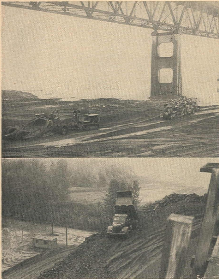
LOADING SAND for fill on Longview Bridge approach, at dredging deposit underneath the structure, top. Spreading rock for blanket on the fill slopes; the rock blanket is 10 ft. thick. Blanket rock was secured from quarry at Oregon end.
