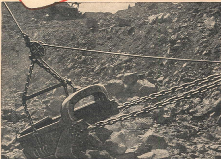
ESCO 4½ yard dragline bucket on SW Monaghan working on Friant Canal, in California
