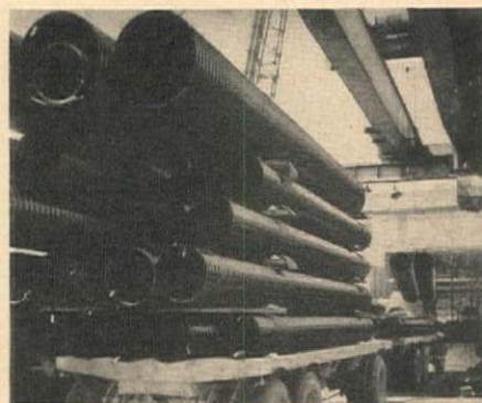
Loading asphalt dipped culvert pipe for shipment to big drainage project.
