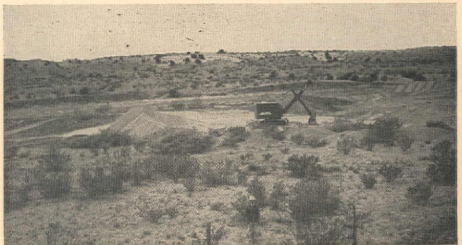
TYPICAL GRAVEL deposit in New Mexico. These deposits are apt to be too small for adequate supply of material, and are often impregnated with various alkali salts.
