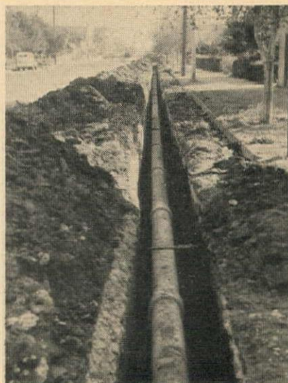
IN THE TRENCH , man-hours are cut. Fewer men are needed for handling. Most sizes can be installed without mechanical handling equipment.
