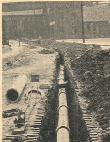
UNDER HEAVY TRAFFIC the Simplex Coupling provides a flexible joint that effectively withstands vibration—absorbs the shocks of heavy vehicles.
