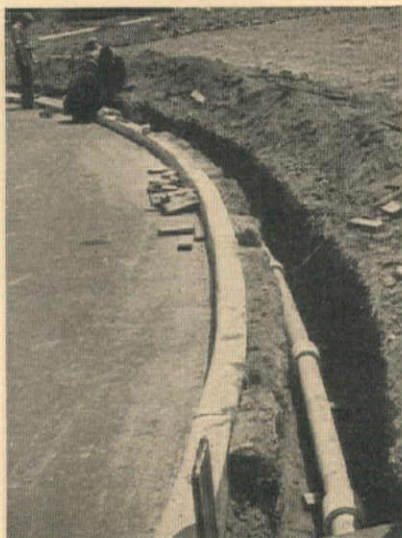
ON CURVES and in hilly terrain, Transite Pipe's flexible Simplex Coupling permits up to 5° deflection at each joint without use of fittings.
