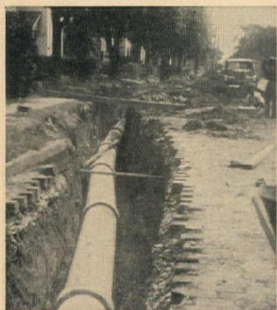
AS DISTRIBUTION MAINS , Transite Pipe cannot cause "red water." Its high corrosion resistance means low maintenance over the years.
