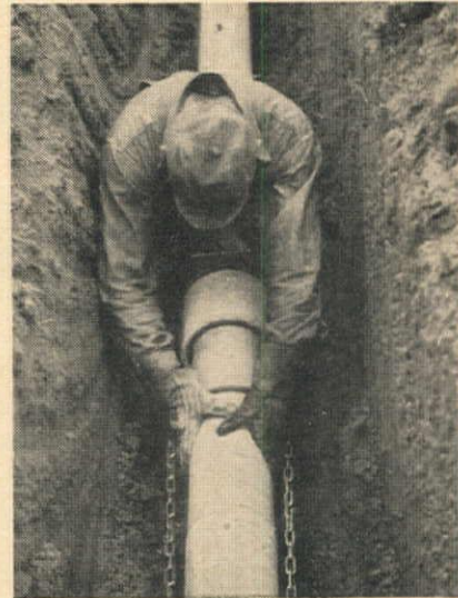
AT THE JOINTS , Simplex Couplings mean quick, easy assembly. They safeguard against underground leakage and undermining of supporting soil.
