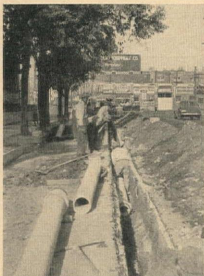
UNDER CITY STREETS , Transite saves by permitting narrower trenches, reducing disturbance to pavement. Fast assembly minimizes traffic tie-ups.
