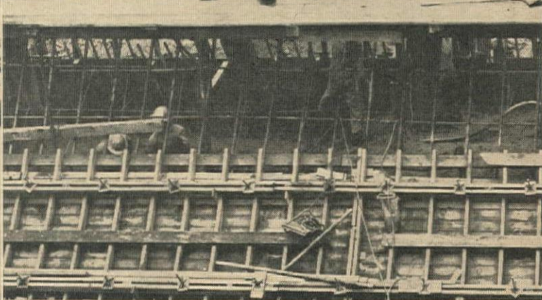
INTERIOR VIEW of control tunnel 2 looking upstream toward needle valves, upper left, showing contact line between original lining and new invert excavated to depth of 18 in. Top right is excavation for deflector construction, with top 40 in. hand-chipped so original reinforcement will be retained. At lower left is cut and cover extension of tunnel 1 with lining of invert being removed for replacement by continuous 25-ft. radius section. Above is detail view of concrete pour in sidewall section of tunnel extension. Concrete in background seals seepage cavern.
