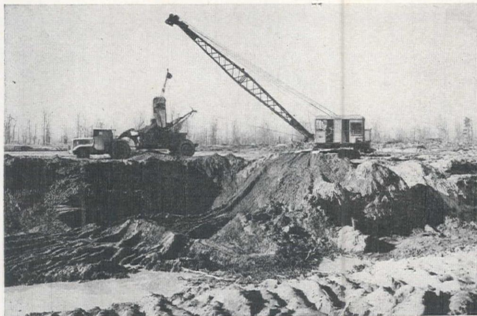
This 2-yard Lorain-82 Dragline...the 5th profit-making Lorain machine for Leonard & Slate of Multnomah, Oregon...is shown here working in a borrow pit on the Troutdale-Wahkeena Creek Section of Columbia River Highway. 260,000 yards of borrow excavation and approximately 240,000 yards of general excavation are involved in the project.
