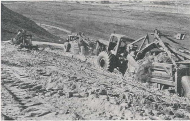
Rooted Sandstone . . . LeTourneau heavy-duty Rooter breaks up sandstone and dry clay to speed Tournapull loading.
