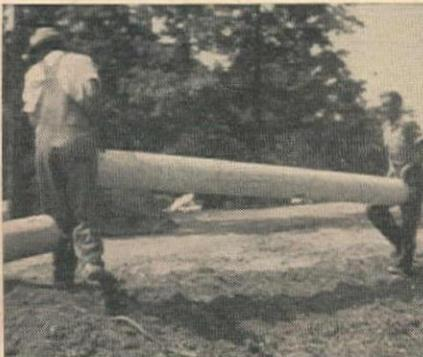
**HANDLING COSTS** too, are low. Fewer man-hours are required for unloading and lowering into the trench. Only the larger sizes require mechanical handling equipment.
