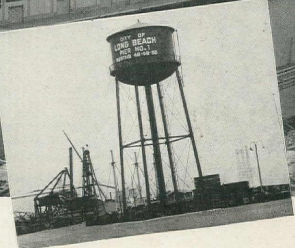
ONE of the best formulas for protecting property and human lives from fire is an automatic sprinkler system plus gravity water pressure. The City of Long Beach, California, uses this type of fire protection for its Pier No. 1 in the Cerritos Channel as shown in the views on this page. This pier is adjacent to Pier No. 2 which suffered a disastrous fire recently.
