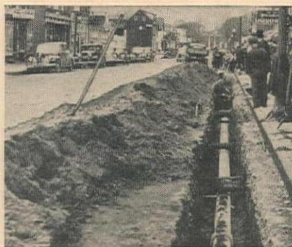
**MAINTENANCE COSTS** are cut with Transite. Its tight joints, high uniform strength, proven durability and corrosion-resistance all contribute to its economical performance.
