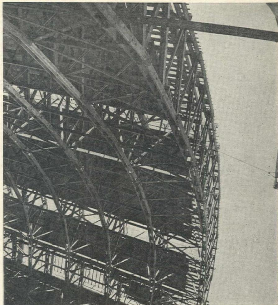
**TIMBER TRUSS** construction on one of the blimp hangars erected at Santa Ana, Calif., similar in all details to those destroyed by wind and fire in Florida hurricane.
