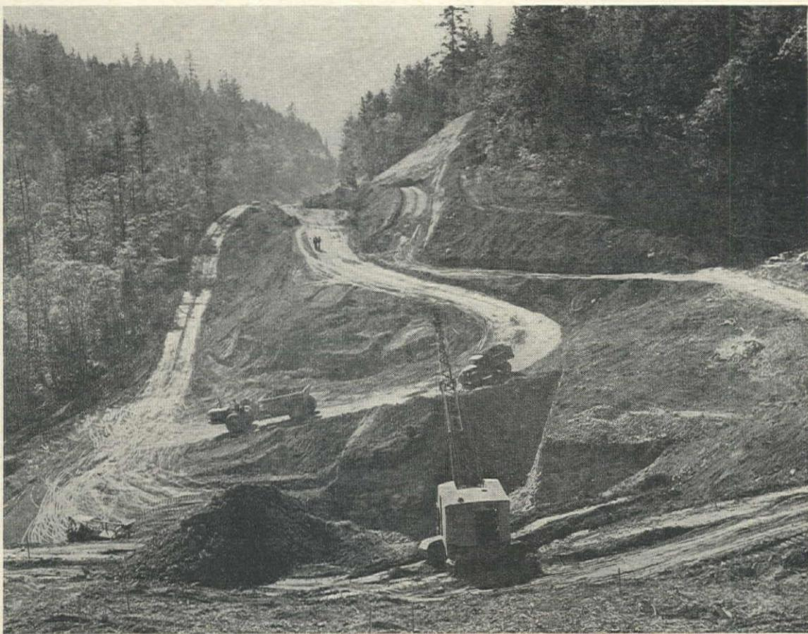
EARTH-MOVING EQUIPMENT backfilling with rock around a culvert and one of the typical embankment stabilization trenches for a big fill on the Grave Creek-Wolf Creek highway project, which involves over 866,000 cu. yd. of excavation.
