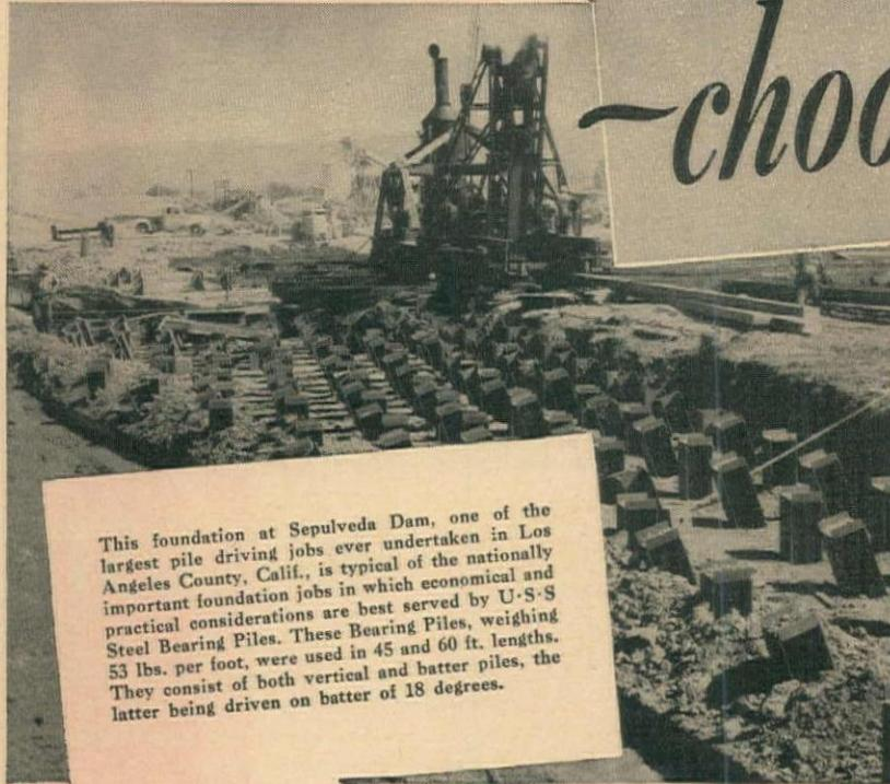
This foundation at Sepulveda Dam, one of the largest pile driving jobs ever undertaken in Los Angeles County, Calif., is typical of the nationally important foundation jobs in which economical and practical considerations are best served by U-S-S Steel Bearing Piles. These Bearing Piles, weighing 53 lbs. per foot, were used in 45 and 60 ft. lengths. They consist of both vertical and batter piles, the latter being driven on batter of 18 degrees.
