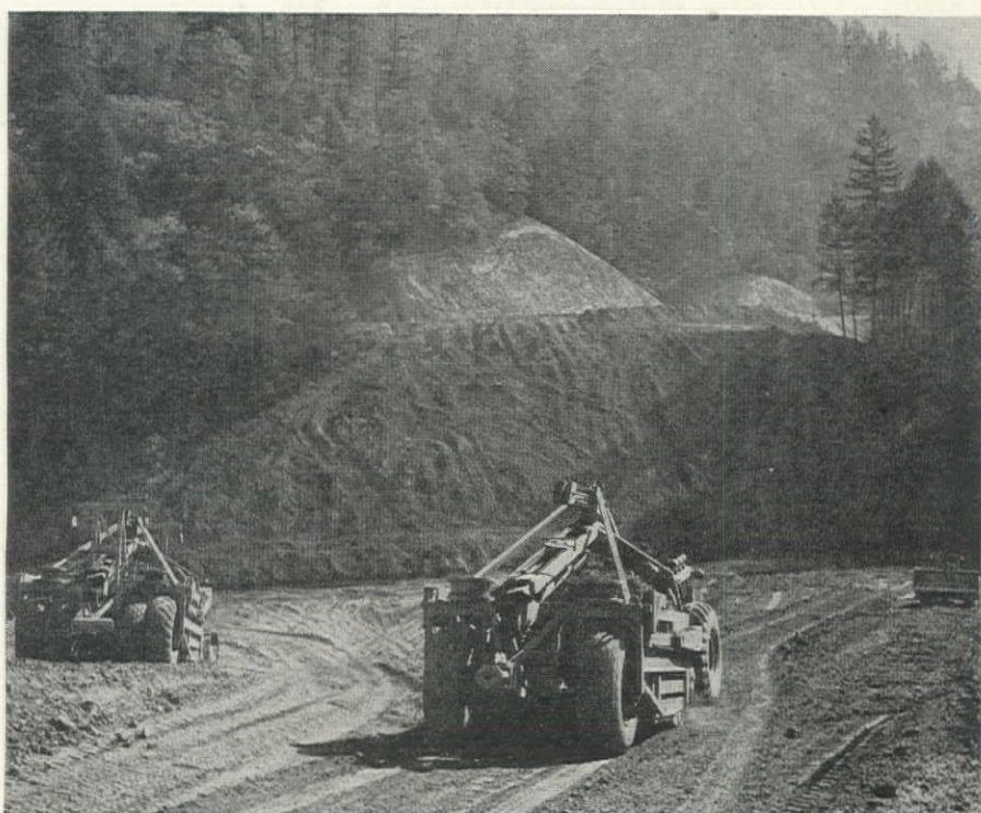
**EMBANKMENT CONSTRUCTION** on the Roseburg highway section. Below, rock backfilling over a culvert. Weepholes in culvert take care of side drainage. The other pictures show heavy equipment depositing and rolling embankment fills. In the upper picture, the equipment is filling over one of culverts, bottom on sidehill.
