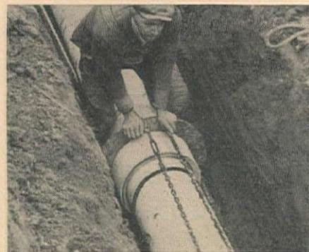
**ASSEMBLY COSTS** drop with Transite. The Simplex Coupling permits quick, easy assembly . . . assures joints that stay tight, even when the line is deflected as much as 5° at each coupling.
