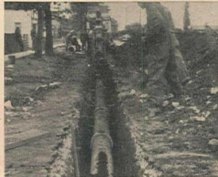
**EXCAVATING COSTS**, as shown above, are low with Transite. Trenches are narrow and disturbance to pavement is kept to a minimum. No bell holes are required at the joints.
