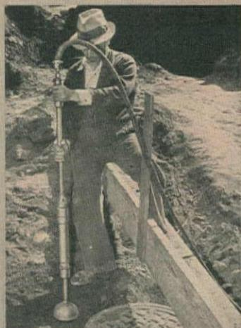
In trench work particularly, CP Backfill Tamers quickly earn their cost by saving the time and labor involved in hauling surplus excavated material. For general tamping, CP-3 is recommended; for heavy tamping CP-MM; for extremely heavy tamping CP-4 is preferred.
