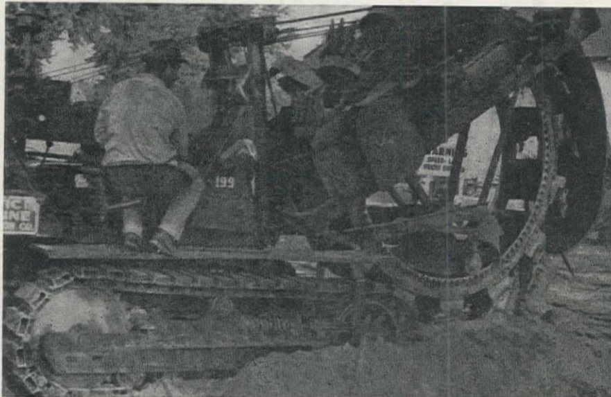
SPECIAL ROUND-NOSED follower attached to trencher digs semi-circular ditch to be used as outside form of pipe. Machine digs effectively through heavy adobe soil, producing smooth-bottomed trench.
