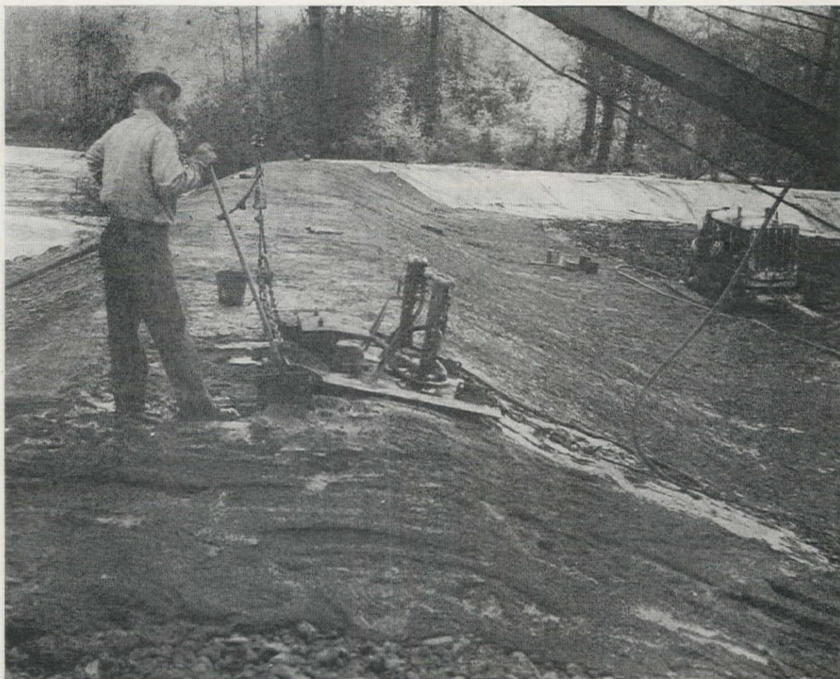
TOPPING THE SLOPE , is an especially constructed agitator used by the contractor to obtain deep bonding of the river rock composing the flood control levee. Shown above is the dragline boom carrying the air hose used to supply two jackhammers for vibrating this animated trowel. Completed portions of the revetment is slow-curing under wet fabric protection in the background.
