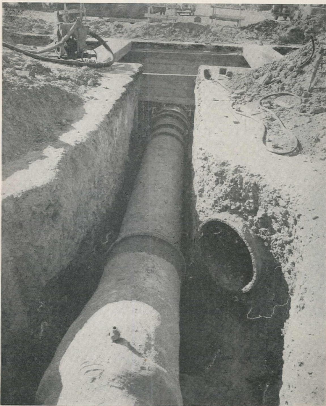
A connection on the Thorn Street Pipe Line, City of San Diego; 12,000 feet 36" Lock Joint Concrete Cylinder Pipe here connects into 30" cast iron pipe line. Reducer appears in foreground.
