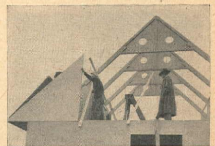
LOWER ROOF serves as horizontal bracing for fabricated plywood rafters of top roof. Over these is laid braced plywood roof decking. Gable ends are placed as decking is added. Insulation is attached to walls and ceiling panels.
