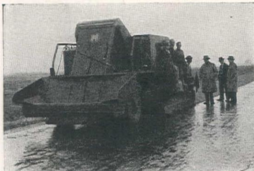
Resurfacing a Michigan Road with the Moto-paver
