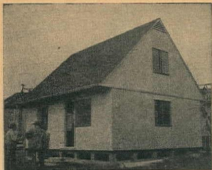
HOMEOLA IS completely enclosed in afternoon. No special equipment is needed because no wall or floor part weighs more than 75 pounds. This house is 20 x 24 ft., with large living room, dining section, kitchen and bathroom downstairs and two bedrooms upstairs.
