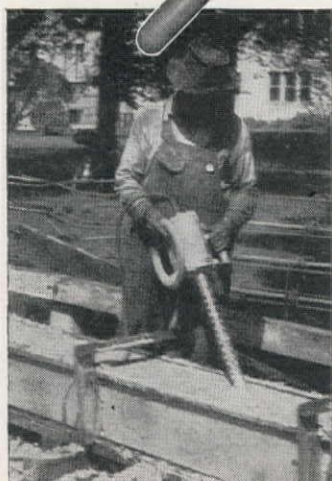
A JACKSON FS-7A Flexible Shaft Vibrator placing concrete in the manufacture of precast piling.
