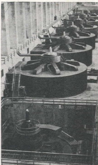
TWO GENERATORS borrowed from the powerhouse at Shasta dam for wartime use at Grand Coulee soon will be replaced with 108,000-kw. units. One of the loaned 75,000-kw. machines shown in line with the larger Coulee units.
