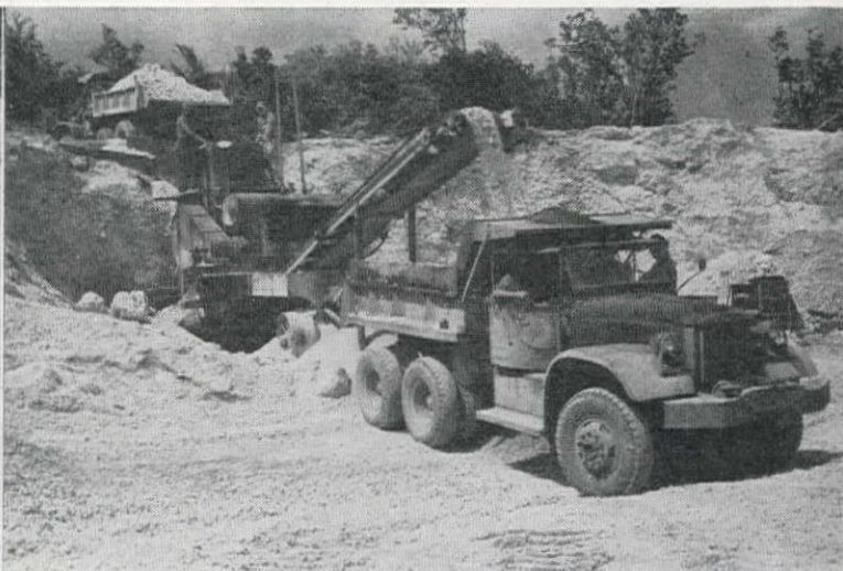
LOADING CORAL from one of many quarries located on Pacific islands, above left. A portable crushing plant with a conveyor belt loading surfacing material, right. Hard and accelerated digging, often by inexperienced operators during the initial stages of the campaign, caused a heavy toll in hoisting rope failures, lower left.
