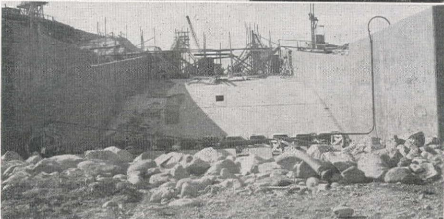
CONCRETE OPERATIONS at spillway. Top, contractor's mixing plant under construction. Next, spillway gate structure forms. Next, housing for winter curing of walls. Bottom, completed spillway apron.
