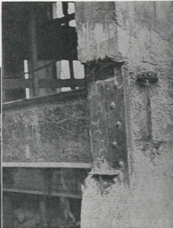
A THICK FLOOR SLAB and supporting girder removed from the original structure before the new construction was initiated, below. Removal of structural members up to 24 in. in size required multiple cutting to reduce them to sizes that could be easily removed from the building.
