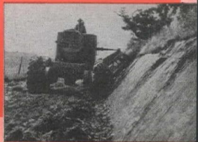
Adjustable blade makes bank cutting possible at any angle.
