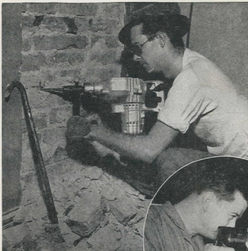
DEMOLITION IS QUICK and sure with the Thor-Nado portable electric hammer.
