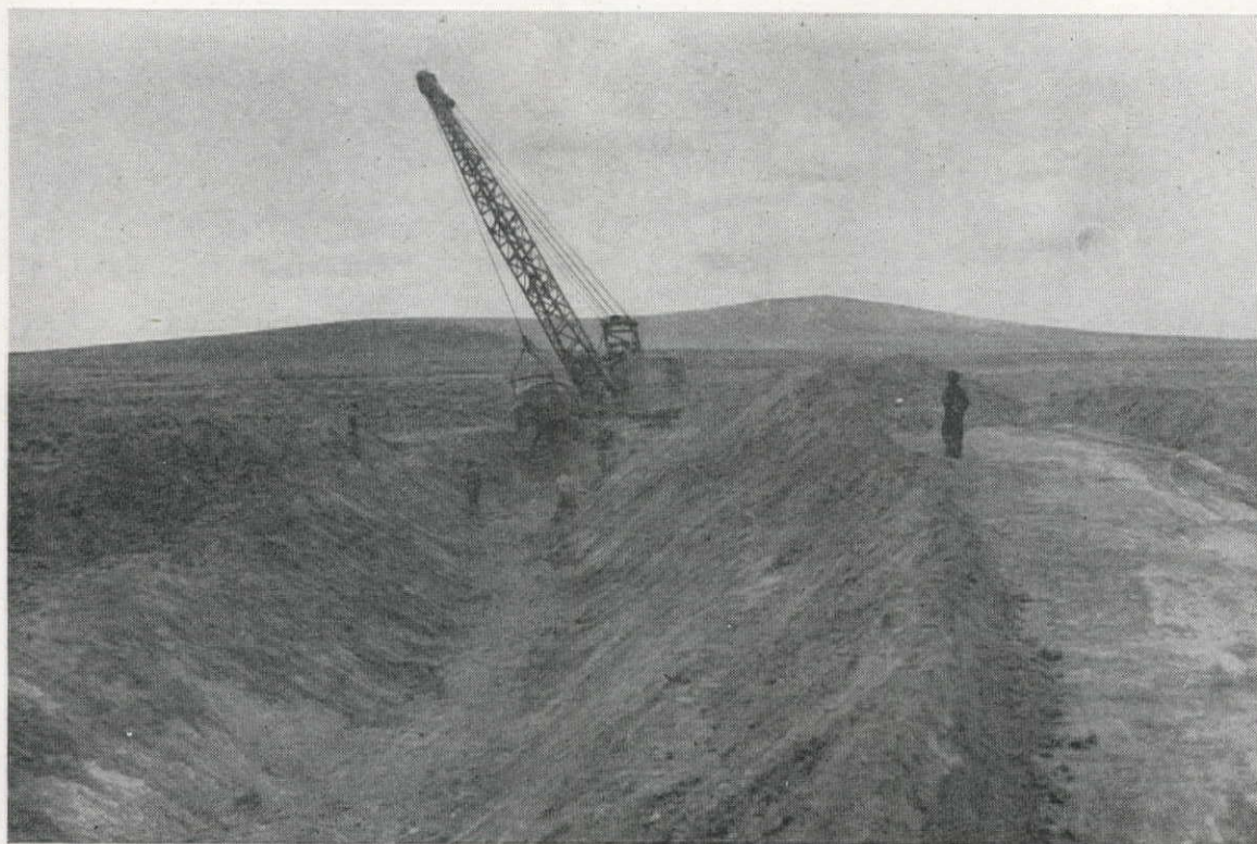
EXCAVATING MAIN YAKIMA Ridge Canal with 2-cu. yd. dragline. Two similar machines excavated over 185,000 cu. yd. of earth and rock on this project. Following the dragline is a three-man crew finishing the cut by hand sloping sides and bottom.
