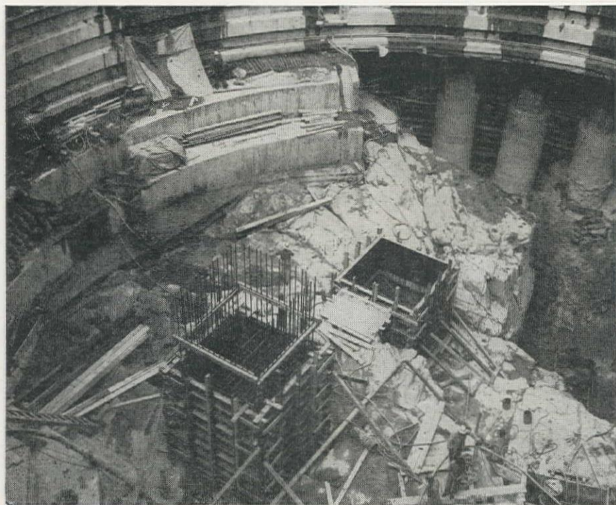
TWO OF THE FOUR central piers upon which the floating steel caisson will be supported inside the drydock. The very rough bedrock is clearly shown, with one of the unexpected deep gullies at the right. Foundation completed along the left wall.
