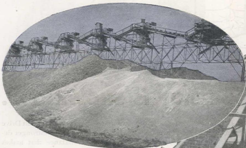
UNDER THIS STOCK PILE the conveyor belt is in a continual shower bath — must withstand constant dampness plus constant abrasion.
