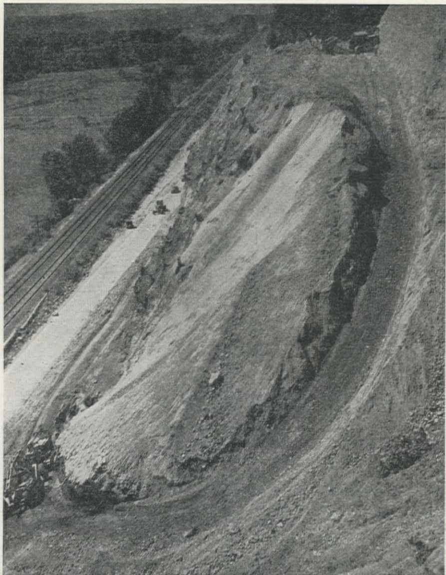
A HIGH CUT on the Leonard & Slate contract at Martins Bluff, showing heavy equipment removing rock for a fill in the background. A berm is usually carried on the outside of the cuts to prevent rock being accidentally precipitated on the road or railroad below. The conglomerate material in this cut forms a stable slope.
