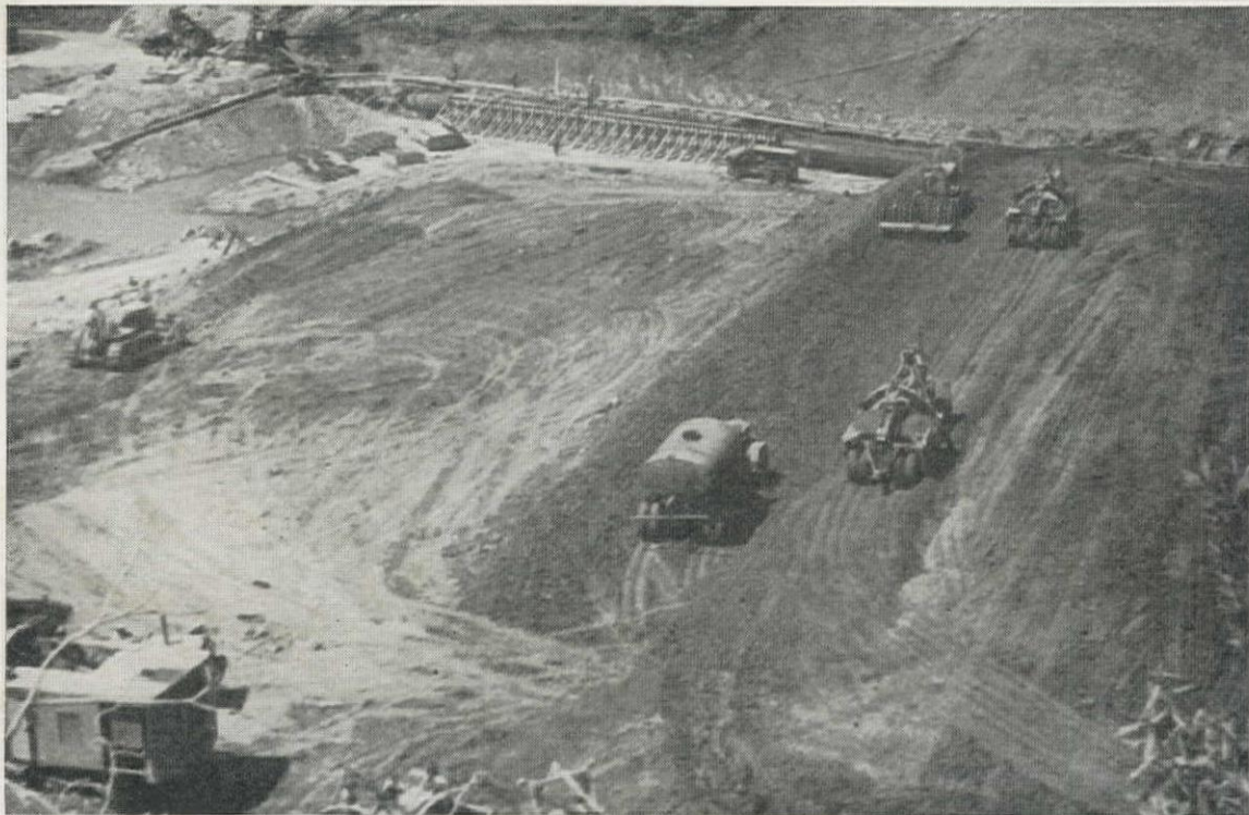
PLACING THE SELECTED impervious clay fill at Conn Creek Dam. A bulldozer is spreading heavy gravel fill on left section, flanking the clay core. In the background a 64-in. outlet conduit is being formed for concrete casing.
