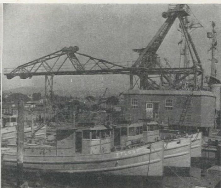
ERECTING THE DERRICK on the barge with the aid of a 40-ton stiff leg crane on the outfitting dock, left. Completed derrick prior to reeving cables and testing.
