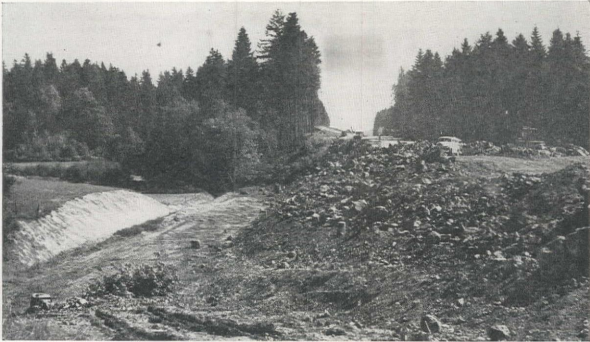
FIRST SAND BLANKET DRAIN in the Northwest is located under this 550 ft. fill on the Kalama-Woodland highway to facilitate rapid drainage of the boggy land underlying the fill. The sand drain empties into the ditch on the left which also diverts a small creek away from the highway. Engineers are closely watching the results of this experimental work.
