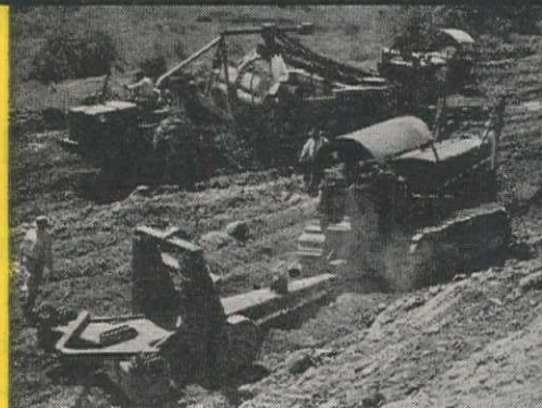
Tough rocky hardpan was loosened by LeTourneau heavy duty Rooter using two teeth.
