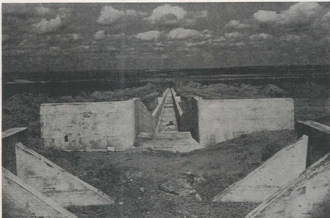
A LIBERTY LATERAL on the Tucumcari project. The long concrete construction is necessary to drop the water from the main canal, at the base of the mesa paralleling the S. Canadian River, without erosion to the fertile valley lands.
