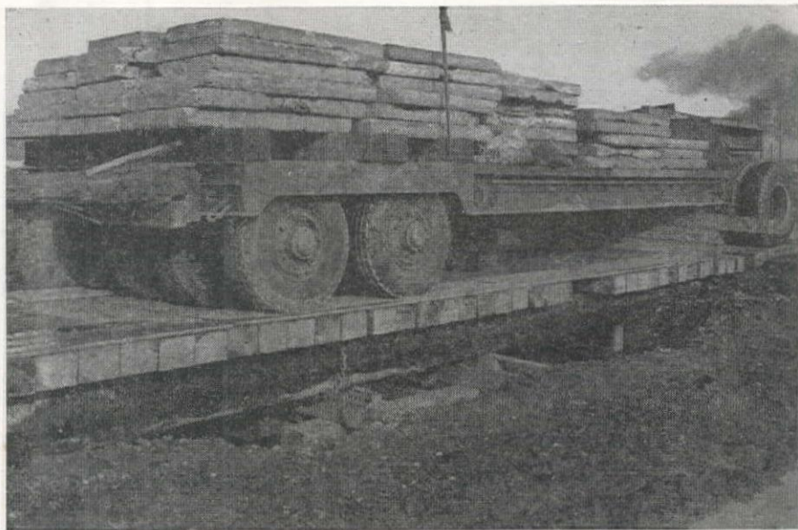
CALIFORNIA BEARING TESTS were conducted at the site of the warehouse prior to construction by the Army Engineer Soils Laboratory at the University of Washington. A truck heavily loaded with concrete slabs was used for measuring soil resistance. Surface soil was sandy, with deposits of silt and carbonaceous material.
