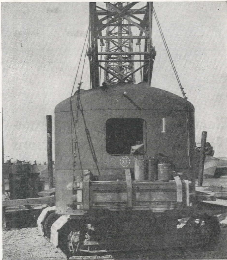
TO INCREASE the stability of the working cranes and keep them level, spare pile hammers and barrels of concrete were lashed to the back end of the crane cabs, as counterweights to help offset the weight of the heavily braced extra-length boom.
