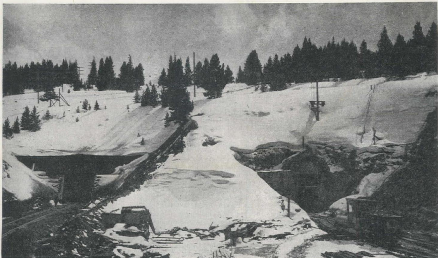
WEST PORTAL of the D. & R. G. W. tunnels at Tennessee Pass, the new one on the right. The old, originally driven in 1890 for narrow gauge trains, will be re-lined and maintained as standby structure.
