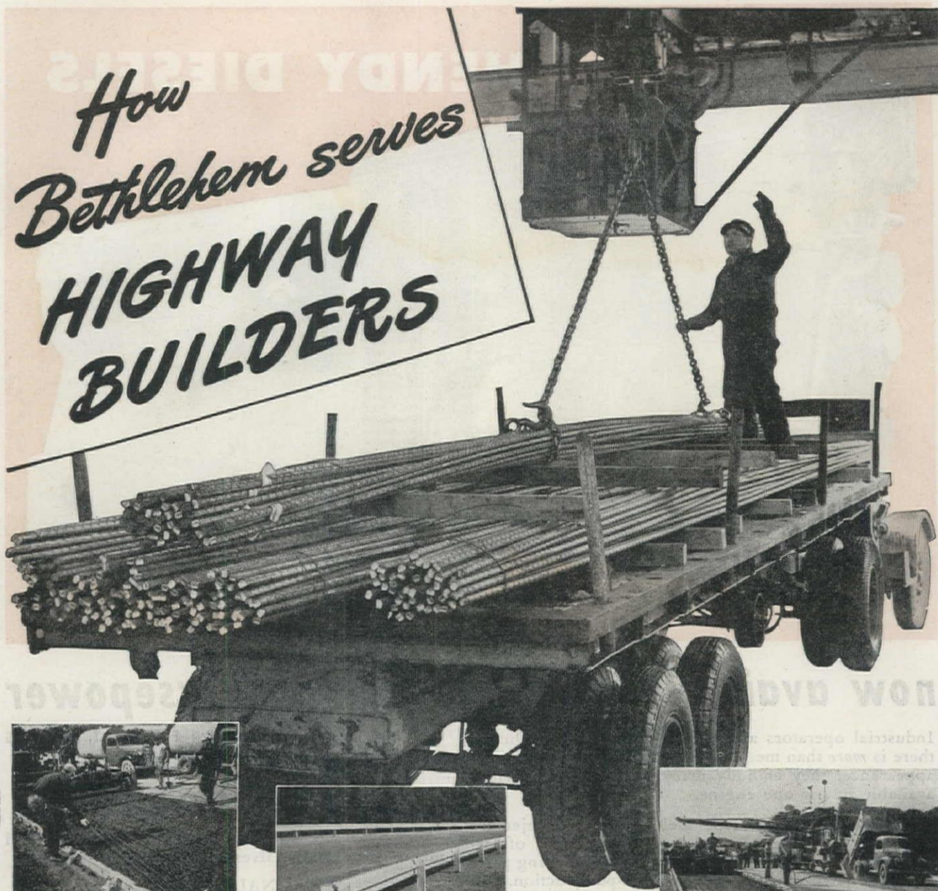
REINFORCING STEEL —Bethlehem Bar Mats, made of deformed bars clipped together, are easy and convenient to install, and lie flat.
