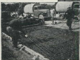
REINFORCING STEEL —Bethlehem Bar Mats, made of deformed bars clipped together, are easy and convenient to install, and lie flat.
