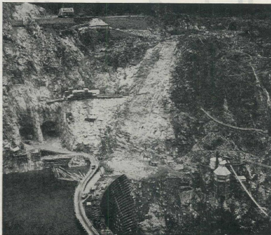
AGGREGATE HANDLING at Ross Dam, above. Left to right, lower face of Ross Dam, batching plant and cement silo, belt conveyor, screened aggregate bins, and below them cement pumping line crossing river, shops and equipment barge in lower right. Trestle being constructed over stockpile area, and aggregate barge landing in background. Below, left abutment wall sealed ready for grouting, and portals of power tunnels driven above the first step of dam so that work can progress without lowering water level.
