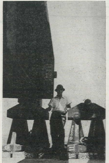
WALTER E. ROBEY , resident engineer for the railway on the Topock bridge, between the rockers used as support for the free ends of Spans 3 and 4 on Pier No. 3. Photo taken before erection of Span 3 by American Bridge Company.
