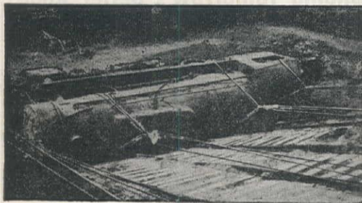
3 Two slings leading from the HYSTER Winches, and double-blocked to hand winches as a safety precaution, were then placed around the locomotive and raising got underway.
