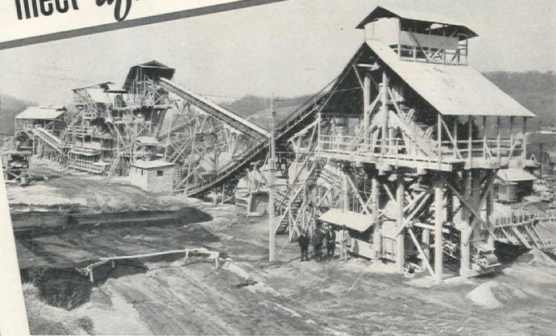
Complete modern TelSmith plant ... producing both coarse and fine aggregates in several sizes.
