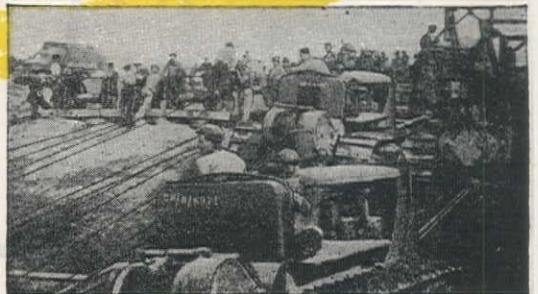
2 A nearby British school of mechanical engineers loaned two "Caterpillar" tractors equipped with HYSTER Towing Winches. A skid mat of rails anchored to ties was built.
