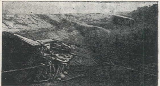
4 The locomotive was finally raised to level ground, rotated parallel to right-of-way, and rolled over on its wheels. Job was completed during bitter cold and stormy weather.
