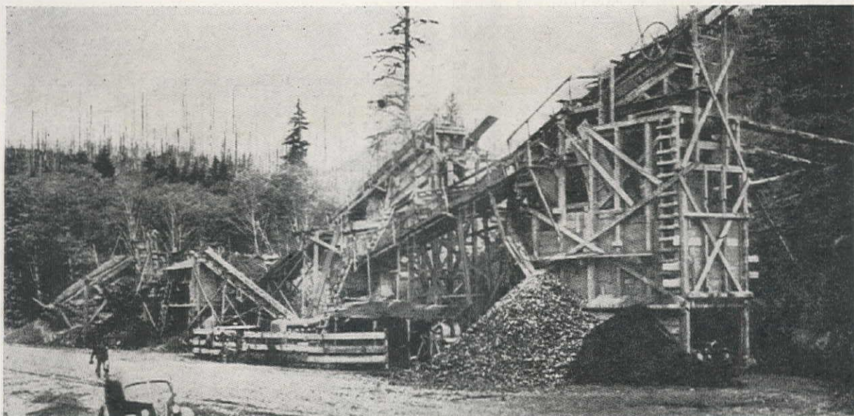
View of temporary West Coast plant using three 4' x 10' Triple Deck Screens to produce 3130 tons per hour of rock.
