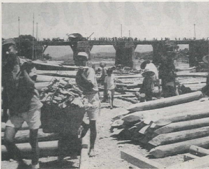
A BRIDGE 1,800 YEARS OLD is being repaired in southwest China, under direction of the U. S. Army Corps of Engineers. The bridge crosses the Yuan Hwo river, and was built during the Tong dynasty. Massive stone piers were built during the
