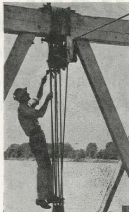
REGULAR CLIP inspection should be made and clips tightened to prevent damage to rope and assure safe rigging.
