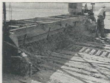
This is an example of deep cutting into tough material—gravel as large as 14" in diameter is handled with ease.
