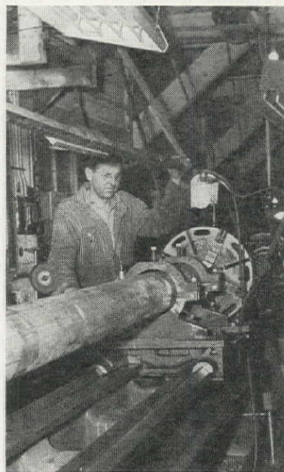
HEAVY ALUMINUM tubing 16 ft. long are centered in the lathe fixture, and inside and outside surfaces machined by a rotating tool held secure in chuck.
