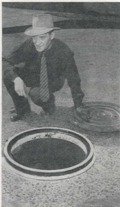
L. F. SAYLES , inventor of the manhole adapter, checks placement of one of the devices before blacktop resurfacing is placed on a Portland street.
