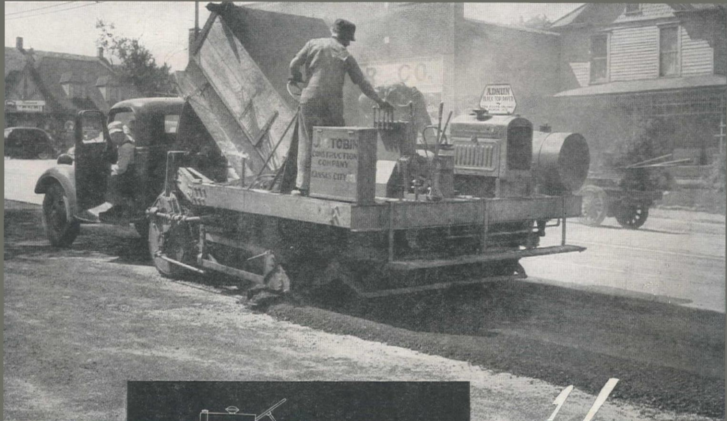
The first course showing front wheel dropped into deep depression.
