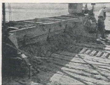
This is an example of deep cutting into tough material—gravel as large as 14" in diameter is handled with ease.
